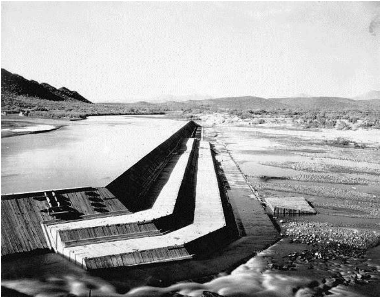
Figure 38: Arizona Canal wood-crib diversion dam, 1902. Source: U.S. Library of Congress, Washington, D.C.
