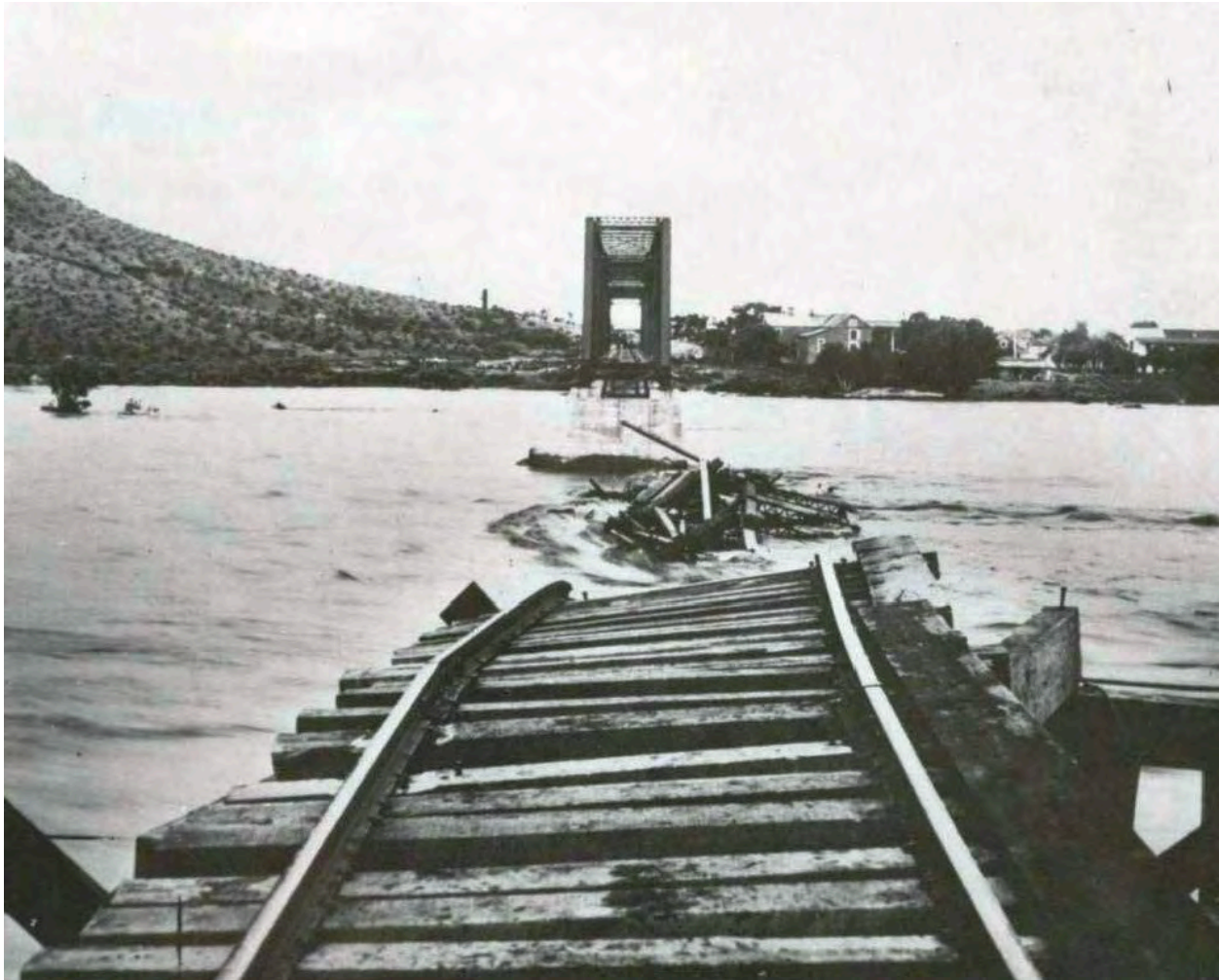
Figure 70: Salt River railroad bridge destroyed by April 1905 flood. Source: Arizona Memory Project (online photographs from multiple archival sources).
