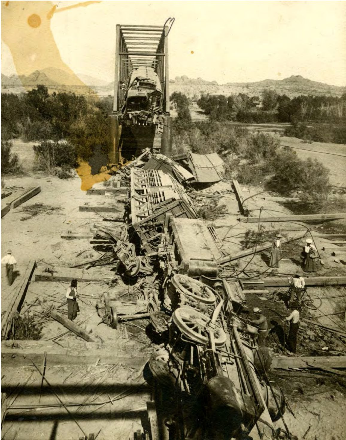
Figure 35: Train wreck on Salt River railroad bridge, 1902. View from Tempe end of bridge. Also observe the phreatophyte growth in the river bed – a characteristic of rivers that are frequently dry. (Stain is on the original source photograph.) Source: Special Collections, Arizona State University, Tempe, Arizona.
