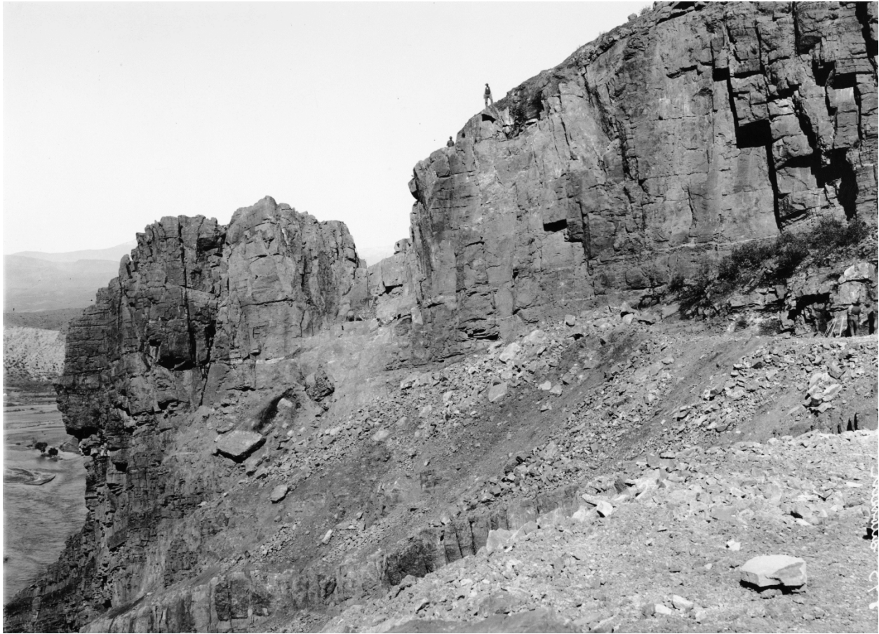
Figure 45: Site of cut for Roosevelt Road (notch in rocks) before excavation, ca. 1906. Cut location is immediately above Roosevelt Dam site. Note man on right side of notch. Source: Records of the U.S. Bureau of Reclamation, U.S. National Archives branch, Denver, Colorado.
