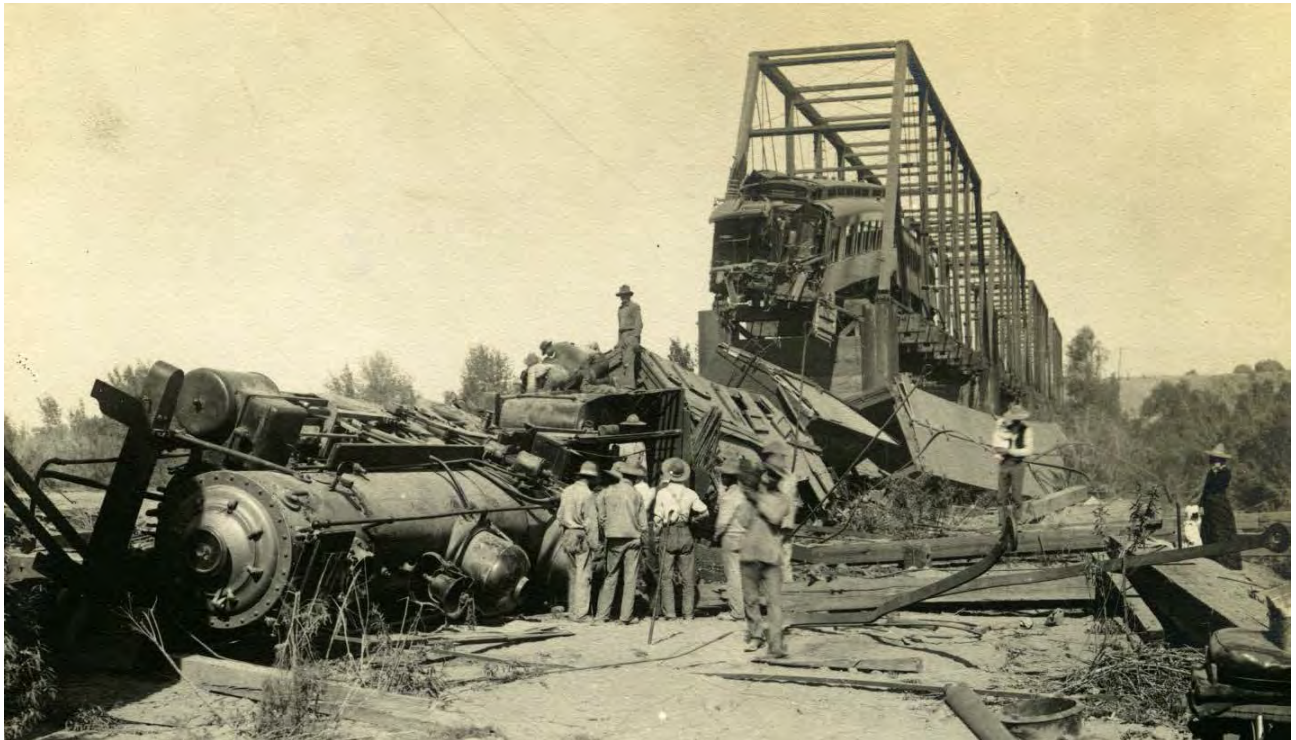
Figure 34: Train wreck on Salt River railroad bridge, 1902. Note that the engine and men are standing in the Salt River's bed. Source: Special Collections, Arizona State University, Tempe, Arizona.
