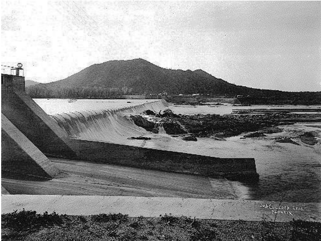
Figure 51: Granite Reef Dam after completion, ca. 1909. Source: Phoenix Public Library, Phoenix, Arizona.
