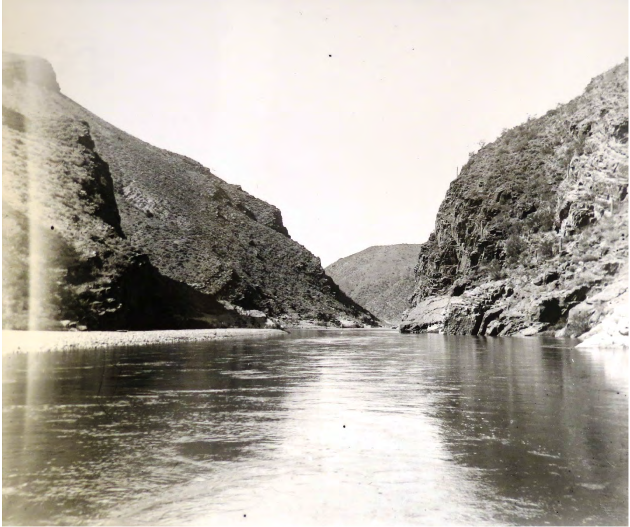
Figure 41: Salt River Canyon, ca. 1900. Note the precipitous cliffs that made constructing the Reclamation Service road from Phoenix to Roosevelt very difficult. Source: Special Collections, Arizona State University, Tempe, Arizona.
