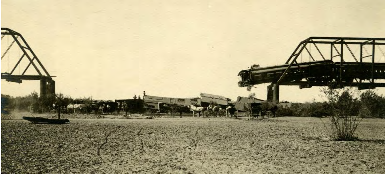
Figure 33: Train wreck on Salt River railroad bridge, 1902. Also observe the height of the concrete towers supporting the bridge and compare to how little of those towers appear during floods. Source: Special Collections, Arizona State University, Tempe, Arizona.
