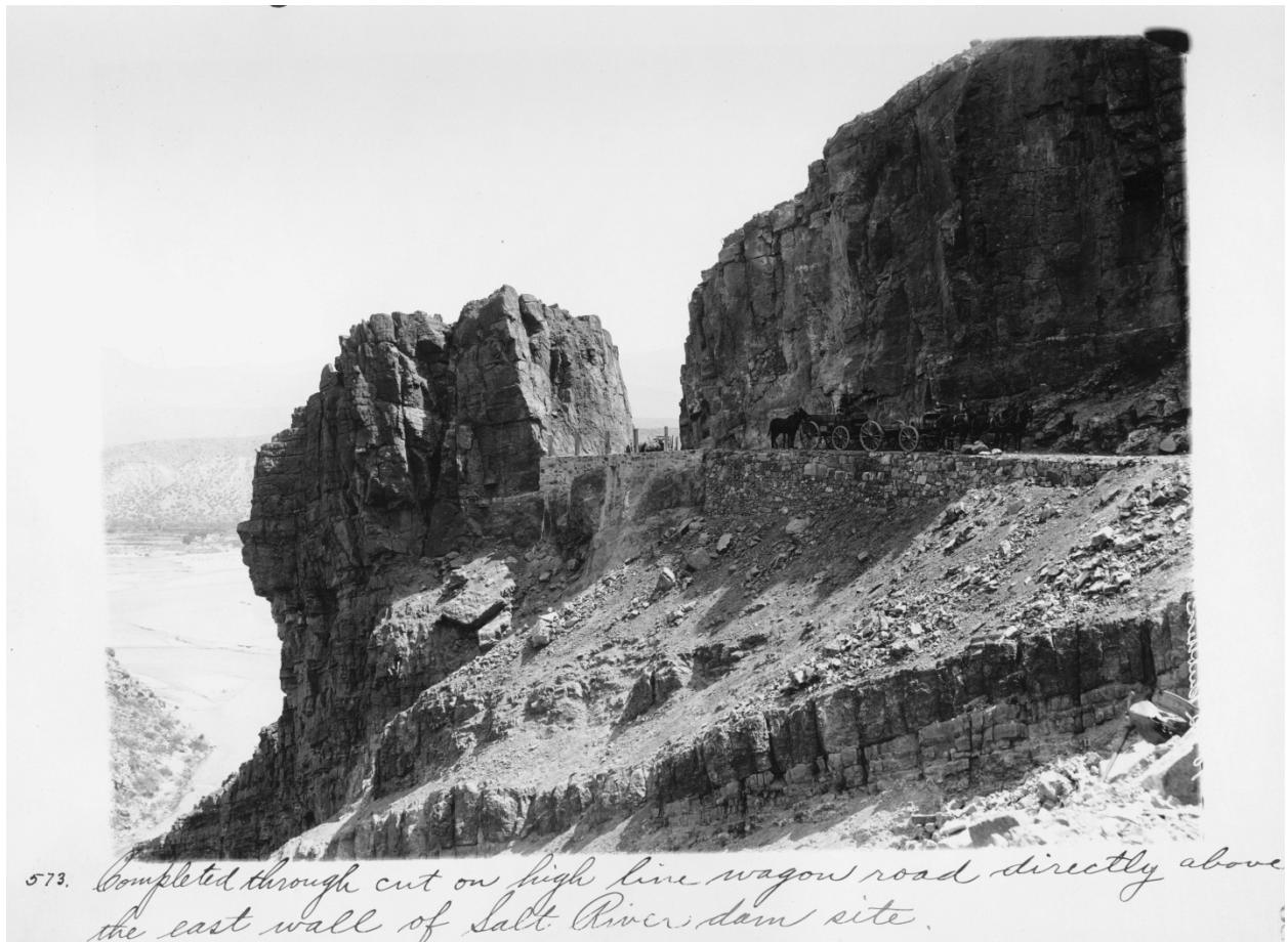
Figure 47: Completed through cut on high line wagon road directly above the east wall of the Salt River dam site, 1907 (viewed from opposite side of cut from previous illustration). Source: Records of the U.S. Bureau of Reclamation, U.S. National Archives branch, Denver, Colorado.
