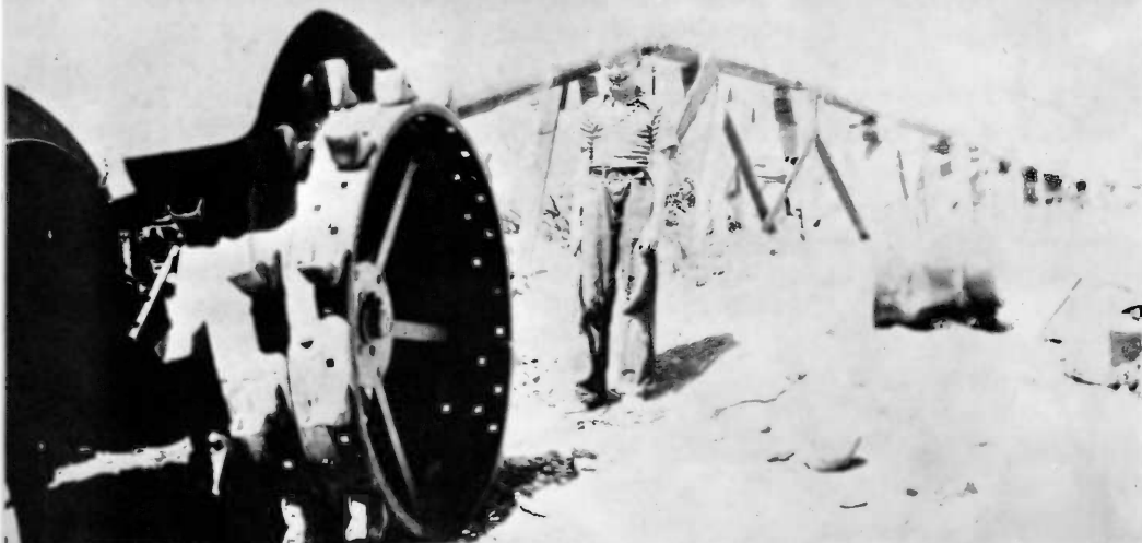
Discharge Pipe delivering water to land from O.K. Ditch from 6" Centrifugal pump operated by old tractor. June 7, 1940.
