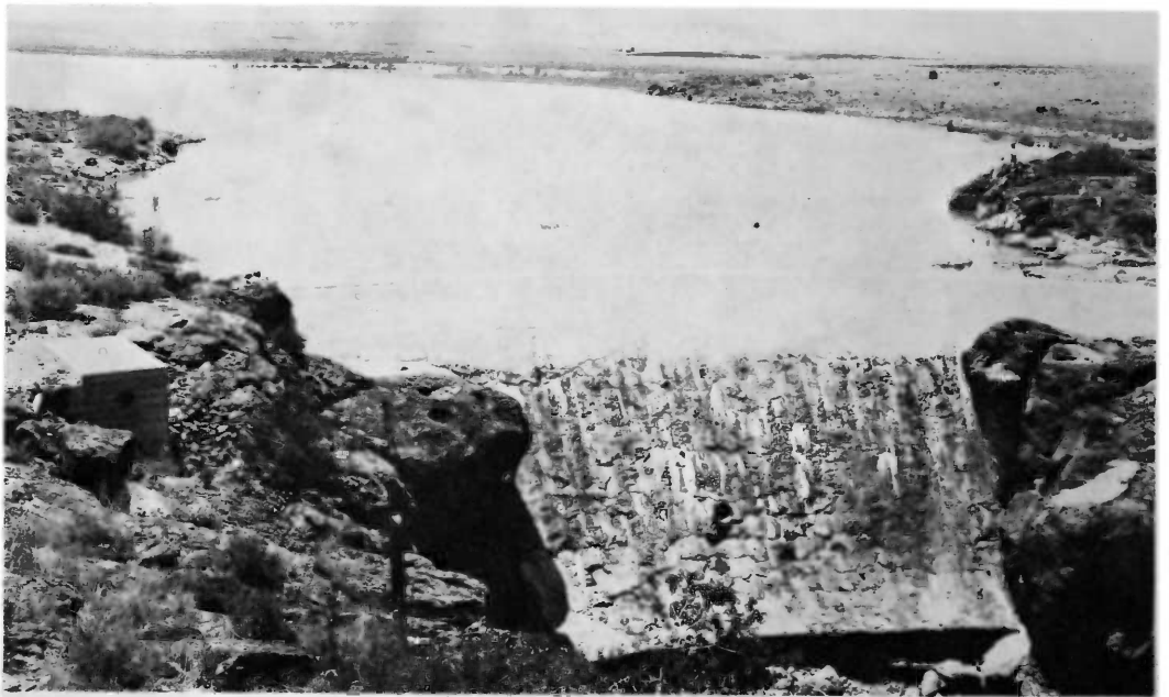
Prescott Gun Club Dam - Head of Verde River Looking West from Highway, July 25, 1940.
