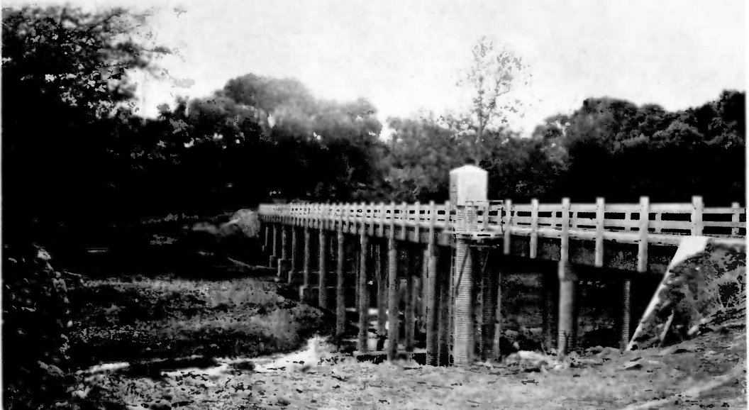
New U.S.G.S. Gaging Station at Highway Bridge, Oak Creek, July 26, 1940.
