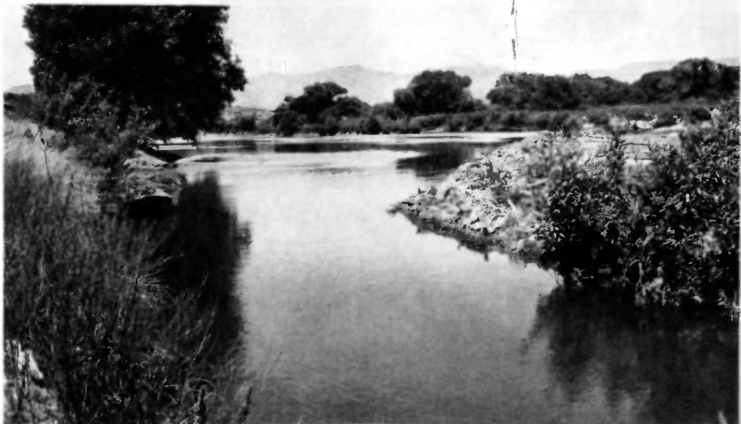
Diversion Dam and Intake - Wood Ditch - June 6, 1940.
