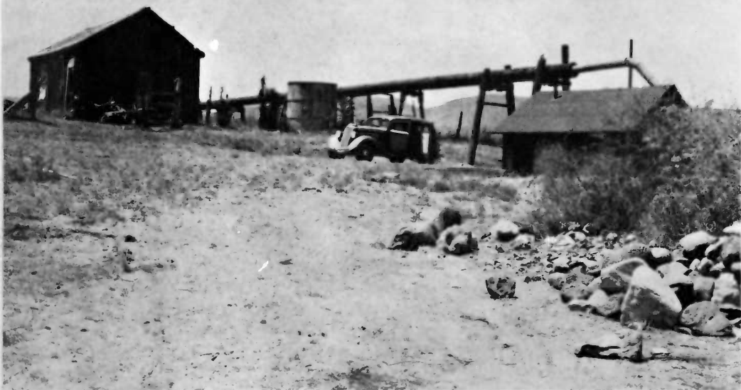
Pumping Plant in pit at extreme right with discharge to Lebsch Ditch, formerly part of C.V. Ditch (Head of Wood Ditch nearby) June 6, 1940.
