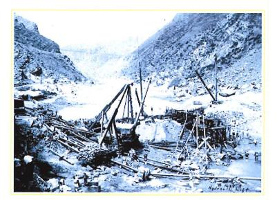
Here, on July 16, 1906, workers are rebuilding the downstream cofferdam, using a "hydraulic lift" much like a canal lock, to lift excavated material. Digging reached bedrock 30 feet below the river surface where foundation stones were laid in cement mortar on the thoroughly washed bedrock. In December, the Salt River flooded, overtopping the cofferdams and washing away everything seen here. But the cemented stones didn't budge.
