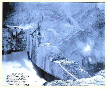
By November 1, 1909 the dam was almost 200 feet high on the south side. A week later the sluicing gates would reopen, diverting the river from flowing
