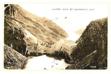
A view of the dam from downstream in late summer 1908 shows the south side rising above 70 feet and work restarted on the lower north side after the sluicing tunnel reopened. The powerhouse is enclosed and water can be seen
