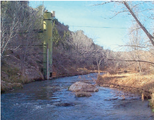
Figure 9.10 —U.S. Geological Survey Paulden Gauging Station upstream of the Verde River Ranch near Paulden, Arizona. (Photo by Daniel G. Neary.)
