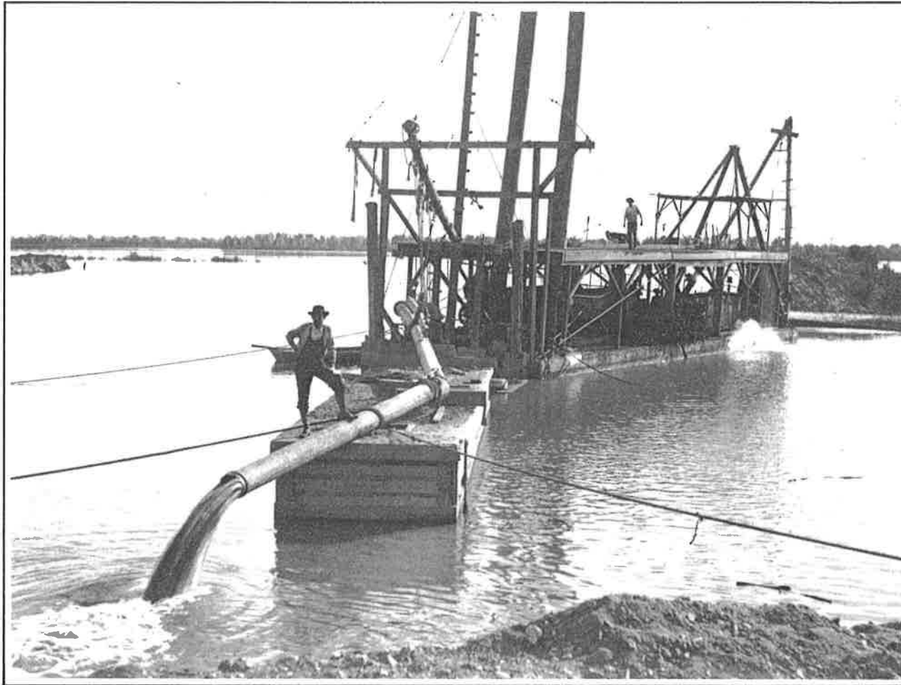
The failure of the Alpha to keep the canal intake free of silt led to construction of this suction dredge, the Beta , but even together they were unable to remove the silt as fast as it settled.
