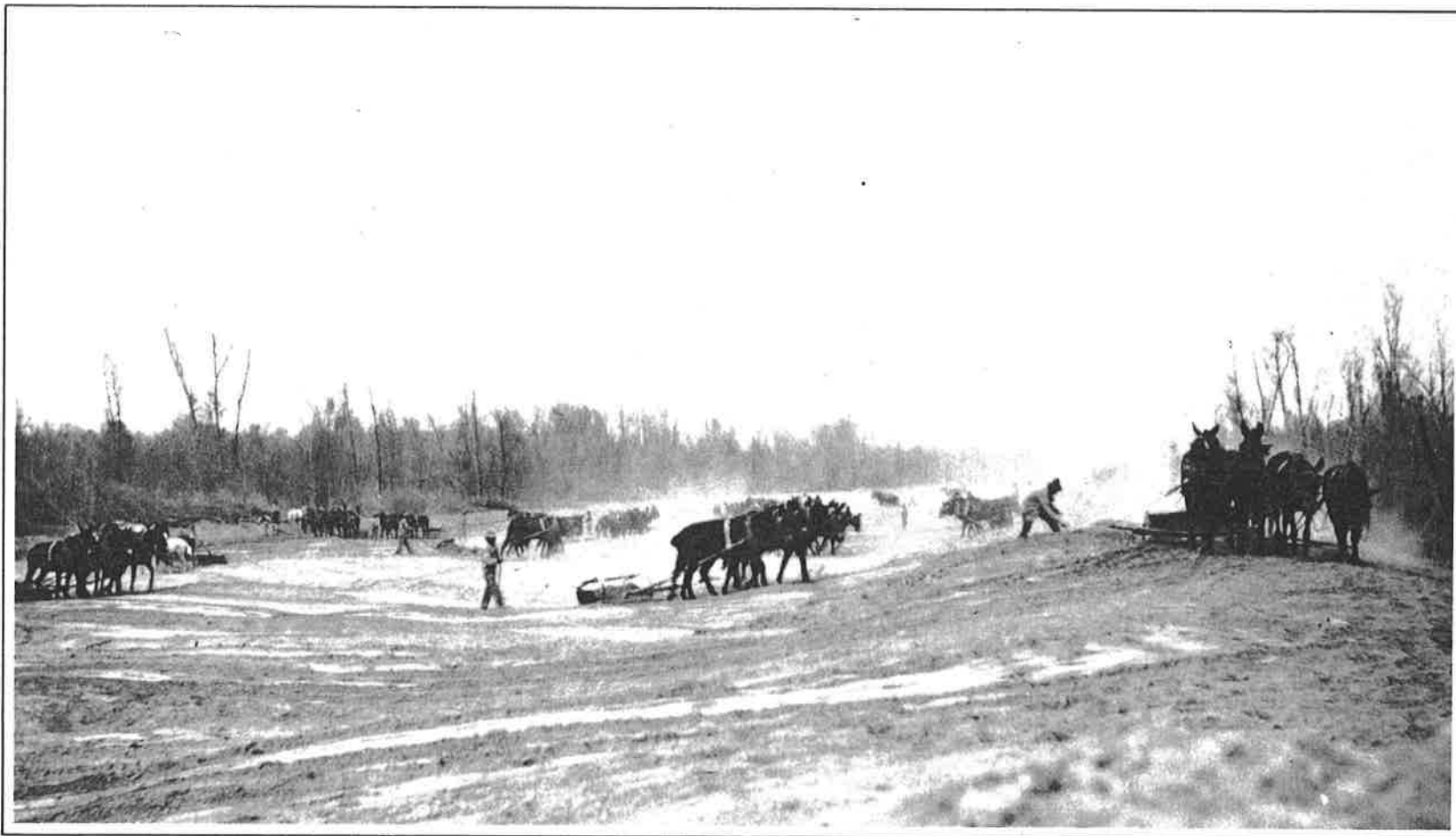
Fresno scrapers aided the dredge in digging connecting canals and deepening the old Alamo overflow channel.
