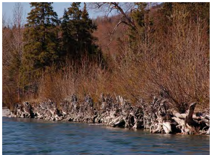
Figure 8.2 | These root wads were installed on the Kenai River in Alaska to prevent erosion. The result is a structure that looks overly symmetrical and obviously man-made, detracting from the natural scenery.
