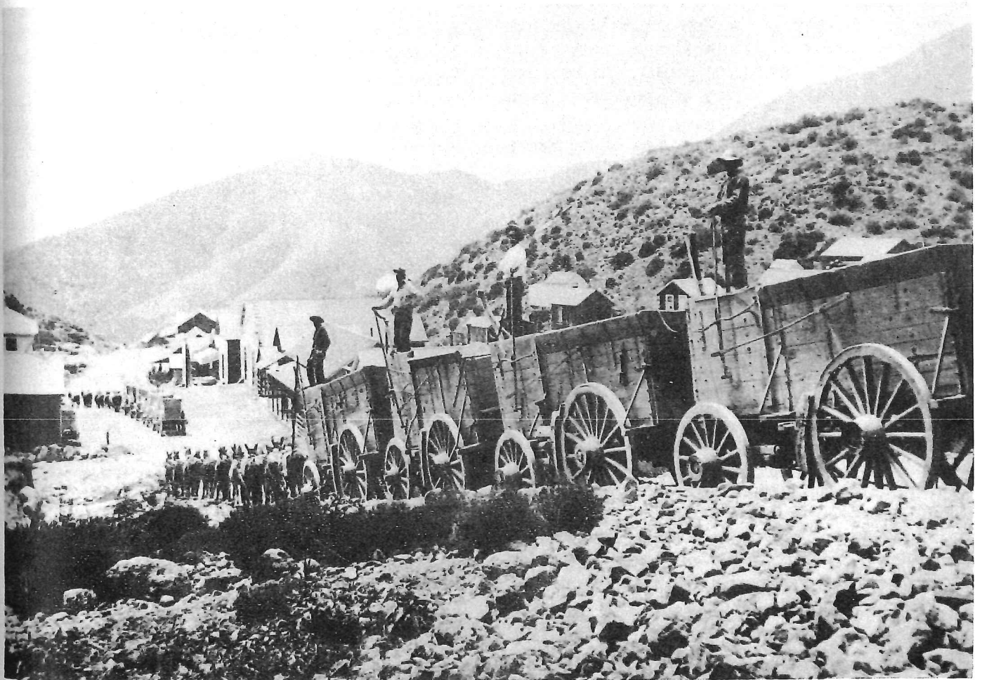
Loaded ore wagons. Note the brakeman on each wagon during the descent into town.
