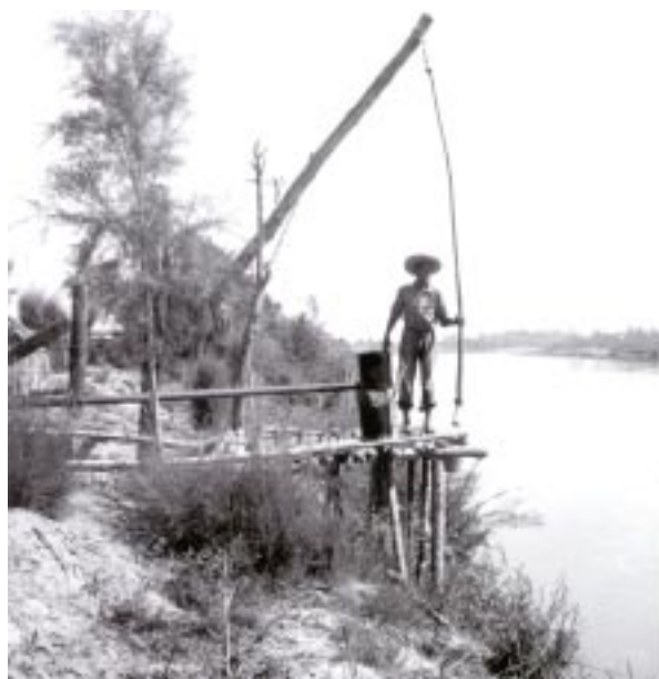
Fig. 18. Primitive water lift believed to have been located in the Colorado River delta (date unknown). Courtesy of the Bureau of Reclamation, Yuma, Arizona.
