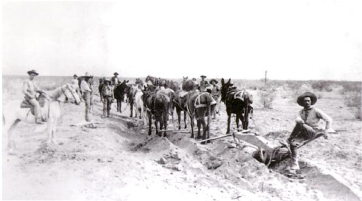
Fig. 19. Early settlers using horse-drawn plows to help dig the first irrigation canals. Courtesy of the Arizona Historical Society, Tucson.
