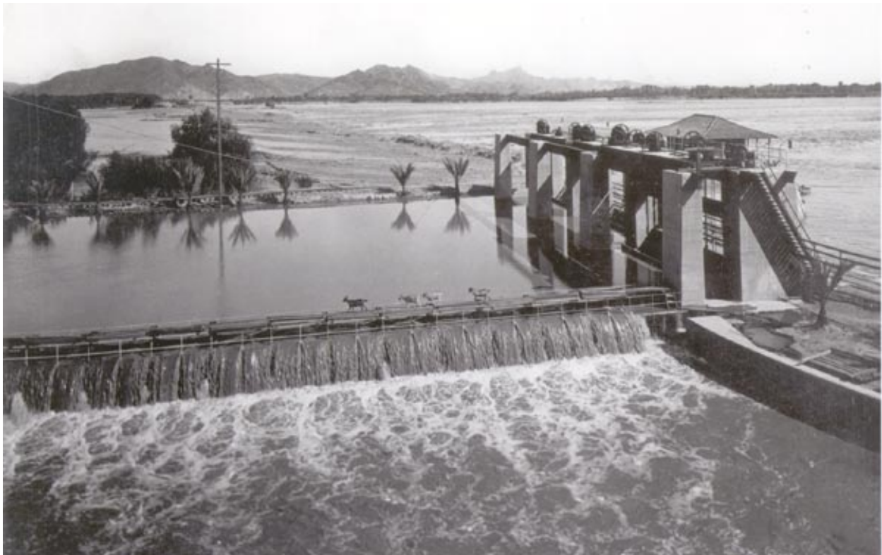
Fig. 63. The flood of 1922 breached the weir at Laguna Dam. Such floods were common until Boulder Dam was built in 1935, P45-300-4414A. Courtesy of the Bureau of Reclamation, Boulder City, Nevada.
