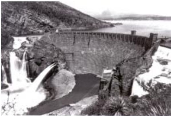
Fig. 26. Theodore Roosevelt Dam, P0025-330-011951. Courtesy of the Bureau of Reclamation, Boulder City, Nevada.
