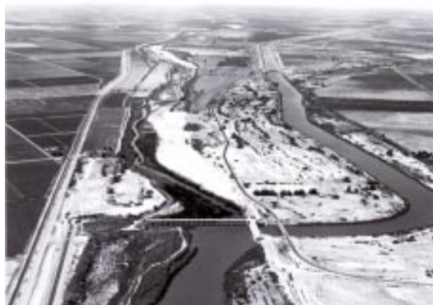
Fig. 31. Morales Dam diverts the remaining waters of the Colorado River to Mexicali Valley (1973). Courtesy of the Bureau of Reclamation, Boulder City, Nevada.
