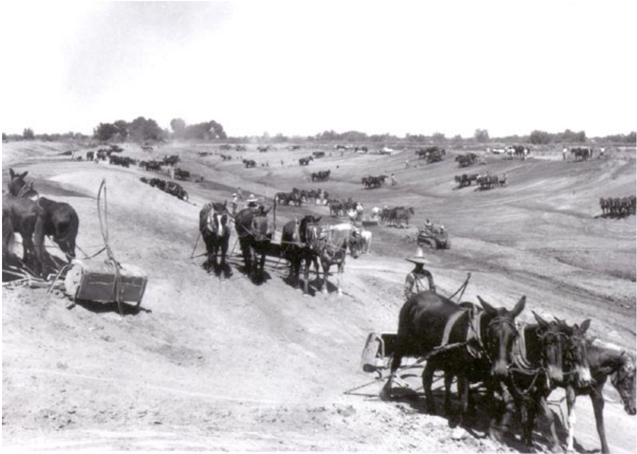
Fig. 22. Horse and mule-drawn scrapers help dig the All-American Canal in 1935, P212-303-269A. Courtesy of the Bureau of Reclamation, Boulder City, Nevada.
