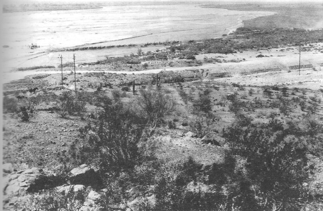
Figure 5. Photograph of the Gila River taken near Olberg in March 1915. View is looking downstream with Sacaton visible to the left in the distance. At least 50 Akimel O'odham men assisted by 21 two-horse powered wagons repair a brush intake weir on the streambed of the Gila River. They are trying to divert water into the historic Santan Canal. The Gila River channel is about one kilometer wide in this view. (Homer Shantz Collection, Herbarium, College of Agriculture, University of Arizona, Tucson).
