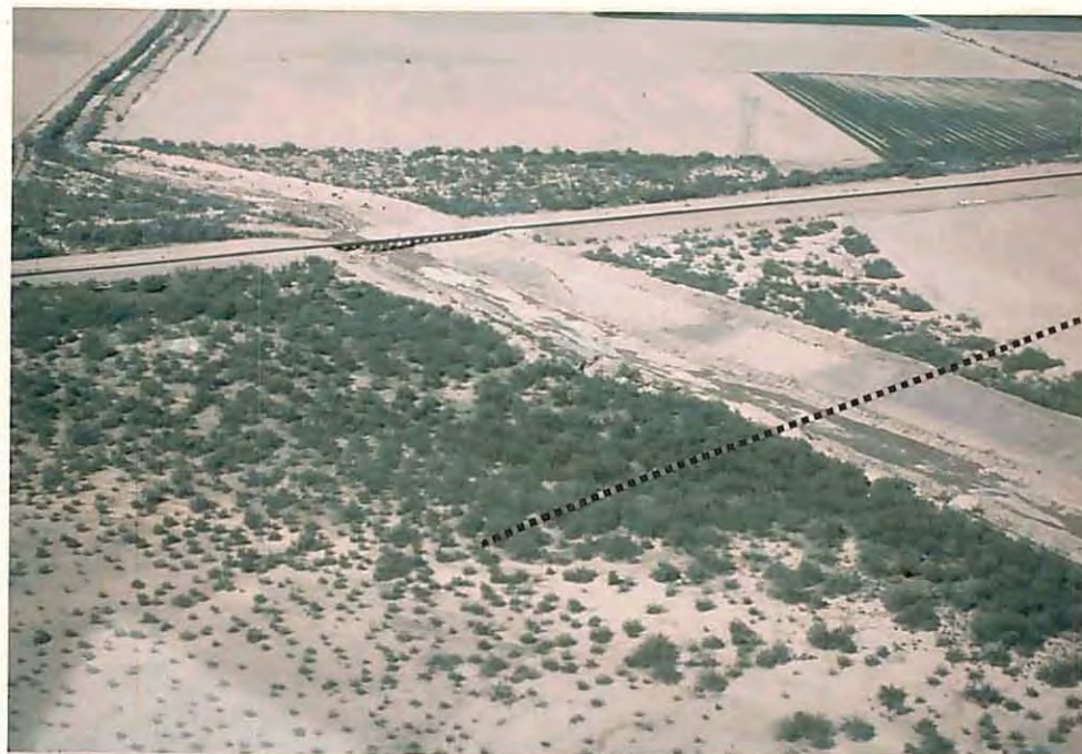
B. Looking upstream and across channel at cross section and railroad bridge from above right bank.
