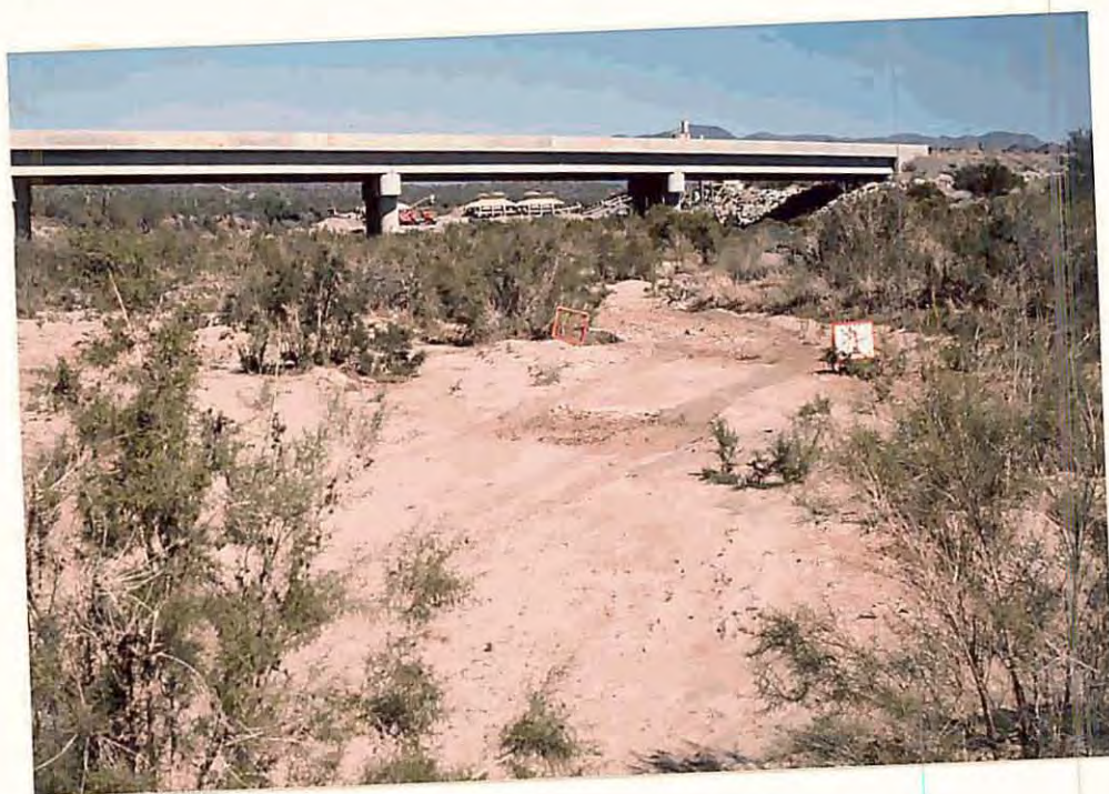
D. Looking upstream at low-flow channel.
