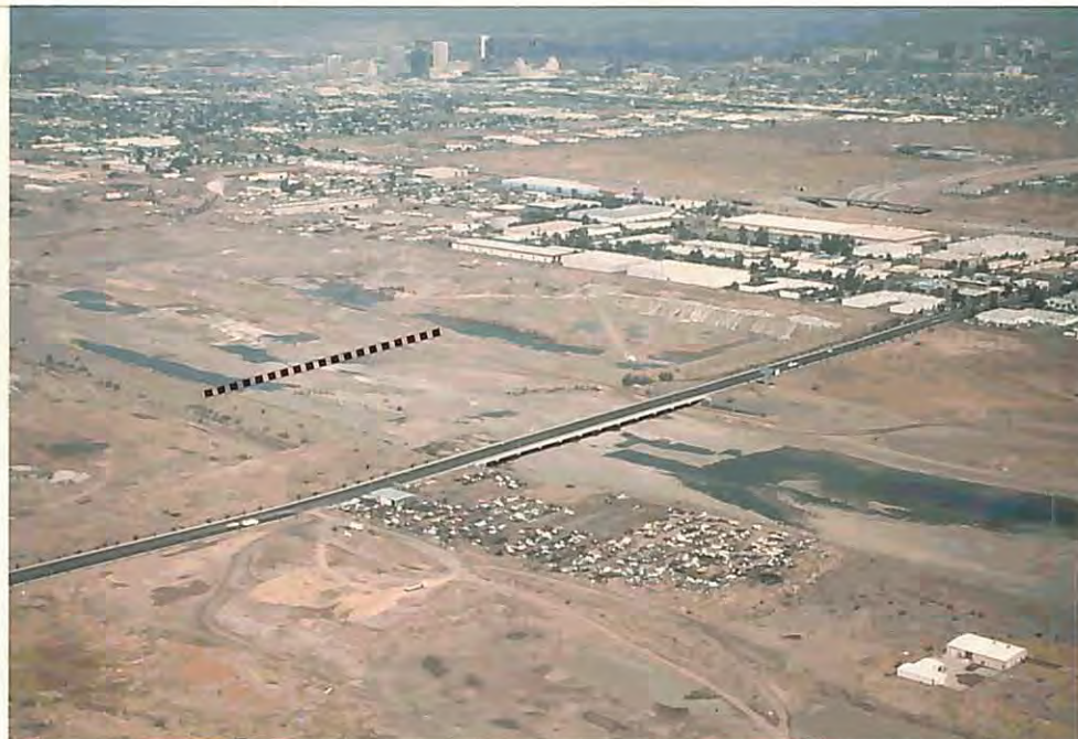
A. Looking downstream and across at cross section from above left side.
