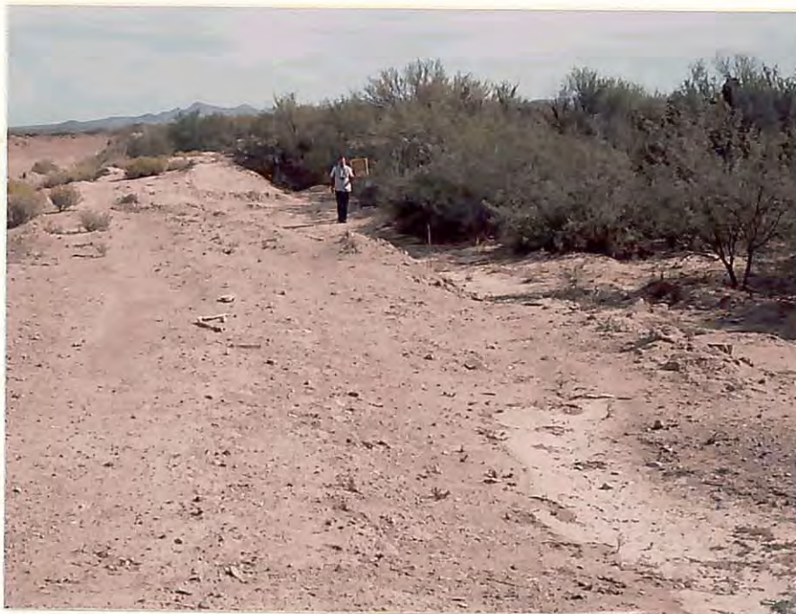
E. Looking downstream along channel side of right bank overflow.
