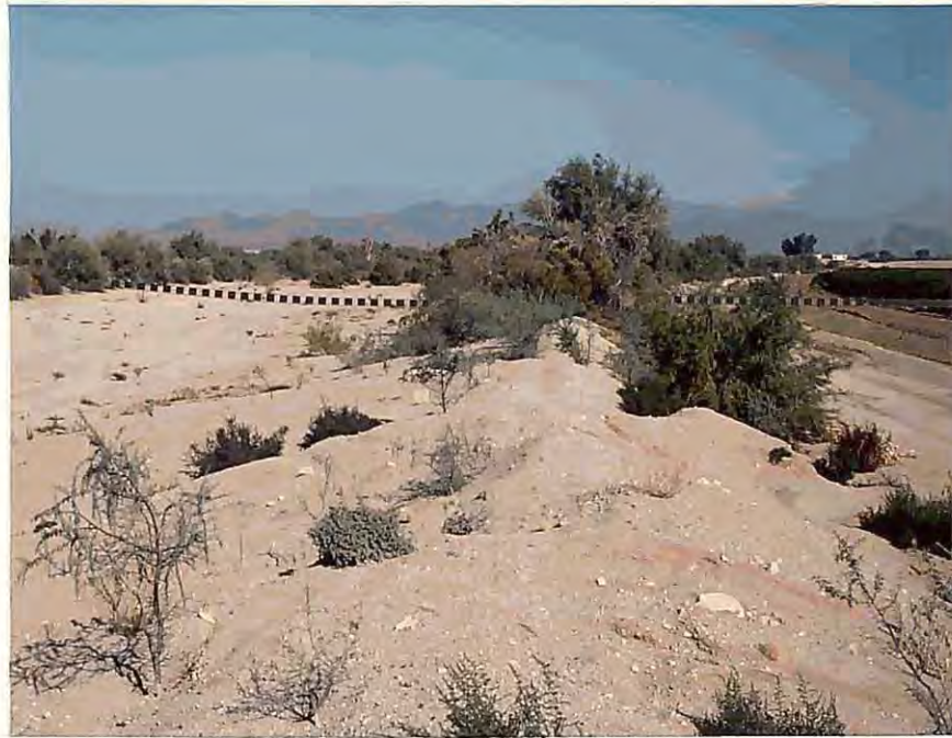
A. Looking downstream at cross section from right bank of main channel.
