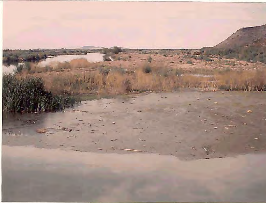
C. Looking upstream from crest of dam at left side of channel.
