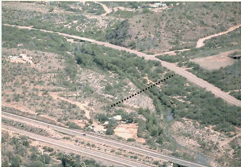
A. Looking upstream at cross section from above Interstate Highway 17.
