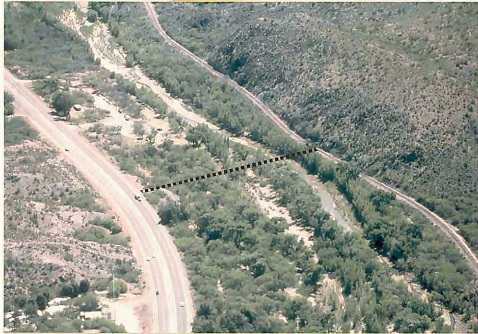
A. Looking downstream at and across from above left bank.
