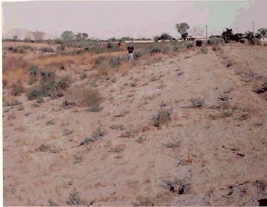
C. Looking downstream along left bank.
