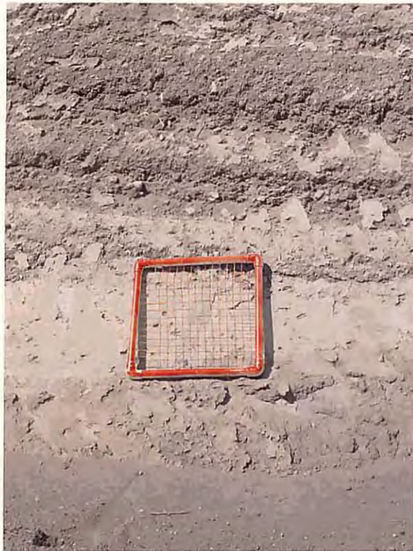
E. Soil cement on right bank.
