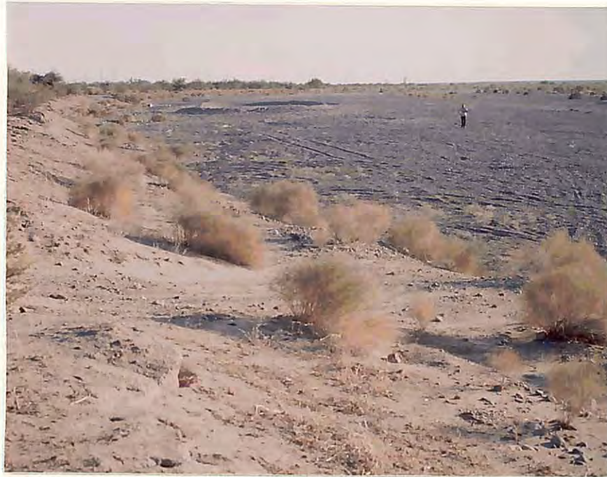
C. Looking downstream along left bank.
