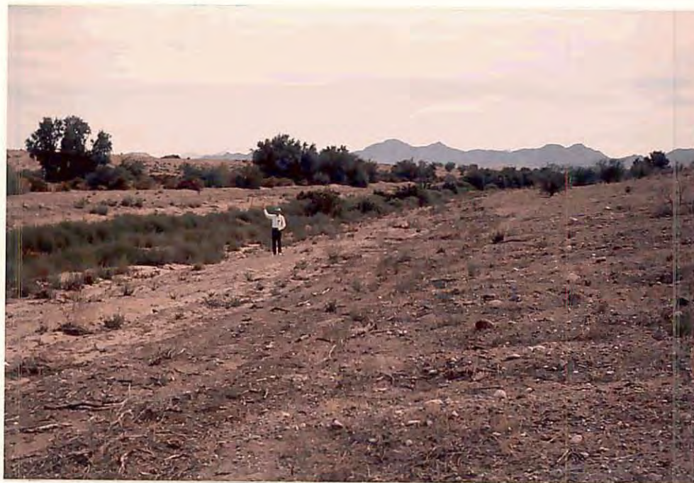
D. Looking downstream along right bank.
