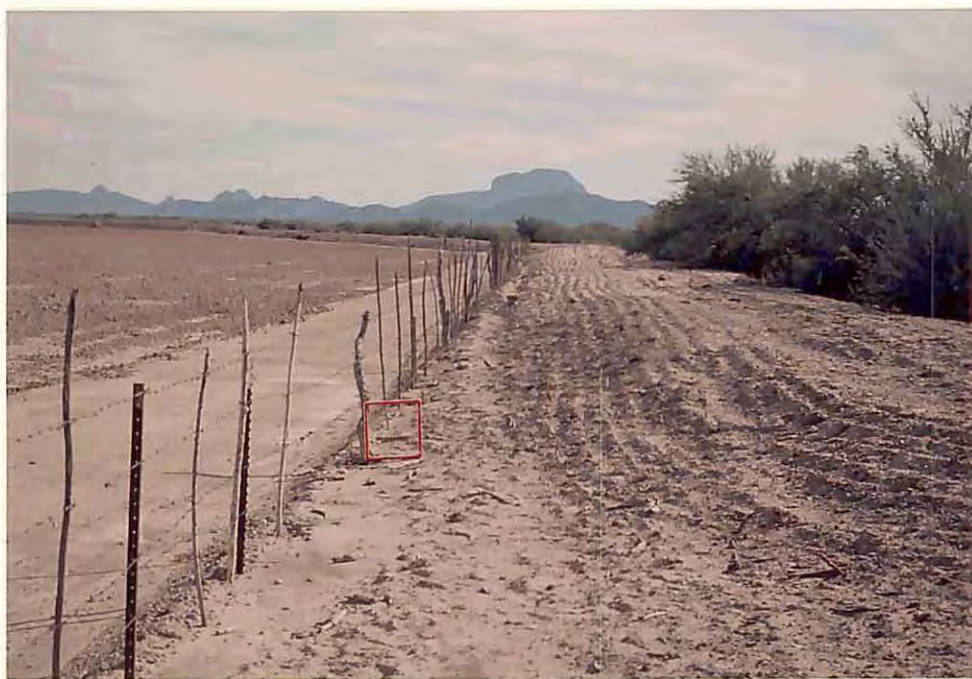
H. Looking downstream at small dike that separates cultivated field from native vegetation on left overflow at cross-section station, 8,570 ft.
