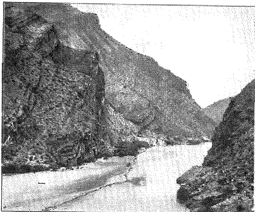
B. SOUTH ABUTMENT OF SALT RIVER DAM, LOOKING DOWNSTREAM.
