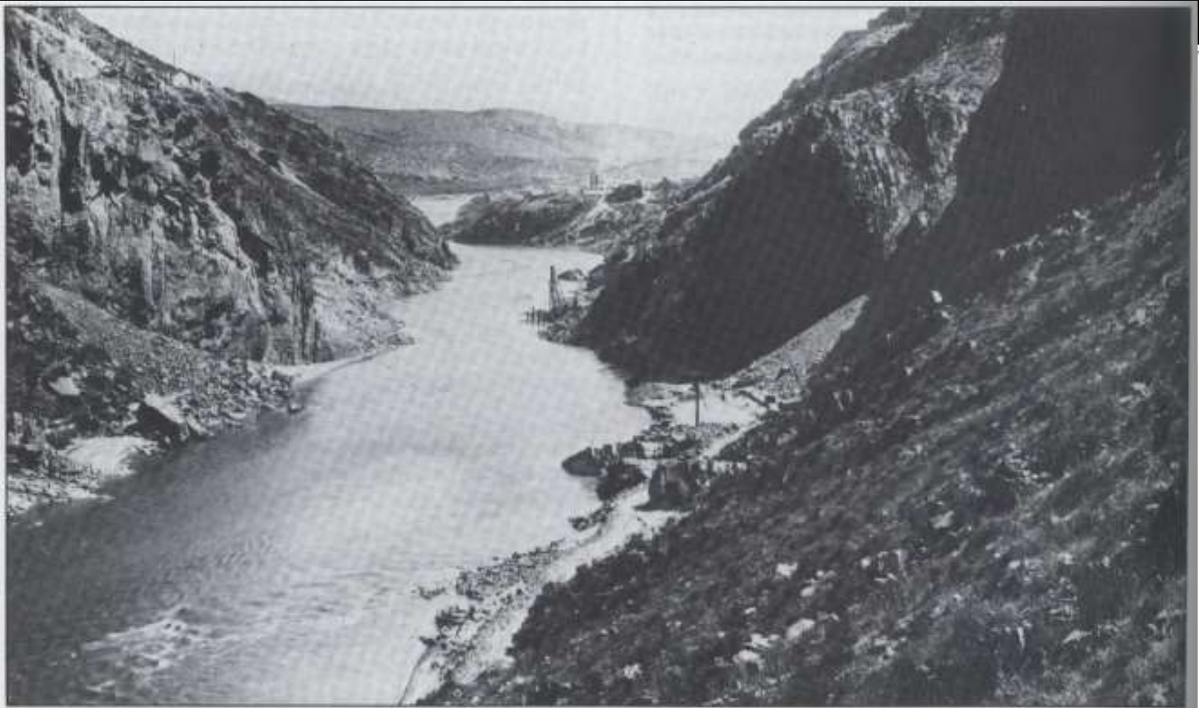
Looking upstream at site of Roosevelt Dam on the Salt River, April 16, 1906.
