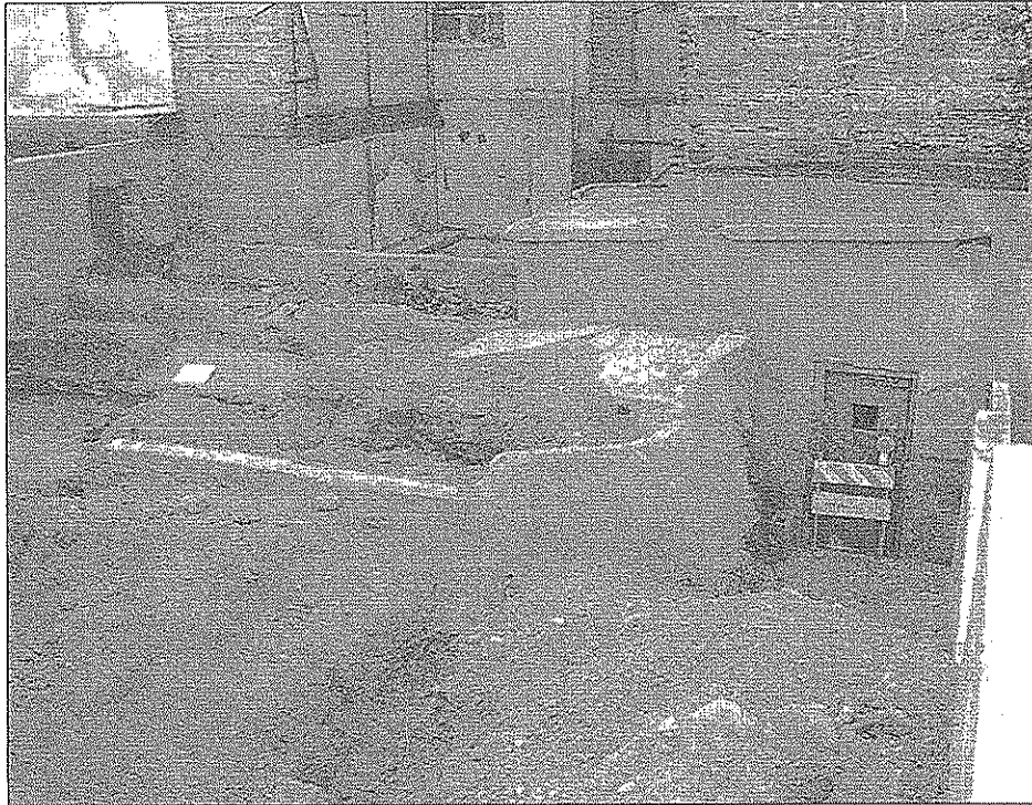
Figure 24.49. Photograph of concrete retaining wall Feature 8, Hayden Ditch site (AZ U:9:189[ASM]), facing southwest towards concrete-lined head race Feature 6 and penstock Feature 39 (AZ U:9:278[ASM]).
