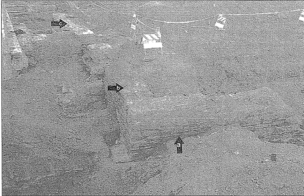
Figure 24.9. Photograph of tail race Feature 7 ([a] western retaining wall extension), Hayden Ditch site (AZ U:9:189[ASM]), and a later east-west wall addition ([b] Feature 53, Wall Segment 3; AZ U:9:278[ASM]) that was part of the foundation of the original adobe mill, facing west.
