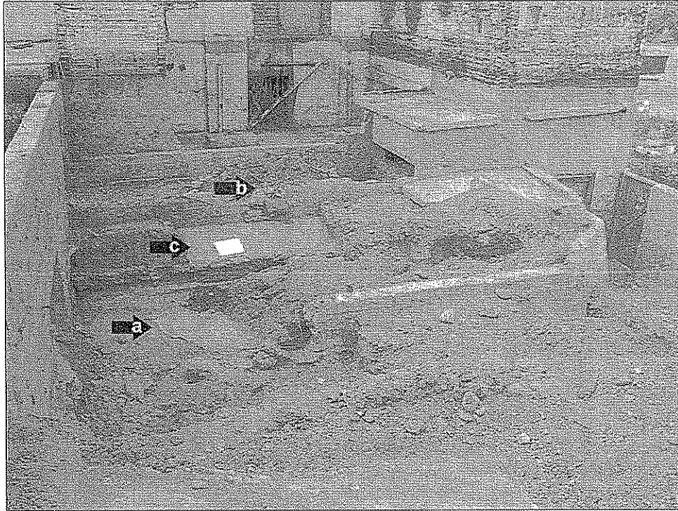
Figure 24.38. Photograph of a sloped concrete surface (Subfeature 5.01 [a]) below the concrete-lined head race (Feature 6 [b]) and its attached sloped concrete slab (Subfeature 6.02 [c]) in the background Hayden Ditch site (AZ U:9:189[ASM]), facing northwest.
