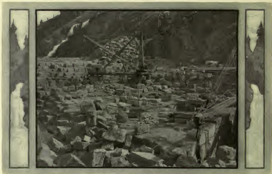
Building the Tonto Dam
