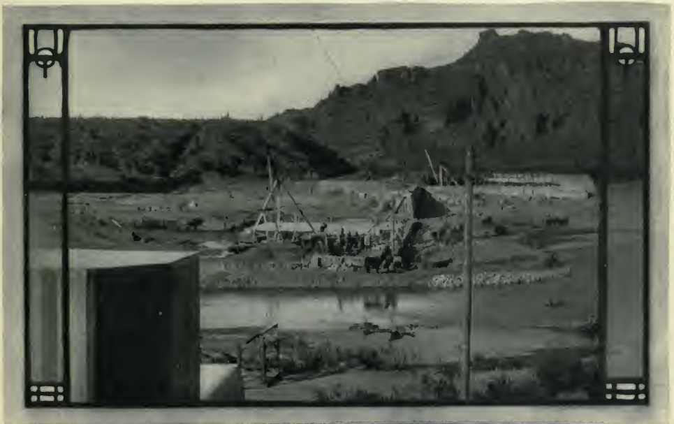
Constructing Granite Reef Division Dam
