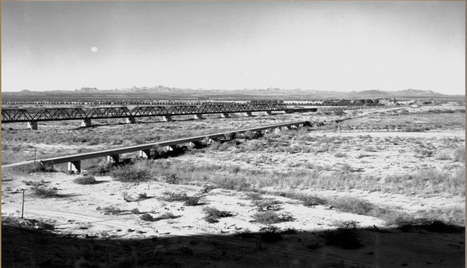
Dry Gila River near Antelope Hill, January 16, 1940. Source: Records of the U.S. Bureau of Reclamation, U.S. National Archives branch, Denver, Colorado.
