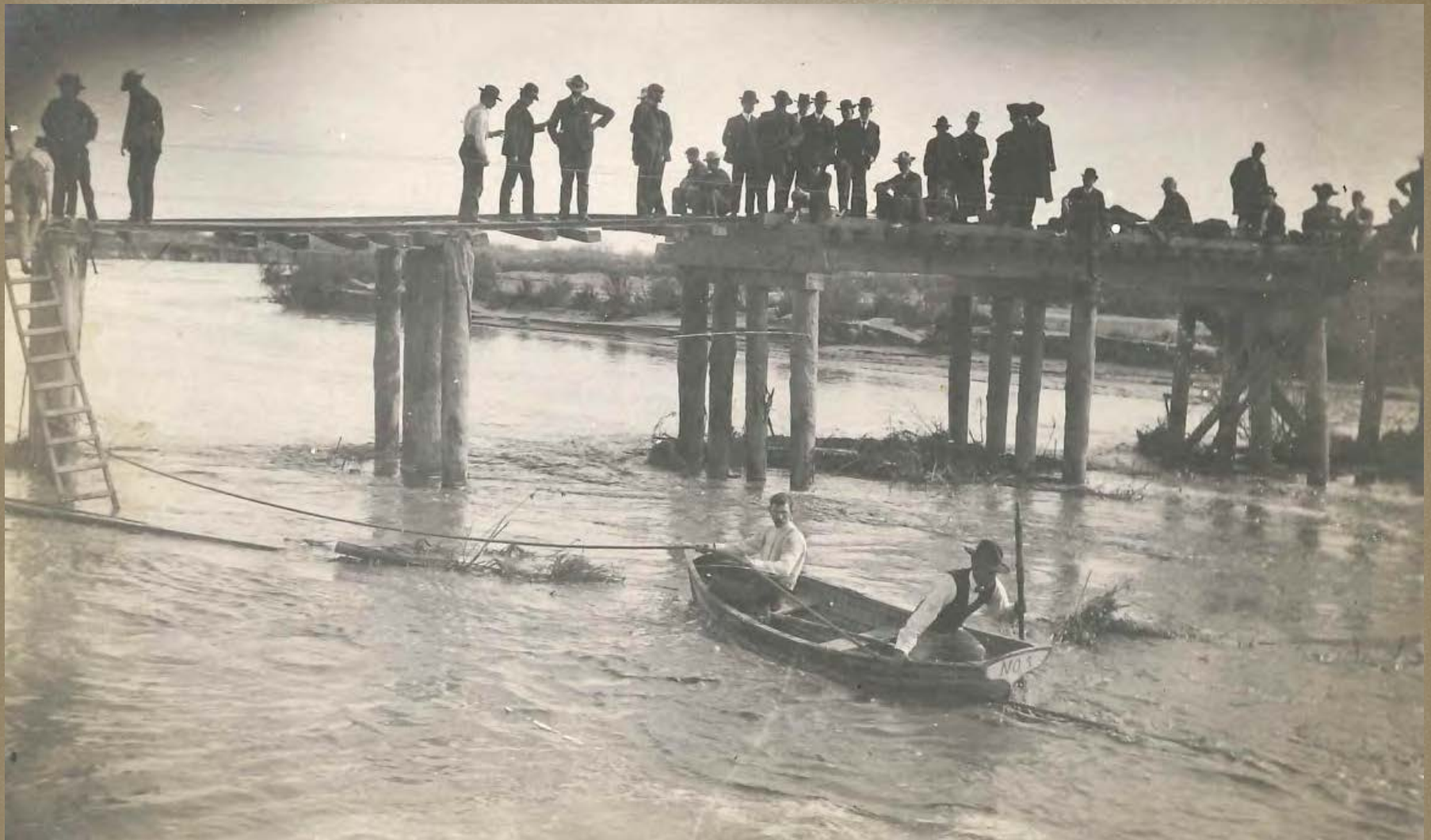
Workers use a small boat to examine the railroad bridge damaged by the 1905 Gila River flood. Source: Arizona Historical Society, Tucson, Arizona.
