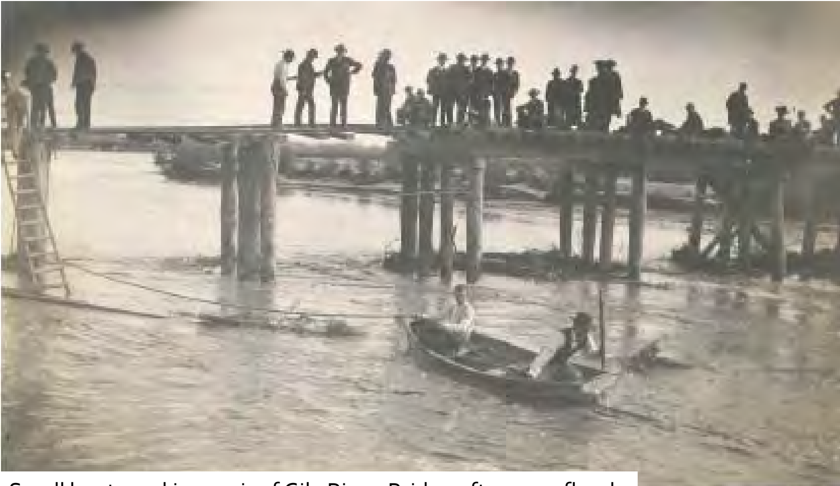
Small boat used in repair of Gila River Bridge after 1905 flood. From Littlefield, 2014
