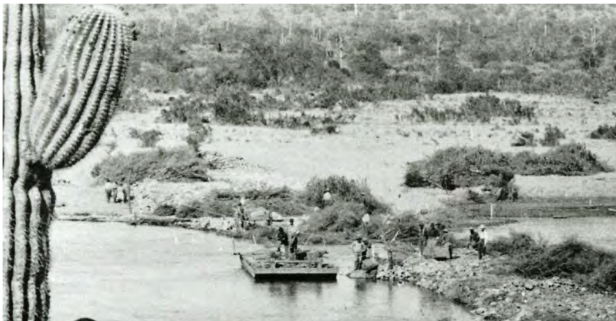
Figure 83: Close-up view of flat-bottomed skiff working on Arizona Canal Diversion Dam, 1885. Note Line across open channel of Salt River being used to pull skiff. Source: Special Collections, Arizona State University, Tempe, Arizona.
