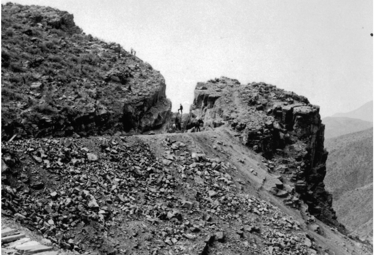
Figure 46: Work on excavating notch on Roosevelt Road above Roosevelt Dam site, ca. 1906. Source: Records of the U.S. Bureau of Reclamation, U.S. National Archives branch, Denver Colorado.
