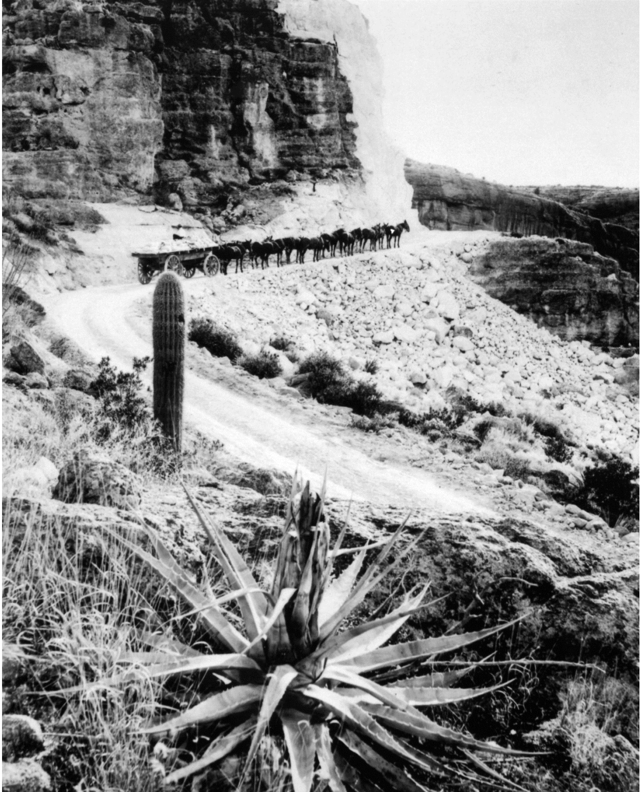
Figure 34: Top of Fish Creek Hill on wagon road to Roosevelt Dam site, March 1907. Source: Records of the Bureau of Reclamation, U.S. National Archives Branch, Rocky Mountain Region, Denver, Colorado.
