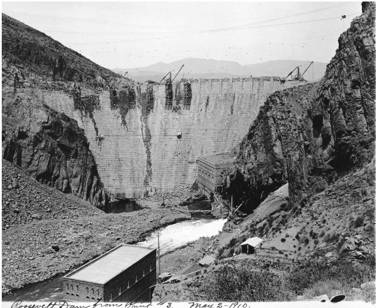
Roosevelt Dam from Point #3, May 2-1910. Figure 27: Roosevelt Dam nearing completion, May 2, 1910. Source: Records of the Bureau of Reclamation, U.S. National Archives Branch, Rocky Mountain Region, Denver, Colorado.
