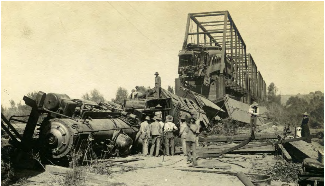
Figure 34: Train wreck on Salt River railroad bridge, 1902. Note that the engine and men are standing in the Salt River's bed. Source: Special Collections, Arizona State University, Tempe, Arizona.
