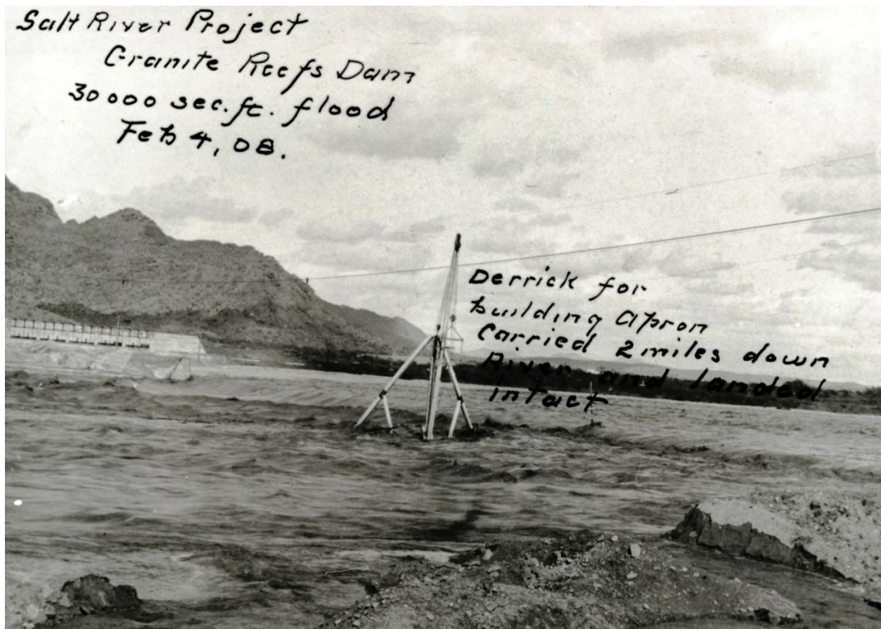
Figure 71: Flood damage at Granite Reef Dam (then under construction), February 4, 1908. Source: Salt River Project Archives, Tempe, Arizona.
