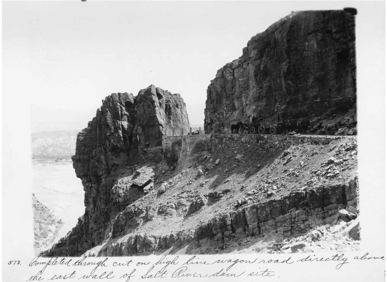
Figure 47: Completed through cut on high line wagon road directly above the east wall of the Salt River dam site, 1907 (viewed from opposite side of cut from previous illustration). Source: Records of the U.S. Bureau of Reclamation, U.S. National Archives branch, Denver, Colorado.
