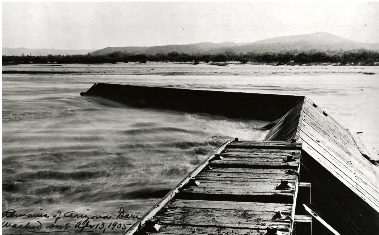
Figure 39: Remains of Arizona Dam, washed out April 13, 1905. Source: Salt River Project Archives, Phoenix, Arizona.
