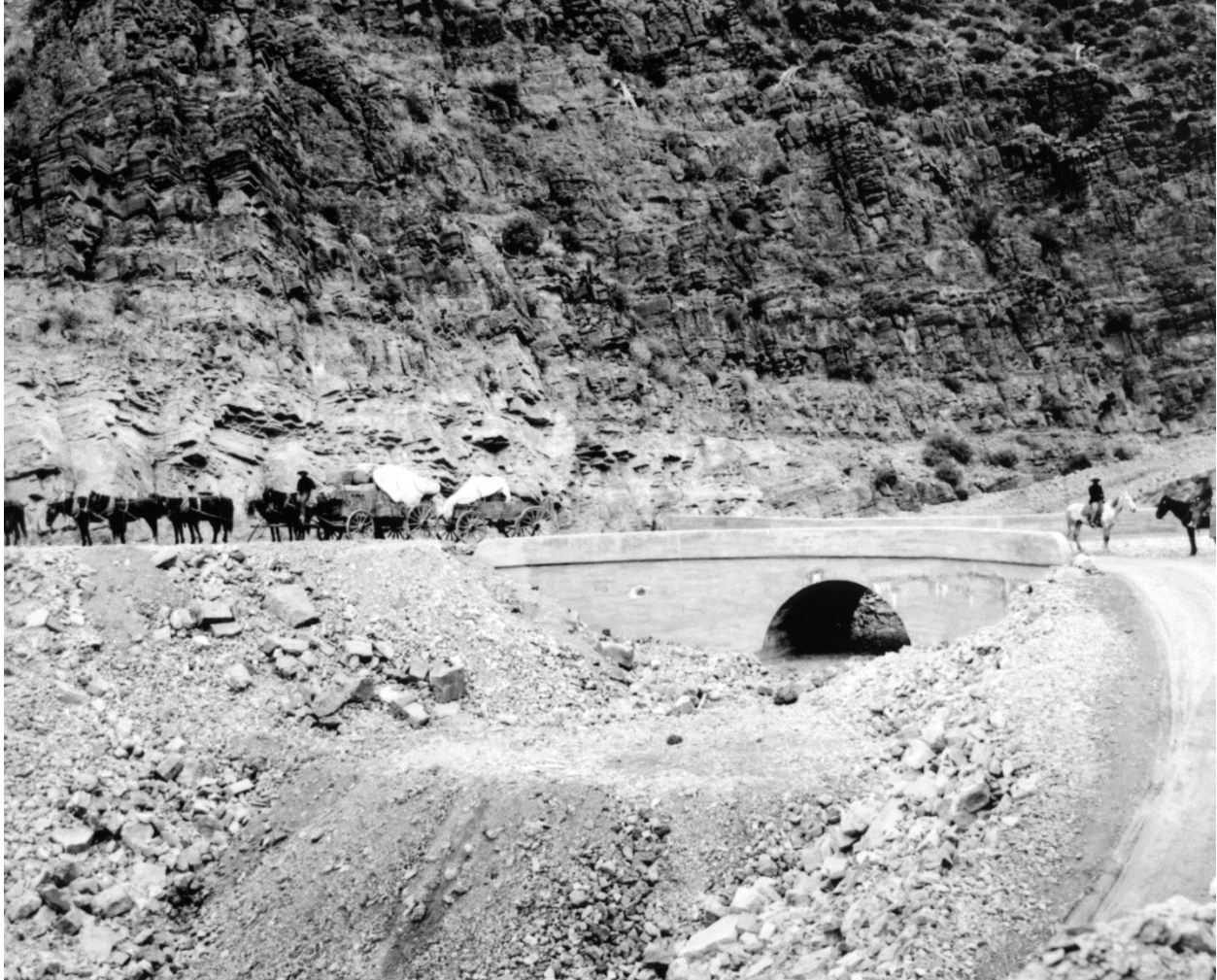
Figure 33: Whitney's Bridge on high line supply road to Roosevelt Dam site, December 1, 1906. Source: Records of the Bureau of Reclamation, U.S. National Archives Branch, Rocky Mountain Region, Denver, Colorado.
