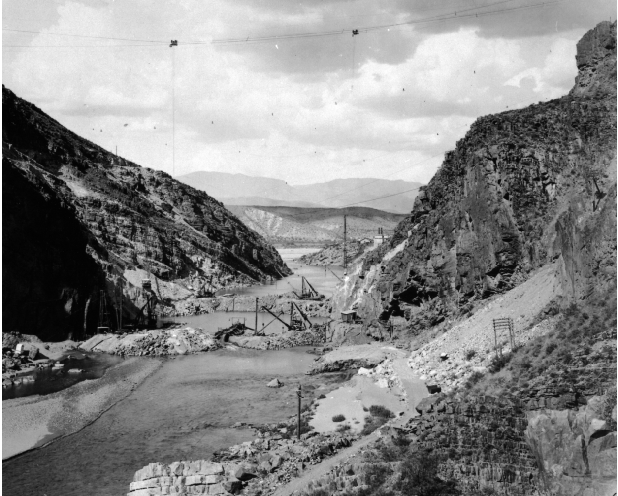
Figure 44: Roosevelt Dam under construction, July 27, 1906. There were no objections by navigation interests to the construction of the dam found in any Reclamation Service records. Source: Records of the U.S. Bureau of Reclamation, U.S. National Archives branch, Denver, Colorado.
