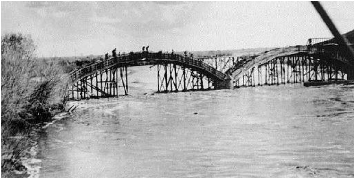
Figure 76: Ash Avenue Bridge between Phoenix and Tempe under construction using convict labor, 1912. Note heavy flow in Salt River. Source: U.S. Library of Congress, Washington, D.C.
