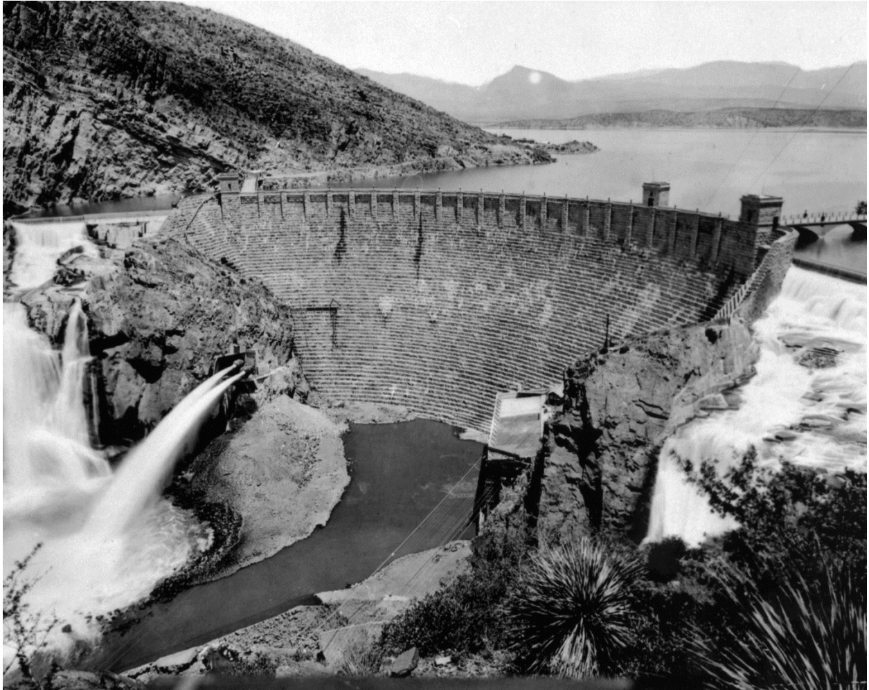
Figure 74: Roosevelt floodways overflowing, 1912. Source: Records of the U.S. Bureau of Reclamation, U.S. National Archives branch, Denver, Colorado.
