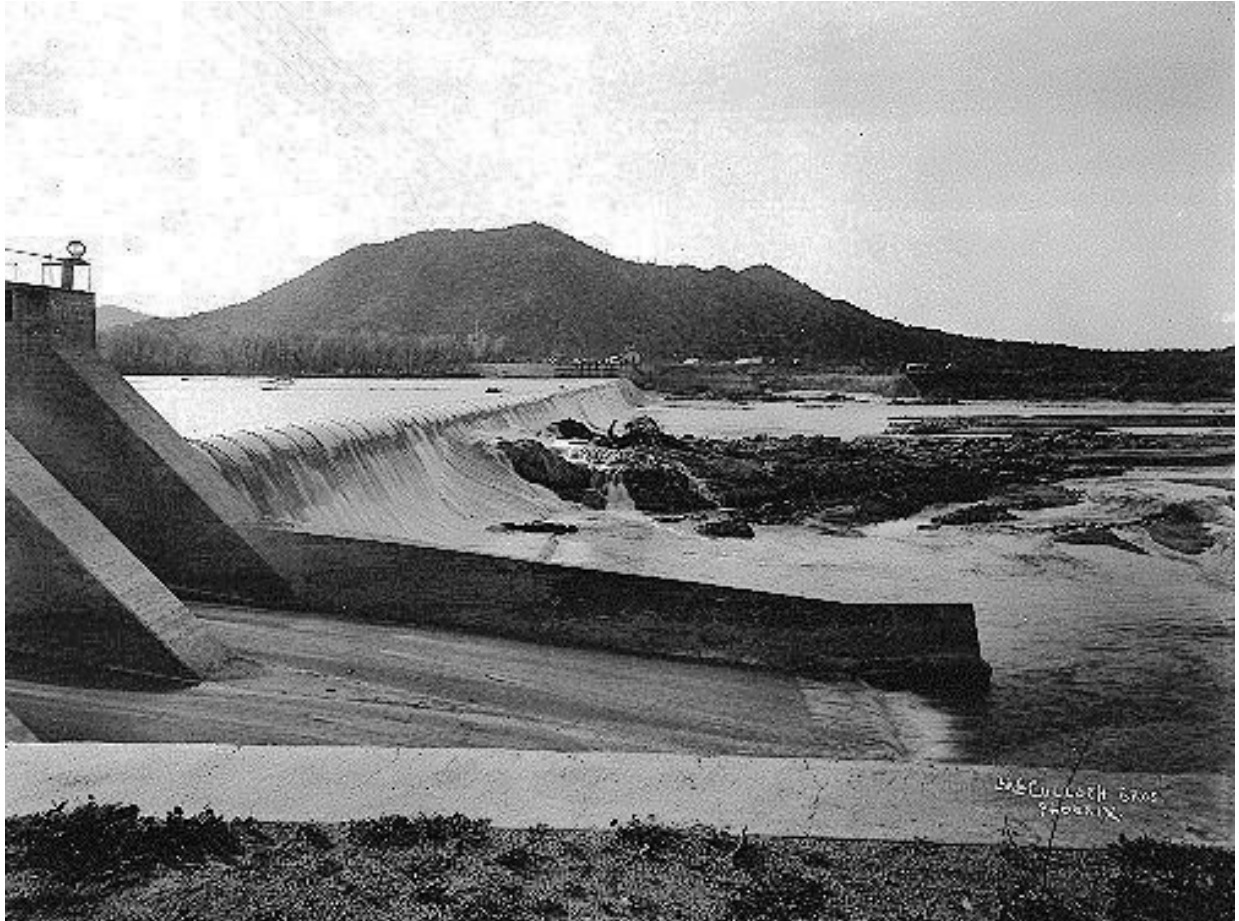
Figure 51: Granite Reef Dam after completion, ca. 1909. Source: Phoenix Public Library, Phoenix, Arizona.
