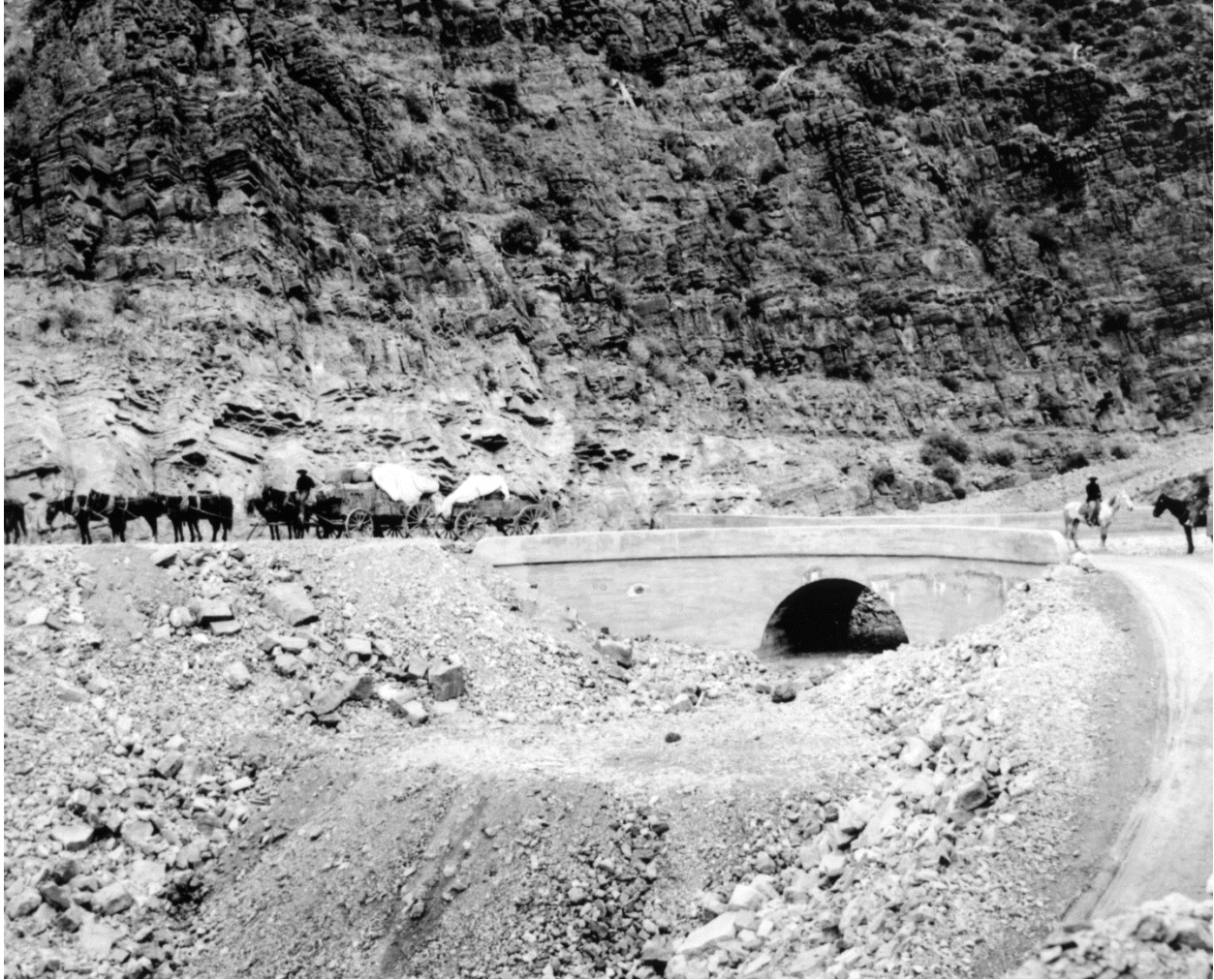
Figure 54: Freighting supplies to Roosevelt Dam site along the Roosevelt Road, 1906. Source: Records of the U.S. Bureau of Reclamation, U.S. National Archives branch, Denver, Colorado.
