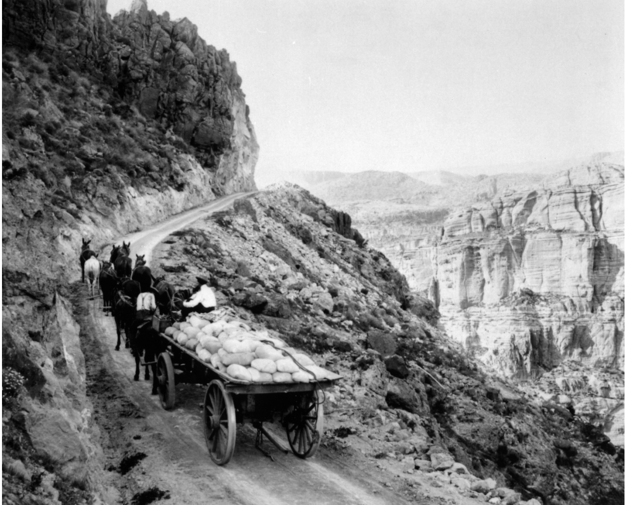
Figure 55: Hauling sacks of concrete down from site of Roosevelt Dam to Granite Reef Diversion dam site, ca. 1907. Not only did the Reclamation Service have to haul supplies up to the Roosevelt Dam site, but the Service also had to carry concrete down from Roosevelt, where the Service's concrete plant was located. The river was not used to convey materials in either direction. Source: Records of the U.S. Bureau of Reclamation, U.S. National Archives branch, Denver, Colorado.
