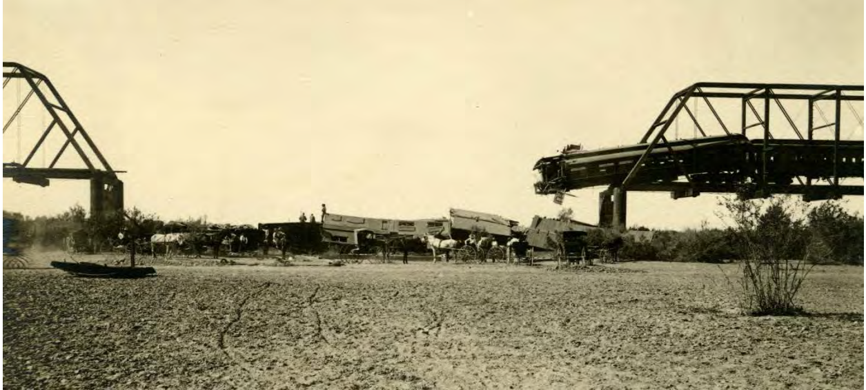
Figure 33: Train wreck on Salt River railroad bridge, 1902. Also observe the height of the concrete towers supporting the bridge and compare to how little of those towers appear during floods. Source: Special Collections, Arizona State University, Tempe, Arizona.
