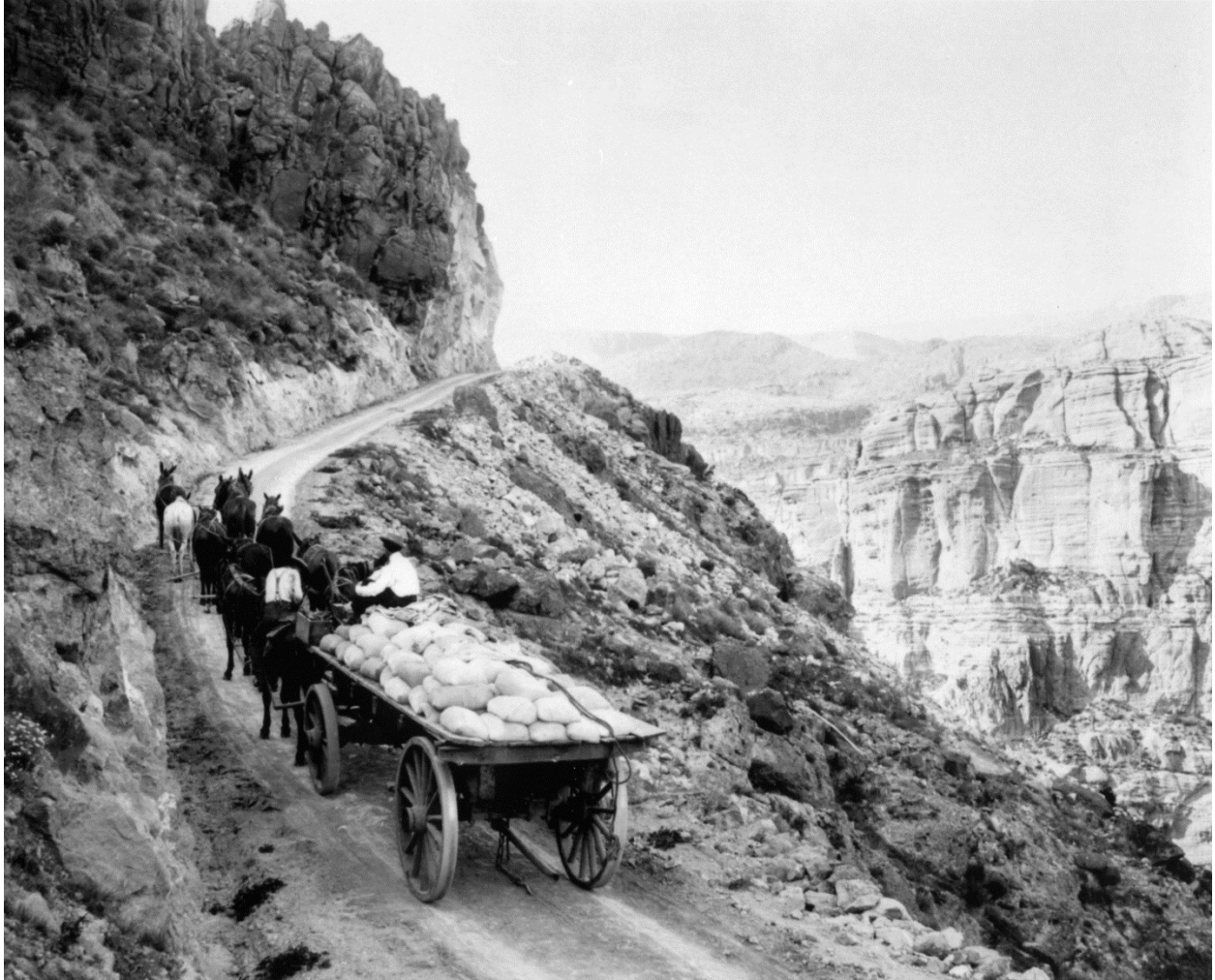
Figure 32: Hauling supplies to Roosevelt Dam site, 1907. Source: Records of the Bureau of Reclamation, U.S. National Archives Branch, Rocky Mountain Region, Denver, Colorado.
