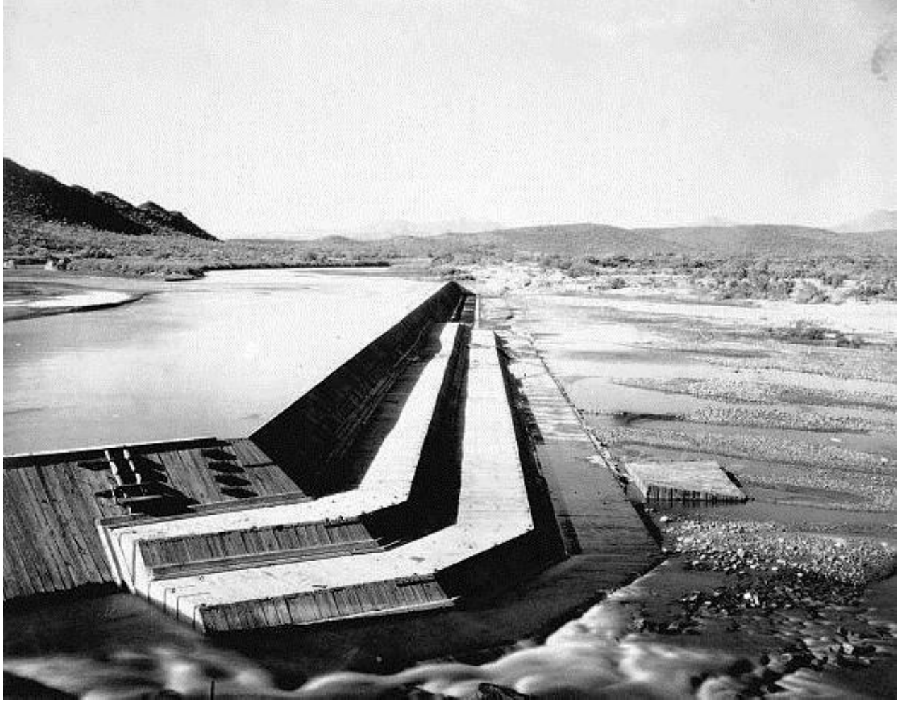
Figure 38: Arizona Canal wood-crib diversion dam, 1902. Source: U.S. Library of Congress, Washington, D.C.
