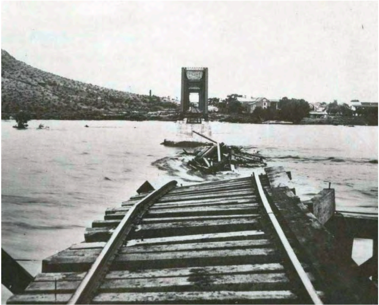
Figure 70: Salt River railroad bridge destroyed by April 1905 flood. Source: Arizona Memory Project (online photographs from multiple archival sources).
