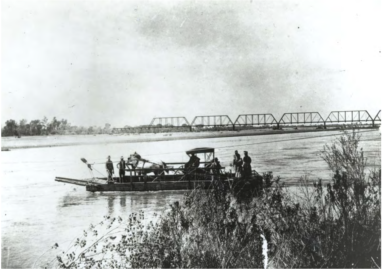
Figure 58: Charles T. Hayden's ferry between Phoenix and Tempe, 1895. Note the line used to move ferry across the Salt River. Source: Special Collections, Arizona State University, Tempe, Arizona.
