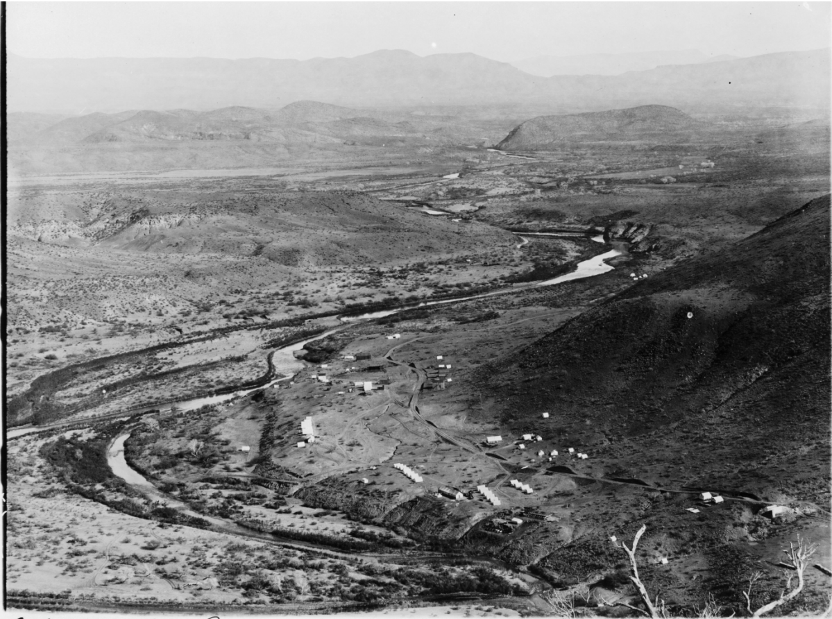
Looking up Salt River, showing junction of Salt and Tonto Rivers, and location of camp at dam site. Jan. 14-1904.
