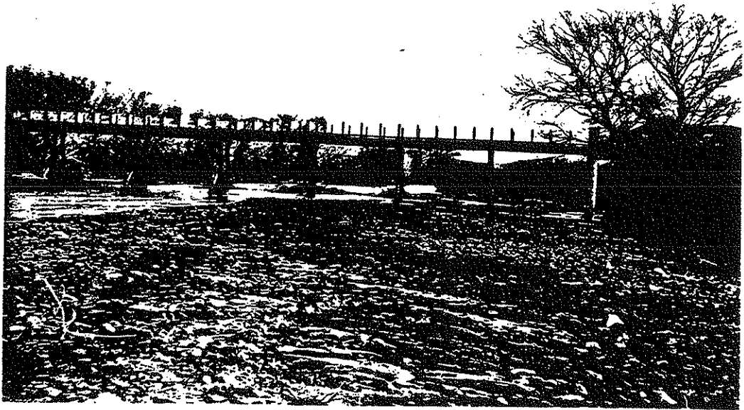
View looking upstream showing channel past gage and bridge from which measurements are made. Only a small stream flows past the gage at present. December 2, 1930.
