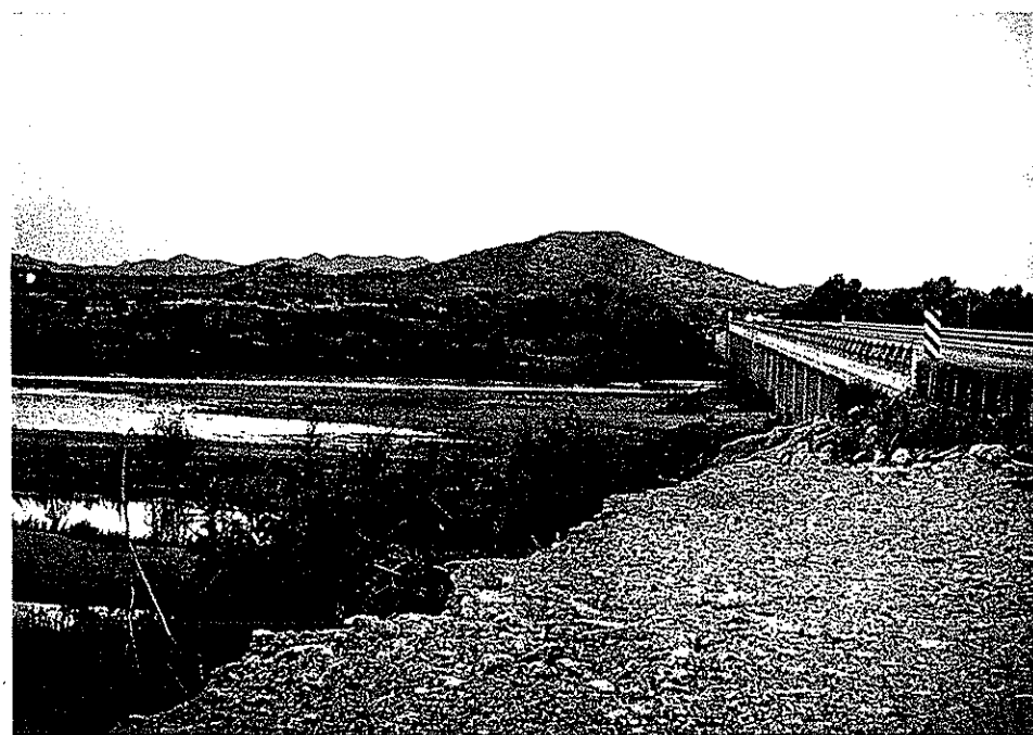
Old Highway 85 Bridge
