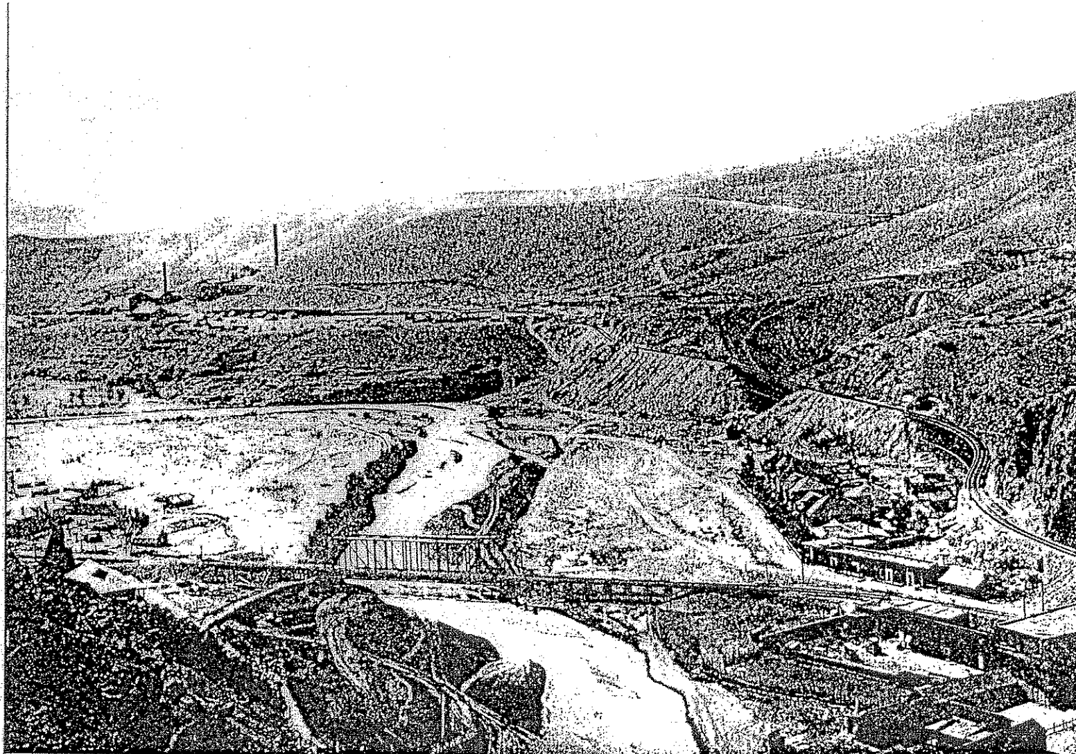
South Clifton, Shannon Works in the distance, A. & N. M. Railway Bridge. Segal (n.d.)
