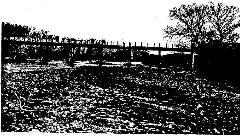
View looking upstream showing channel past gage and bridge from which measurements are made. Only a small stream flows past the gage at present. December 2, 1930.
