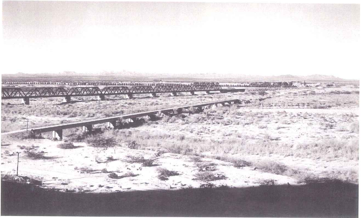
Photograph of Gila River Channel Near Antelope Hill, January 16, 1940, Records of the U.S. Bureau of Reclamation, U.S. National Archives Branch, Rocky Mountain Region, Denver, Colorado
