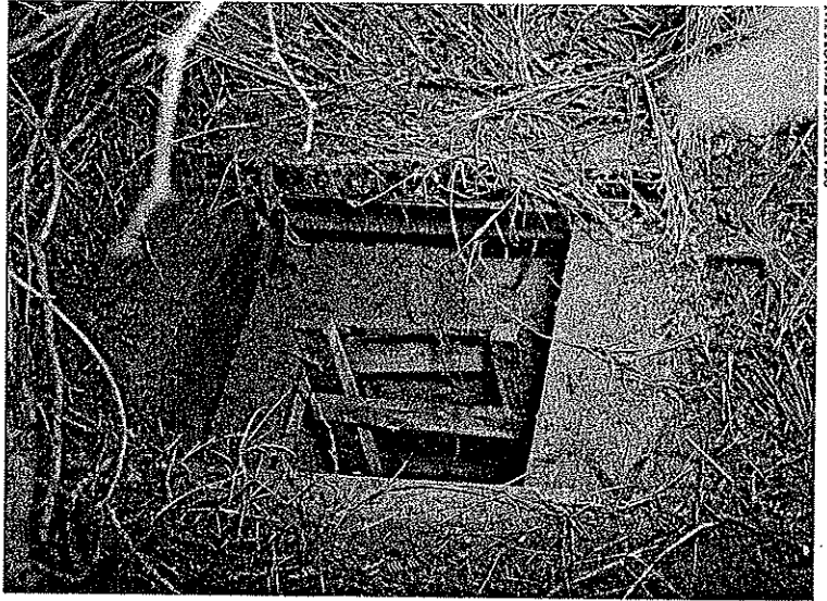
The carefully constructed exit. Dirt-filled boxes covering this opening held grass and weeds cultivated to blend with the surrounding area.
