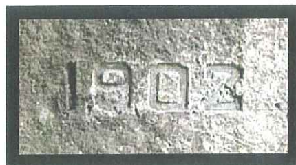
1902 Date Carved In Northern Abutment
