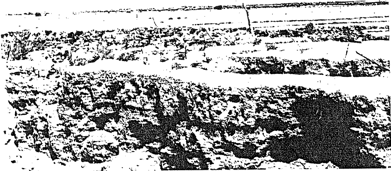
Figure 10-7. Entrenchment in the San Simon Valley in eastern Arizona. The vertical walls are 3 to 4 m. The photograph was taken about 12 km upstream from the mouth in the mid-1960s by Bureau of Land Management personnel.
