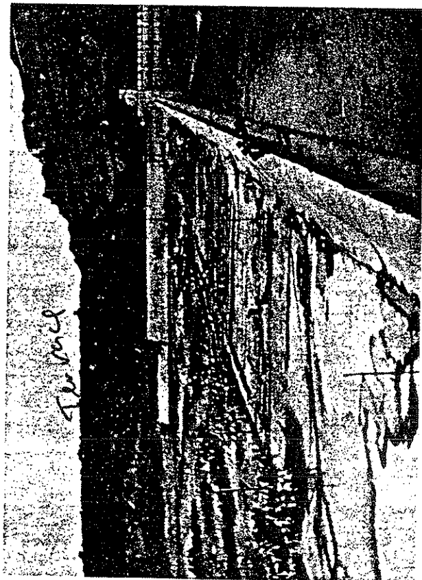
Figure 4.4 Reconstruction of the Granite Reef Dam splash apron after it was removed during the 1920 flood. The photo was taken on February 2, 1920 (photograph courtesy of the Arizona Historical Foundation, Arizona State University, Gregory Collection, QD-50 1990).
