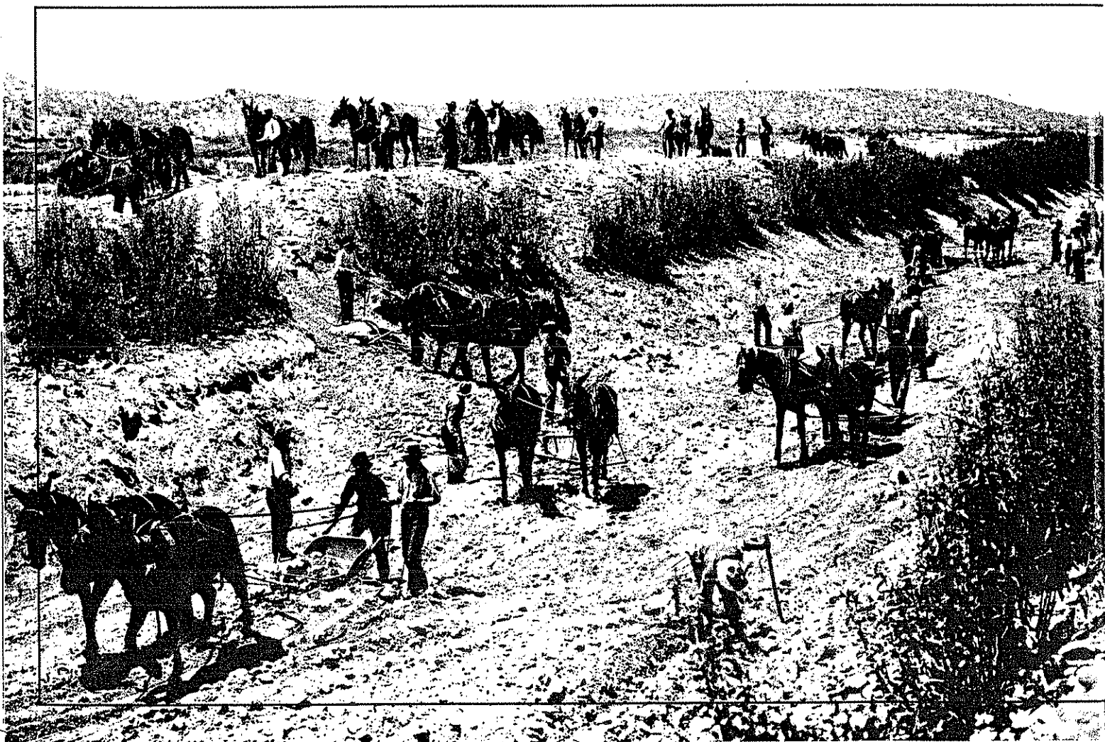
U.S. Reclamation Service crews enlarge the Arizona Canal in June 190
