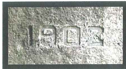
1902 Date Carved In Northern Abutment
