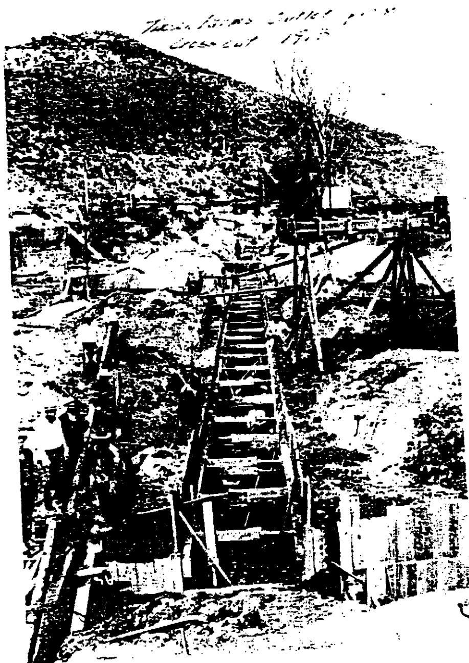
Figure 43. Outlet from the Crosscut in the streambed of the West Branch in 1913 (Photograph by Percy Jones, Special Collections, University of Arizona Library, Tucson, Negative No. 2709; U.S.G.S. Stake 1066).
