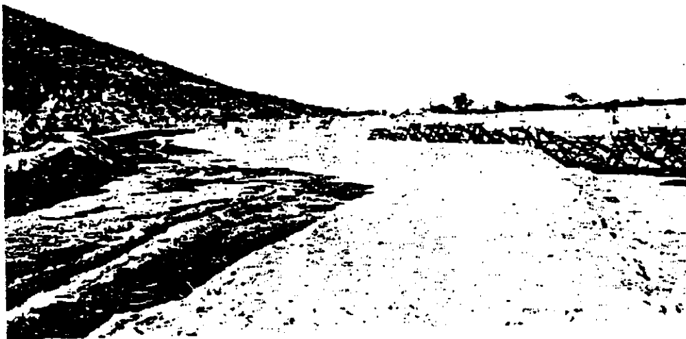
Figure 70. In 1935, the Works Projects Administration (WPA) constructed several flood control features along the Santa Cruz River. In the reach just south of Sentinel Peak (left), the river's flow was deflected into pilot channels by means of revetments, in this case fashioned from old automobile frames (right). By the following year, summer flows had filled the area behind the revetment with about 1 m of sediment. The intent was to eliminate sharp meanders and to reclaim the areas they incorporated for cultivation (Photograph by R.C. Baker, State of Arizona Archives, Phoenix, U.S.G.S. Stake 1074).
