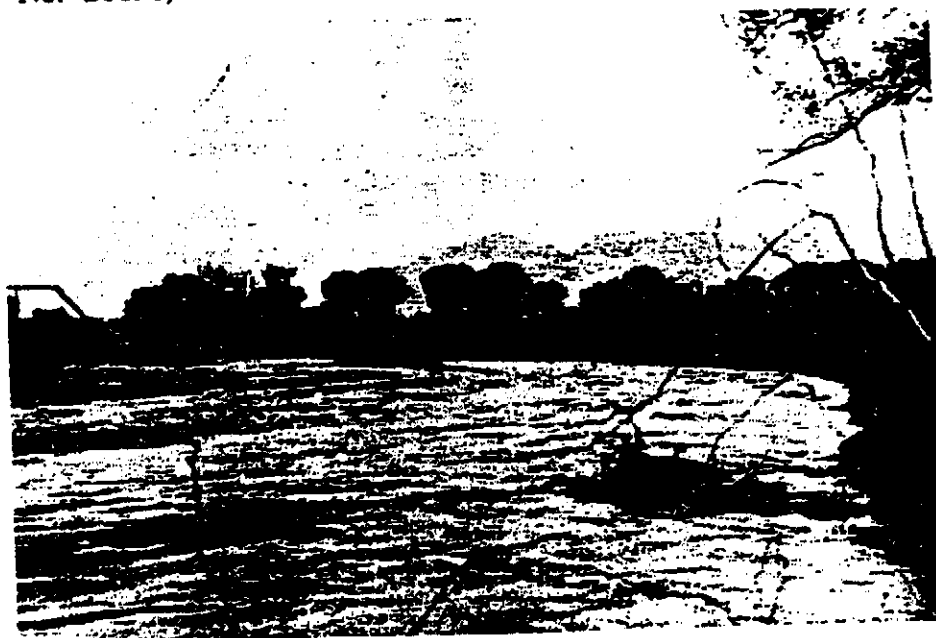
Figure 30. Downstream view of the Santa Cruz river in 1902. This photograph shows active erosion where the meandering thalweg strikes the right bank. Congress Street is on far left and is seemingly in a precarious position should the meander continue eroding downstream. The Santa Catalina Mountains are in the background (Arizona Historical Society, Tucson, Negative No. 26699).
