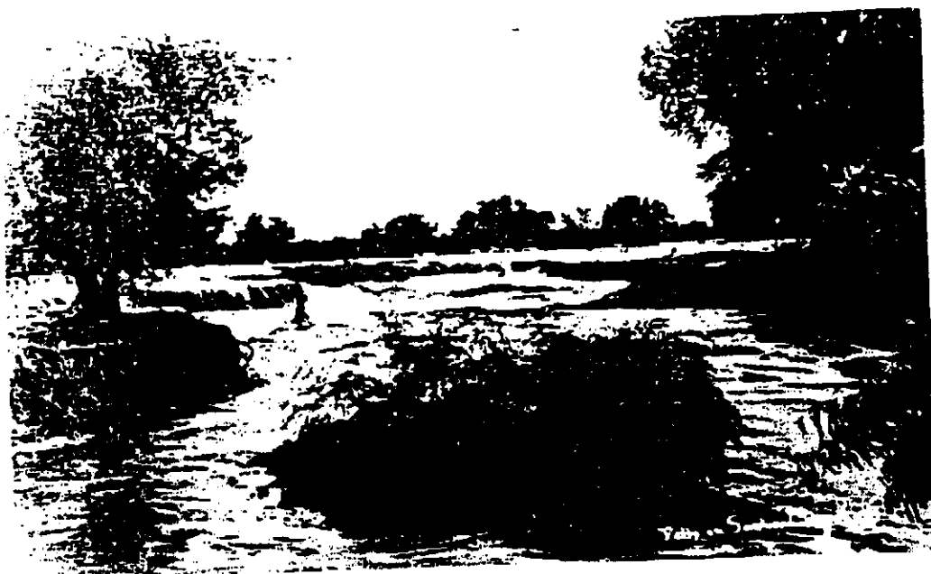
Figure 22. Upstream view of the heading of Sam Hughes' intercept ditch at the St. Mary's Road crossing in October 1889. The heading here behaved as a headcut actively eroding even with minor flooding. Note that in 1889, this reach was unentrenched and even moderate flows would inundate the valley (Photograph by H. Buchman, Special Collections, University of Arizona Library, Tucson).
