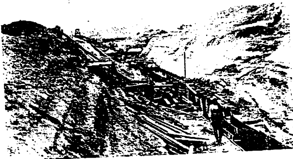
Figure 42. West view of the Crosscut under construction in 1912 (Photograph by Percy Jones, Special Collections, University of Arizona Library, Tucson, Negative No. 2758).
