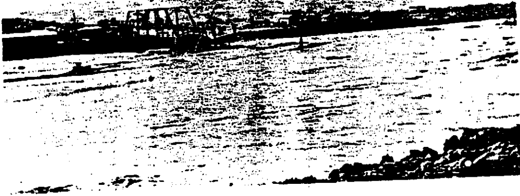
Figure 54. The Congress Street Bridge after erosion of east bank in January 1915, looking northwest. The cottonwood stand evident in 1902 (Fig. 29) was completely removed during the 1915 flood (Special Collections, University of Arizona Library, Tucson).
