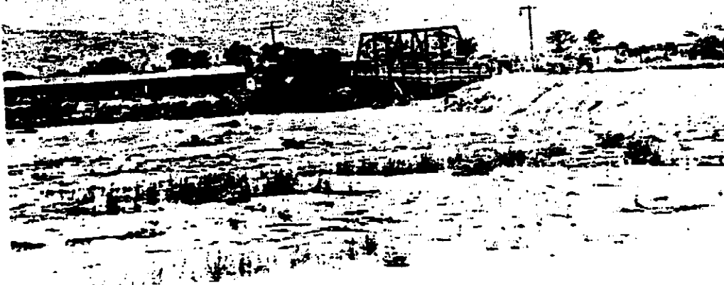
Figure 55. A similar view as Figure 54 in July 1915. A berm was built to join the east approach to the bridge (Special Collections, University of Arizona Library, Tucson).
