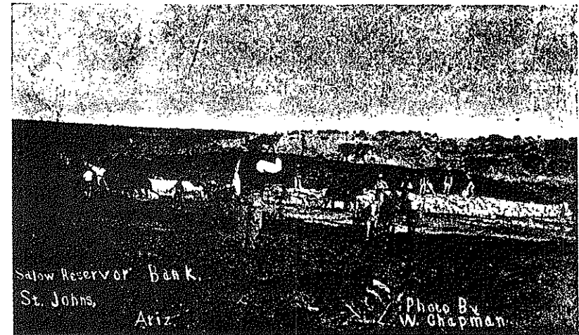
RESERVOIR BUILDING OPERATIONS
