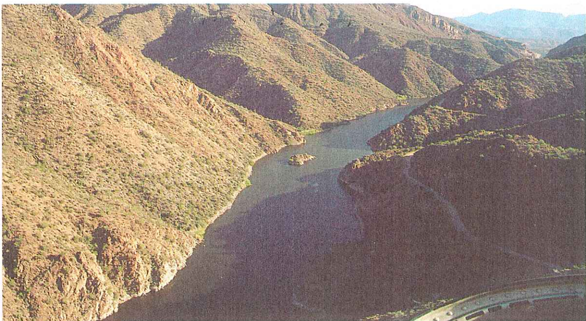
Figure 6. Salt River downstream of Roosevelt Dam. Note bedrock island.
