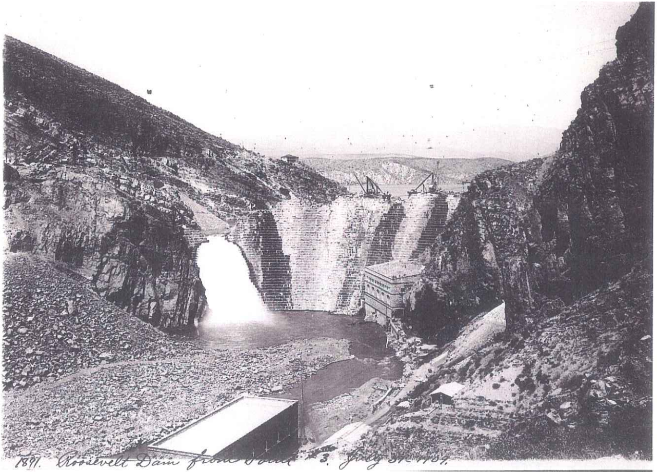
Photograph of "Roosevelt Dam from Point #3 [Looking Upstream]," July 31, 1909, Records of the Bureau of Reclamation, U.S. National Archives Branch, Rocky Mountain Region, Denver, Colorado
