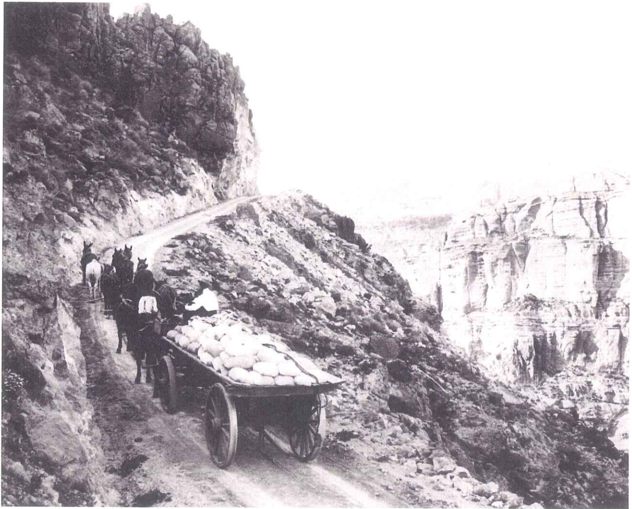
Photograph of "Meeting a 12 Horse Freighting Outfit Coming Up Fish Creek Hill, Ariz. 11,000 lbs. Being Shipped from Govt. Cement Plant at Roosevelt, Ariz. to Granite Reef, Ariz." March 27, 1907, Records of the Bureau of Reclamation, U.S. National Archives Branch, Rocky Mountain Region, Denver, Colorado
