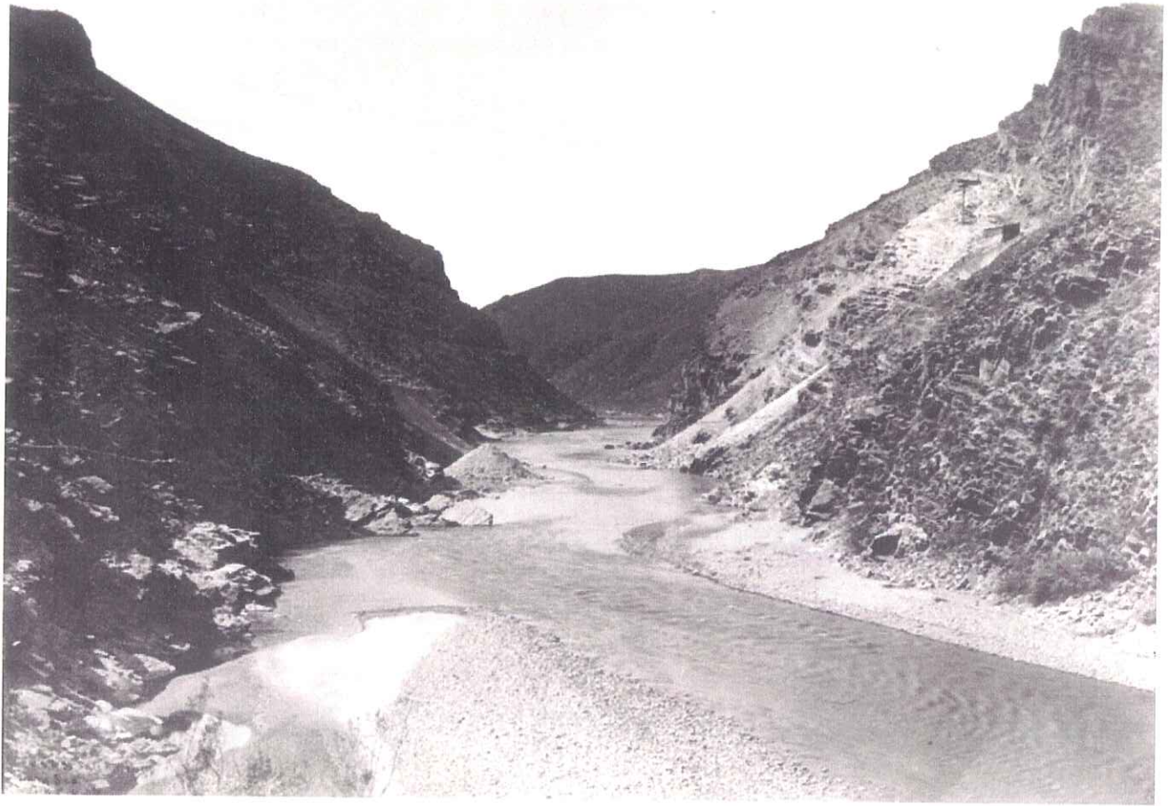
Photograph of "Roosevelt Damsite Looking Downstream," March 6, 1906, Records of the Bureau of Reclamation, U.S. National Archives Branch, Rocky Mountain Region, Denver, Colorado
