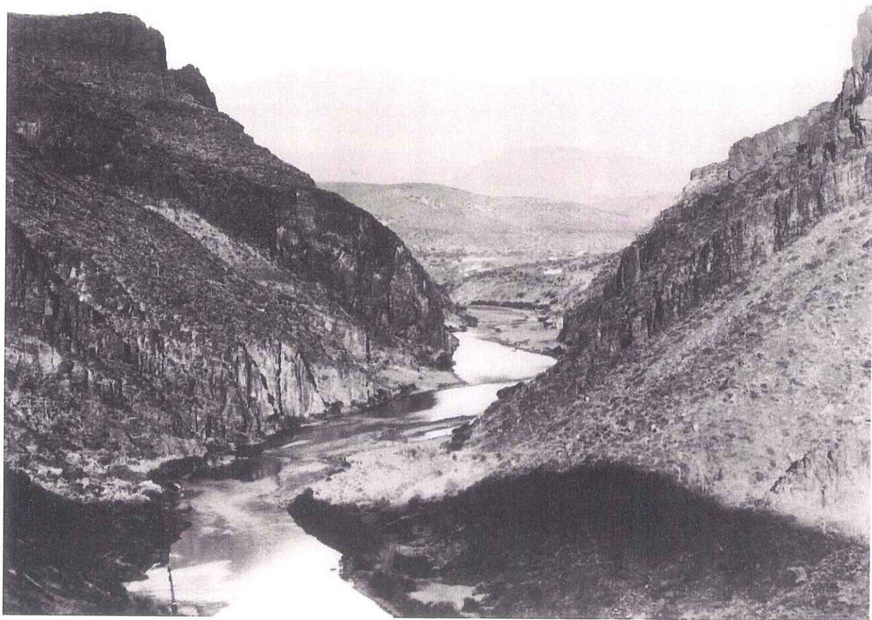
Photograph of "Canyon just below Damsite, Showing Damsite," January 16, 1904, Records of the Bureau of Reclamation, U.S. National Archives Branch, Rocky Mountain Region, Denver, Colorado
