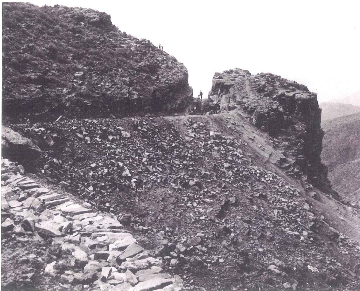
Photograph of "View Showing Construction on High Line Wagon Road Directly above Salt River Dam Site on East Side of Canyon," March 29, 1905, Records of the Bureau of Reclamation, U.S. National Archives Branch, Rocky Mountain Region, Denver, Colorado
