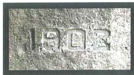
1902 Date Carved In Northern Abutment
