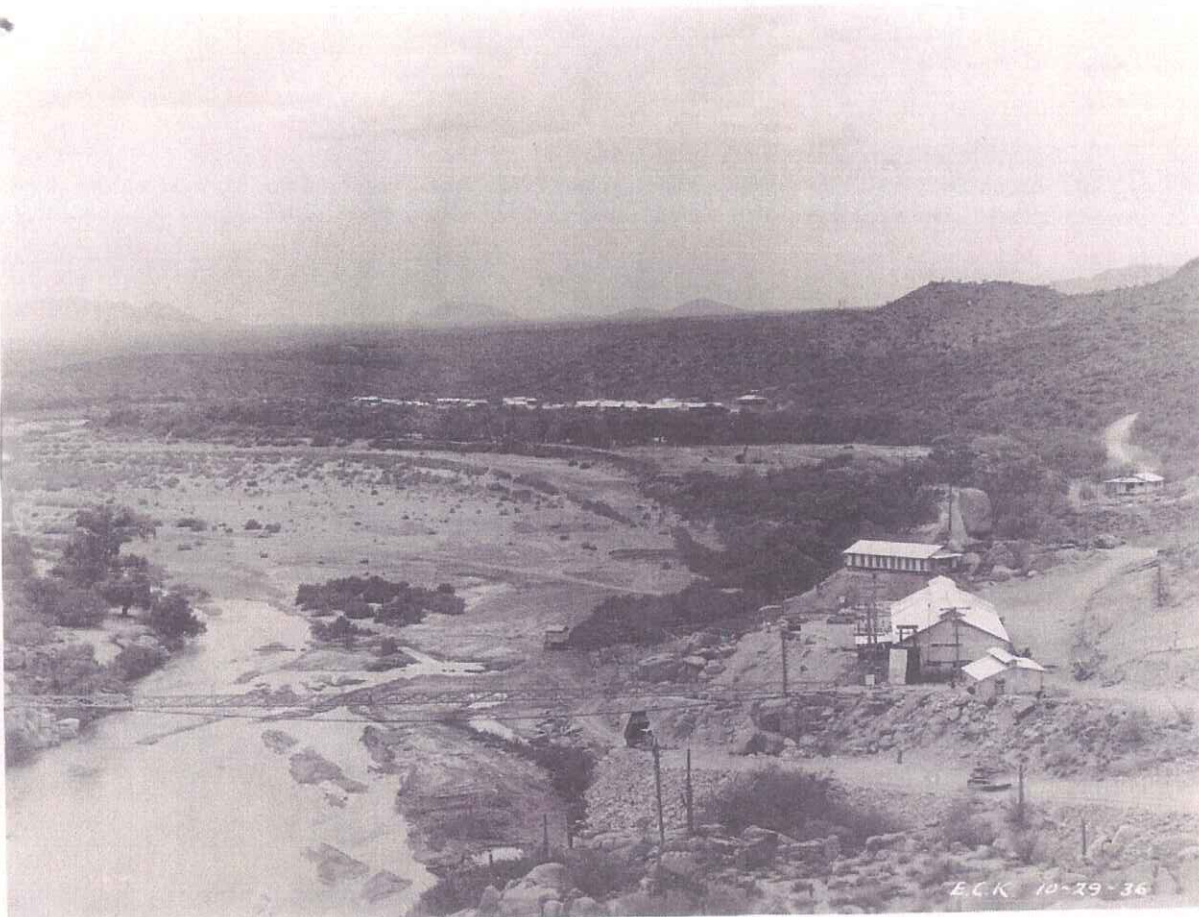
Figure 63. Photograph of “Bartlett Dam Site Looking Downstream on the Verde,” 1936, Records of the U.S. Bureau of Reclamation, National Archives branch, Rocky Mountain Region, Denver, Colorado
