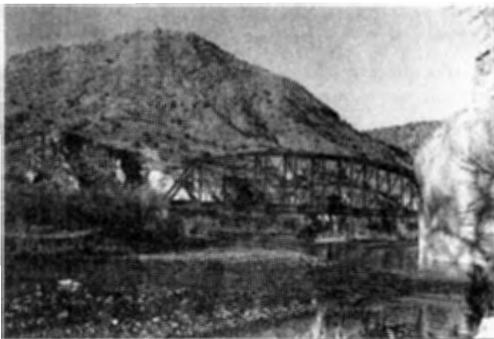
~ Looking Down at the Perkinsville Railroad Bridge - Mile 26.5 ~ poses only.
