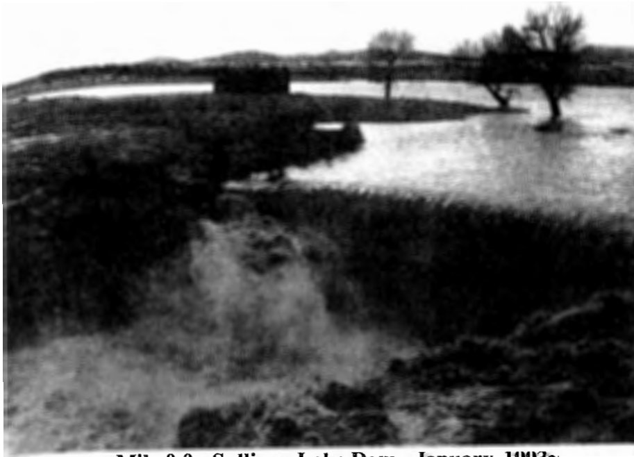
~Mile 0.0 - Sullivan Lake Dam - January, 1993~
