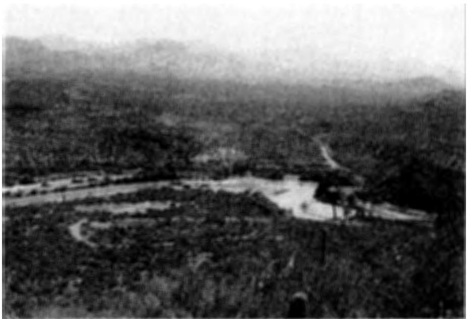
~ FR269 Overlook into Sheep Bridge area ~
