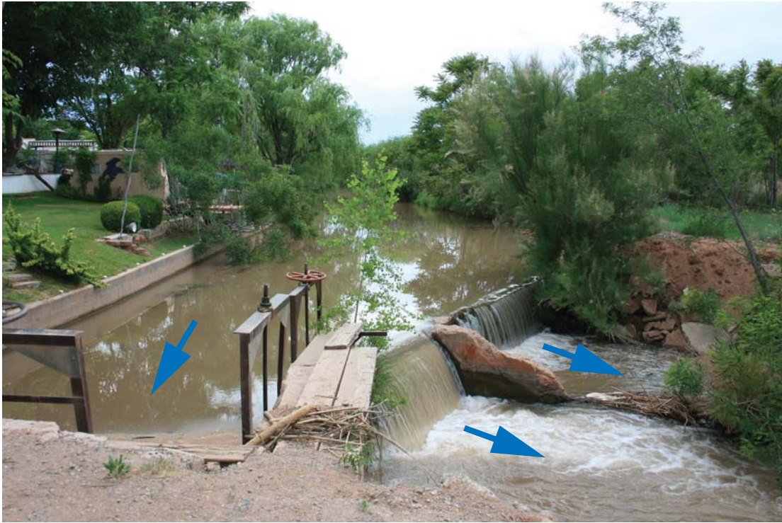
Figure 8 - Verde Ditch head gate and spillway. Initial spillway is on right side of picture, while the head gate is on the lower left side. Note the large percentage of flow that the spillway is returning to the river. Blue arrows indicate flow direction.
