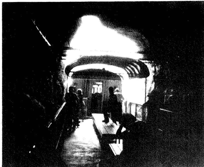
~ Mile 30 - Railroad Tunnel ~
