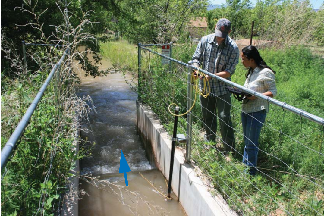
Figure 28 - Example of pressure transducer deployed at head gate of the Eureka Ditch, Camp Verde, central Arizona. This deployment is down the ditch from the head gates, and is above the first water user. This site is located within a concrete weir, and the site is also utilized by Salt River Project (SRP) as a gauging station. Blue arrow indicates flow direction.
