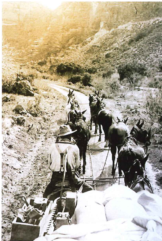
Government freight wagon at foot of Fish Creek Hill on way to dam site, 1907. (Reclamation photograph)
