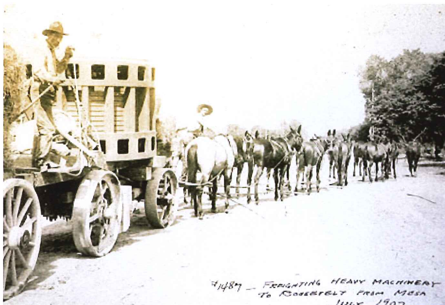
Freight wagon with generator headed for Roosevelt Dam from Mesa, 1907. (Reclamation photograph)
