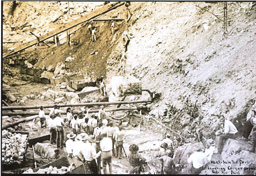
The cornerstone for Roosevelt Dam was laid September 20, 1906. (Reclamation photograph)
