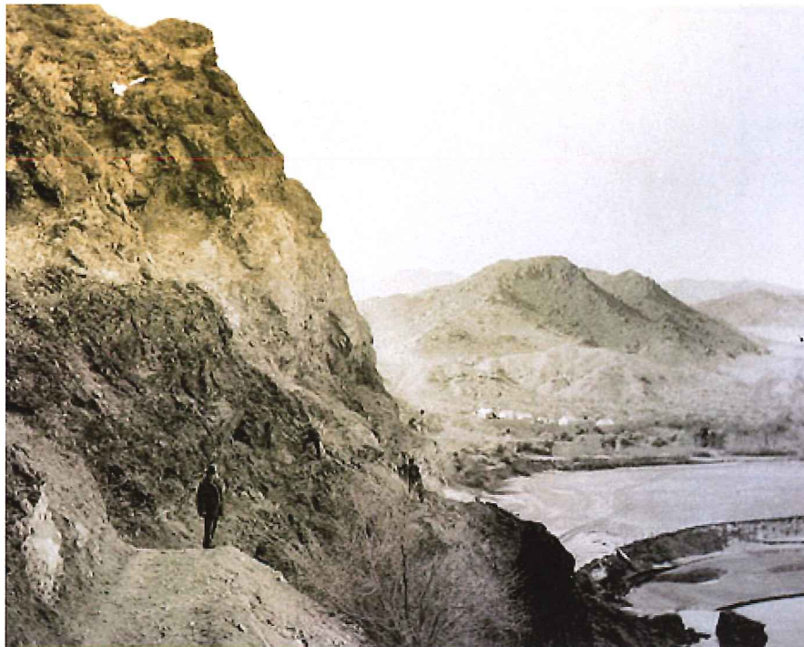
Black canyon dam site with beginnings of a construction camp in the background. (Reclamation photography)
