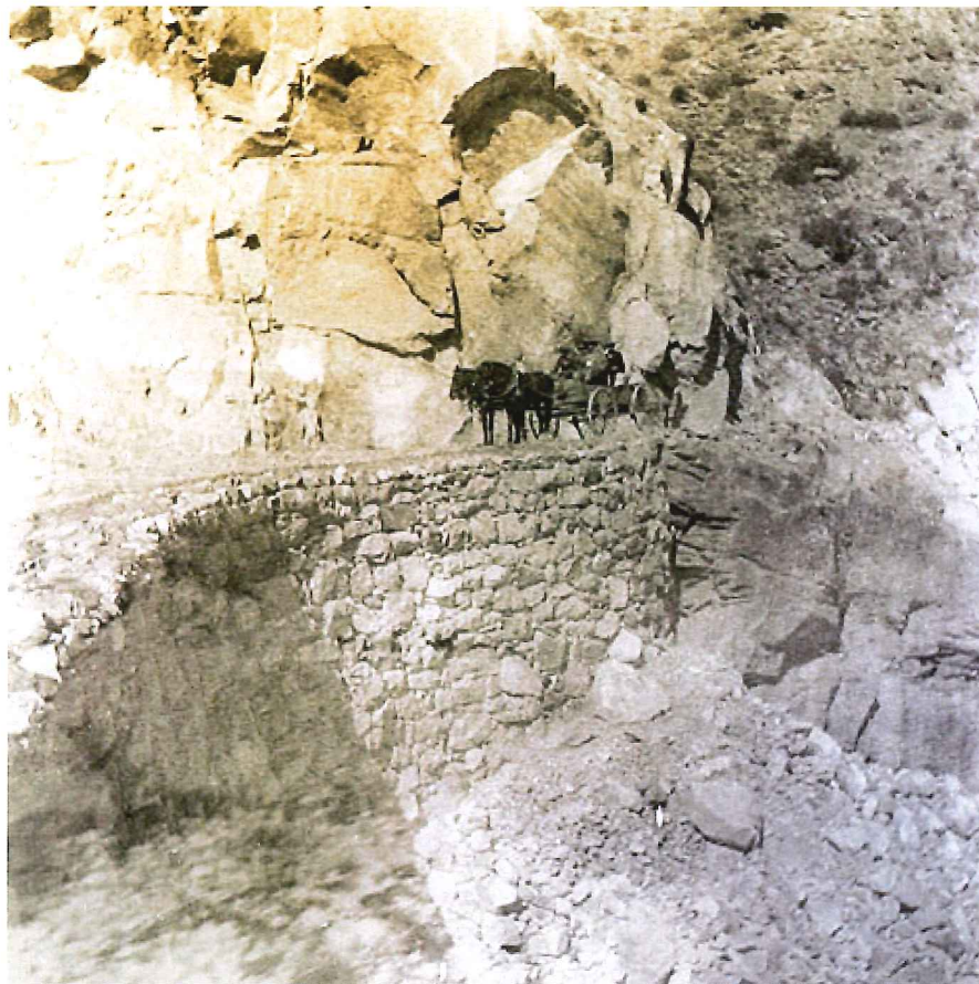
Apache workers were known for their skill in building dry-laid stone walls. Without using mortar, they constructed many such retaining walls along the various roads they built. This fine example is on Fish Creek Hill on the Mesa to Roosevelt Road, known today as the Apache Trail, 1905. (Courtesy of Salt River Project)
