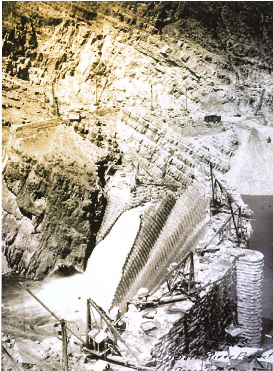
Lubken primarily documented the construction of Roosevelt Dam while in Arizona. This 1909 photograph shows the massive wall of the dam still under construction. (Reclamation photograph)
