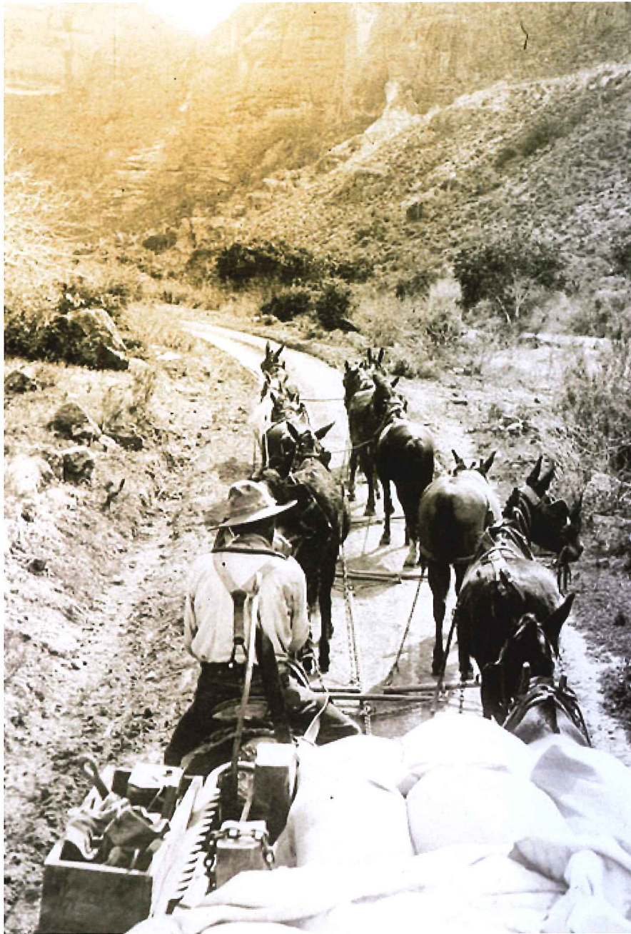
Government freight wagon at foot of Fish Creek Hill on way to dam site, 1907. (Reclamation photograph)
