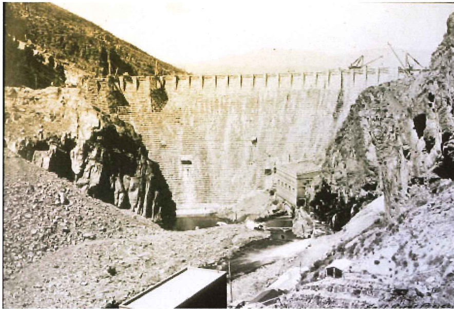
View of the dam nearing completion, 1910. (Reclamation photograph)
