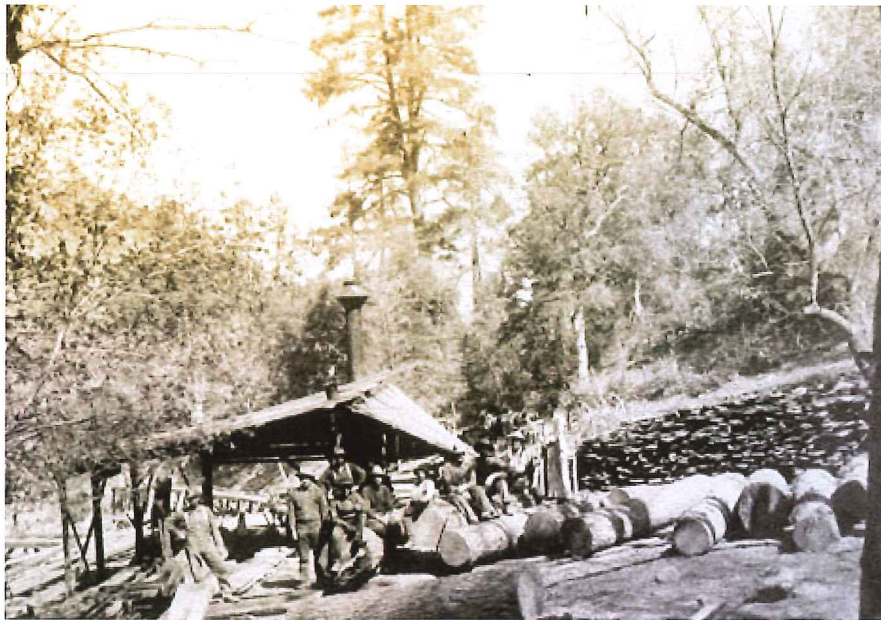
As construction got underway, the Reclamation Service established a lumber mill in the Sierra Ancha Mountains north of the Roosevelt Dam site. A local source for construction lumber was less expensive than hauling it from Mesa, 1904. (Reclamation photograph)
