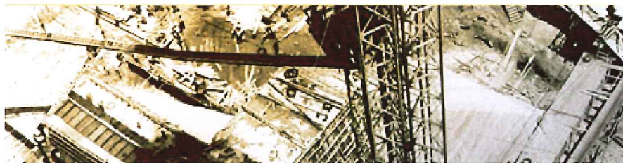
Horse Mesa Dam looking downstream, 1927. (SRP photograph)
