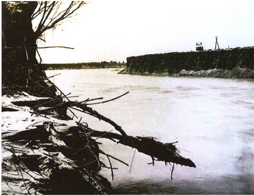
Serious erosion along the banks of the Colorado occurred when the river overflowed. (Reclamation photograph)
