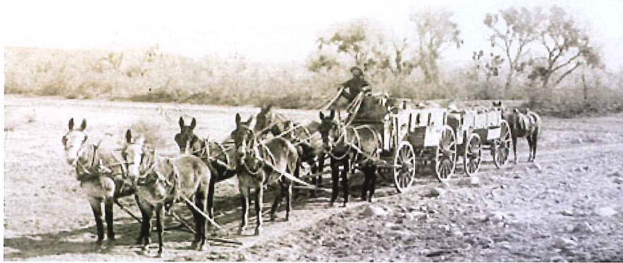
Freight wagons with mule team bringing supplies to the Roosevelt Dam site on the road from Globe, 1904. (Reclamation photograph)
