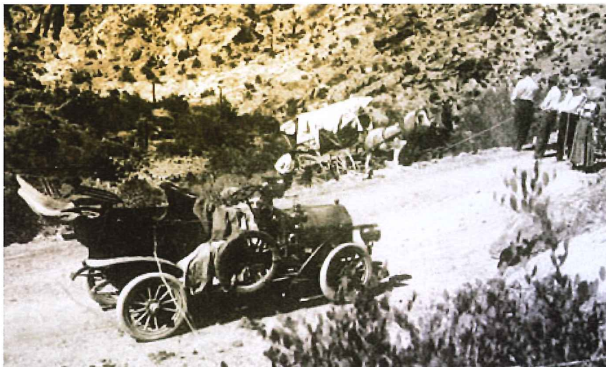
Assisting stage coach on Roosevelt Road, 1910. (Reclamation photograph)
