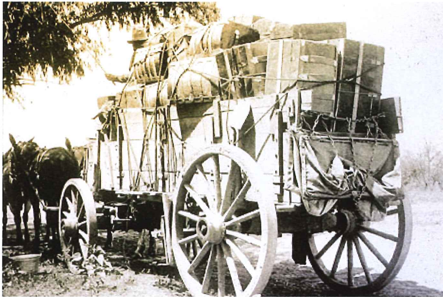
Freight wagon with luggage and baggage belonging to Italian stone masons from Pennsylvania hired to work on construction of the dam, 1906. (Reclamation photograph)
