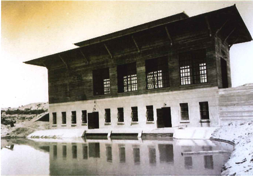
This 1922 photograph shows the forebay of the new power plant for the pump station constructed at the base of Yuma Mesa. (Reclamation photograph)
