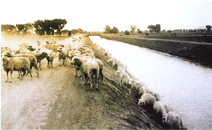
Canal maintenance was an on-going problem, and Government sheep were used to control weeds and grass along the canals, 1914. (Reclamation photograph)
