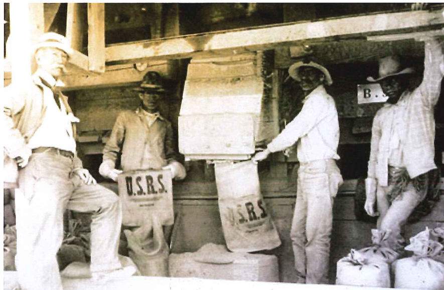
Because it was expensive to haul supplies from Mesa to the dam, the U.S. Reclamation Service built a cement plant on site, 1910. (Reclamation photograph)
