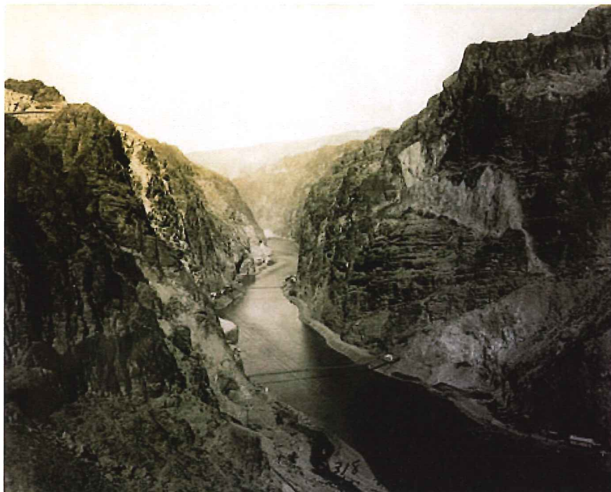
This photograph shows preliminary work on the Black Canyon site. Note portals to tunnels No.2, No. 3, and No. 4. In the upper left, a retaining wall on the road to dam, can be seen. The dam site is located at the uppermost bridge crossing the river. (Reclamation photograph)
