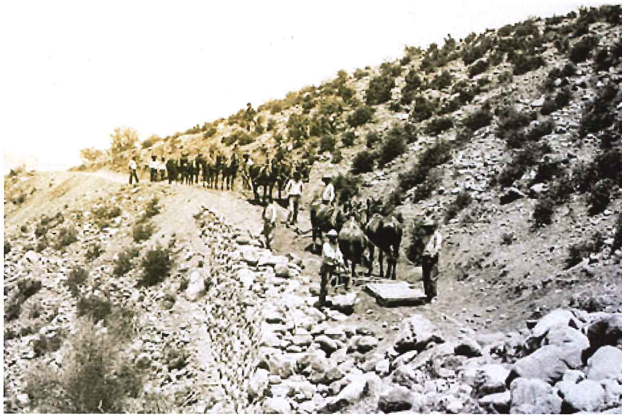
Apache teamsters placing fill on the new Tonto Highline Road. Note the dry-laid masonry retaining wall. (Reclamation photograph)
