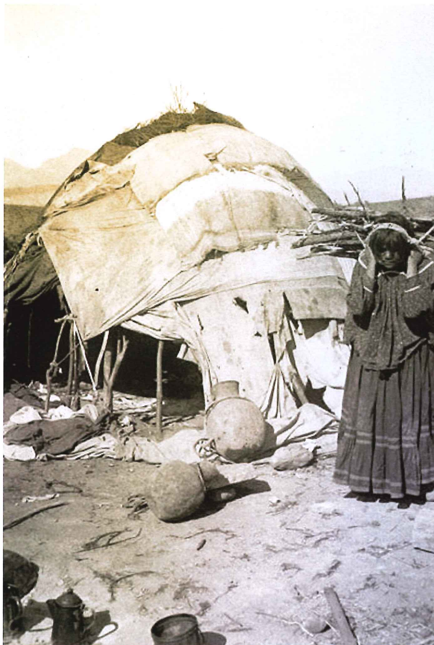
Apache workers often brought their families to live with them. They lived in a segregated area and maintained their traditional lifestyle. Here an Apache woman brings firewood to her wickiup, a structure of bent poles covered with brush that is also covered with blankets, tarps, and hides. Note the use of large ceramic storage jars and metal pots and pans, 1911. (Reclamation photograph)
