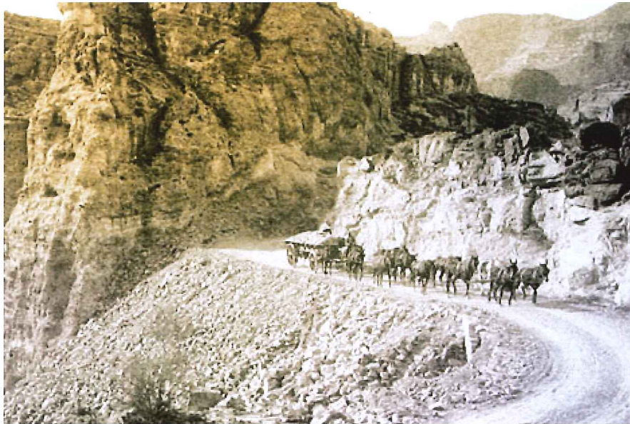
A portion of Mesa to Roosevelt Road at Fish Creek Hill. Note the extensive road work required to cut through the mountain and provide fill for a stable road bed. American Indians, primarily Apaches, constructed over 100 miles of roads to provide access for men, equipment, and supplies to the dam site, 1905. (Reclamation photograph)
