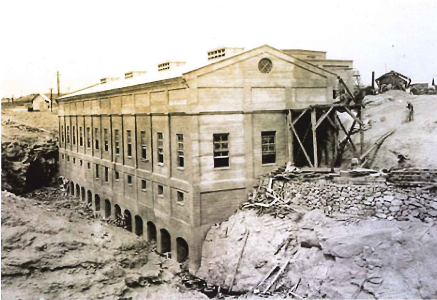
Construction of the Crosscut Powerhouse. Henry T. Cowling, 1914.
