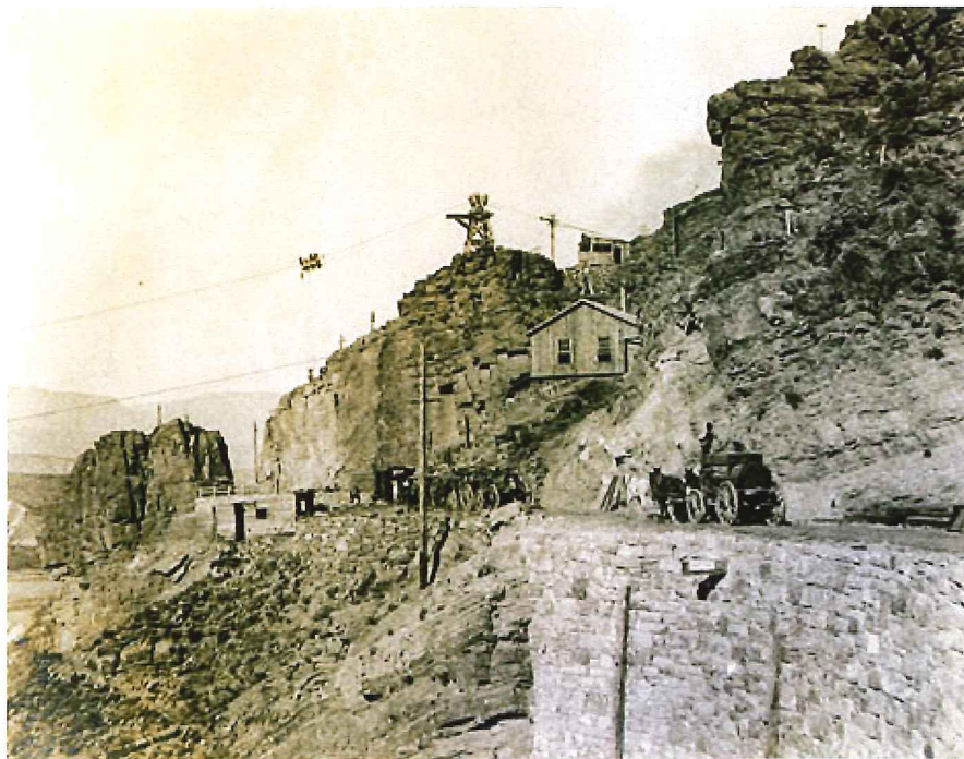
In this photograph, two freight wagons approach the construction site for the Roosevelt Dam, No date. (Courtesy of Salt River Project)
