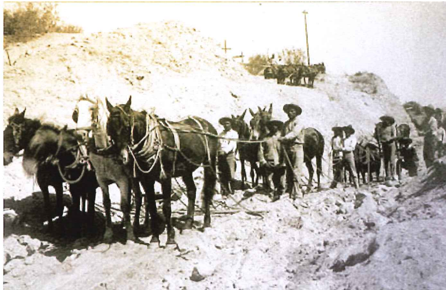
Apache workers on the cutoff canal, Roosevelt Dam site, 1909. (Reclamation photograph)
