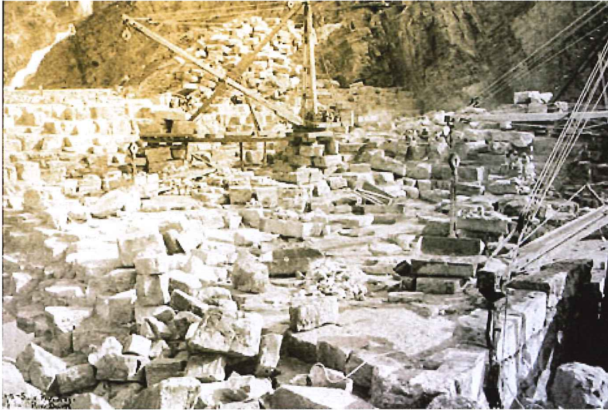
By 1907, construction of the Roosevelt Dam was well underway. (Reclamation photograph)
