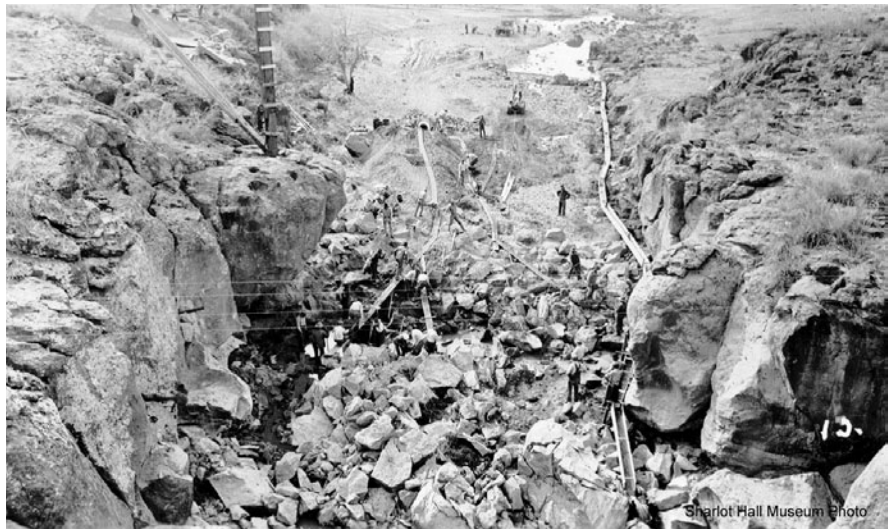
Figure 2.14 —A 1936 photo showing the early construction phase of excavating basalt rock for the base of Sullivan Dam. Perennial flow from Del Rio Springs was routed through a sluice box visible on the right side of the rock cut. (Photo courtesy of the Sharlot Hall Museum, Prescott, Arizona.)
