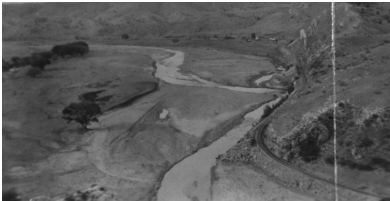
Figure 2.41 —A 1925 photograph of the Perkinsville area looking northwest along the Santa Fe Railroad (Verde River Railroad) toward the Station (light colored buildings in the upper right quadrant). (Photo courtesy of the Sharlot Hall Museum, Prescott, Arizona.)
