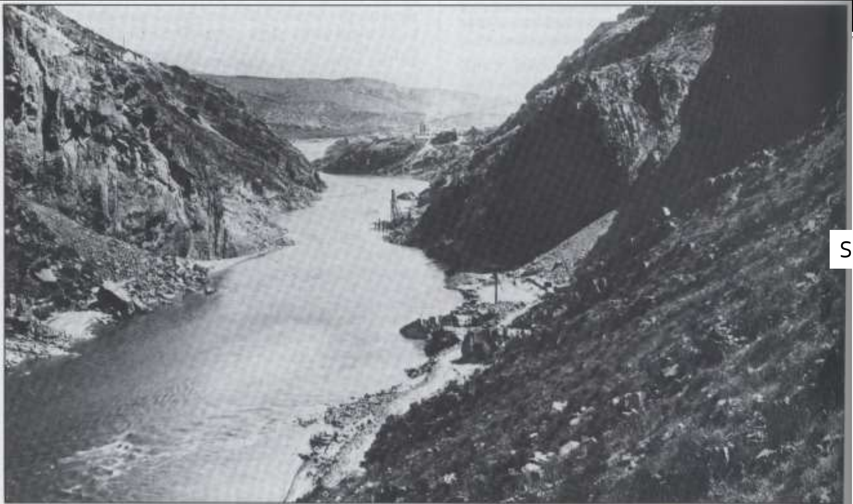
Looking upstream at site of Roosevelt Dam on the Salt River, April 16, 1906.
