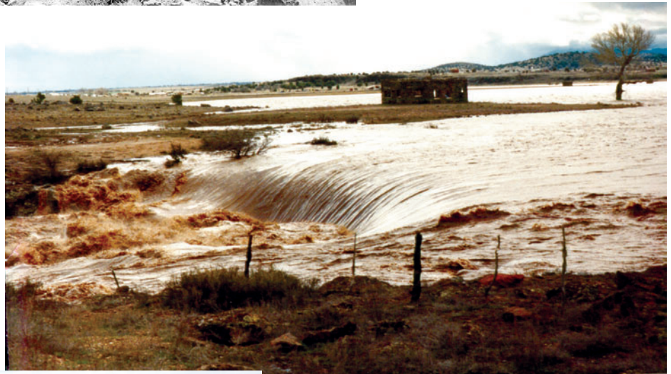
Figure 2.17 —Flood runoff from the February 1993 storms going over Sullivan Dam. The reddish, sediment-laden water is characteristic of the soils from the Big Chino Wash high in the watershed. (Photo by Alvin L. Medina.)
