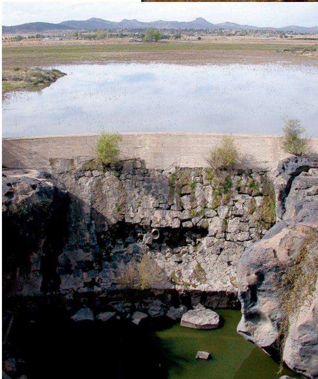
Figure 2.18 —This 2011 photo illustrates the current condition of the Sullivan Dam wall and minimal water storage in the remnants of Sullivan Lake. (Photo by Alvin L. Medina.)
