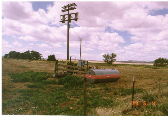
•Irrigation well on K4 farm (presently diesel fueled)
