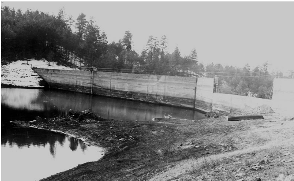
Title: Construction of Goldwater Dam, Prescott, Arizona, C.1934 Date of Photograph: 1934
