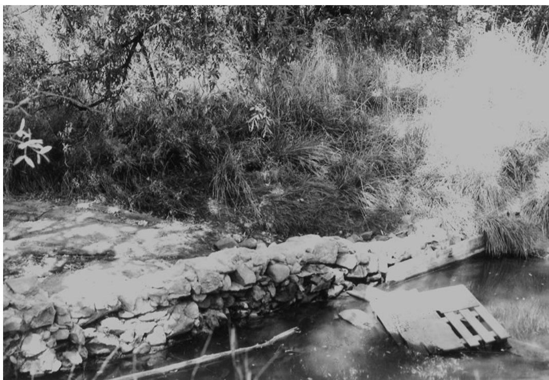
Title: Water plant and old city dam, Prescott, Arizona, September, 1928 Date of Photograph: 1928
