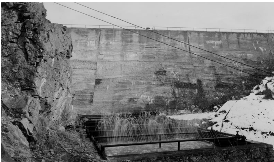
Title: Construction of Goldwater Dam, Prescott, Arizona, C.1934 Date of Photograph: 1934
