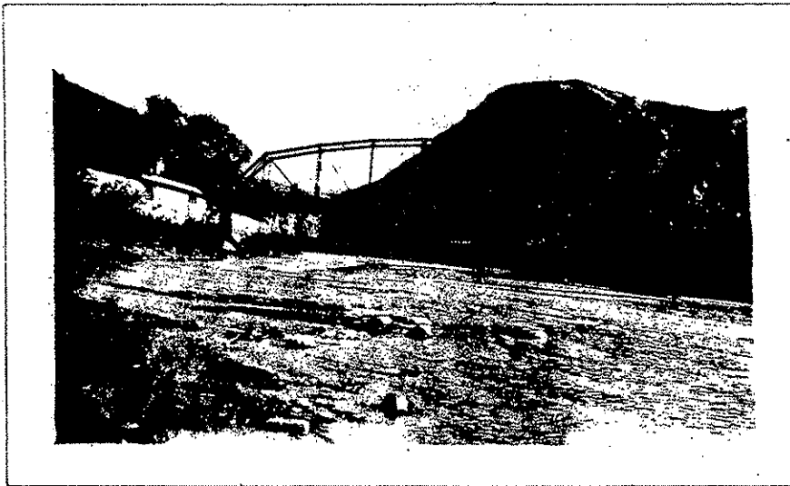
Looking downstream shows high water measuring section 1927 — 48 and after
