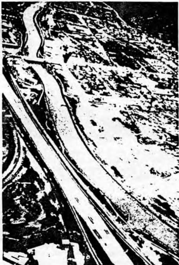
FIGURE 3 View looking downstream at the entrenched channel of the Santa Cruz River at Tucson, Arizona. Floodwater of the 100-year flood is confined within the channel of the reach. Lateral erosion of the channel banks is restricted by massive soil-cement banks. Interstate 10 is located to the left of the 200-foot-wide by 20-foot-deep river channel. Since 1914, the channel has widened about 100 feet and deepened about 15 feet.
