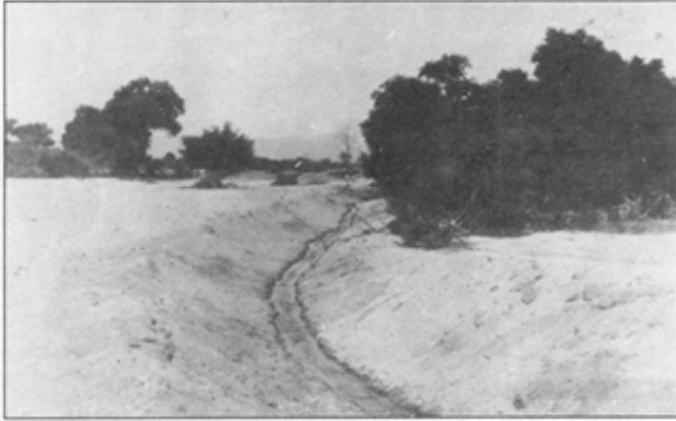
The Allison brothers' West Side Canal was built in the early 1890s to revive irrigated agriculture after the river became entrenched (photo 110. 4250 courtesy of the Arizona Historical Society).
