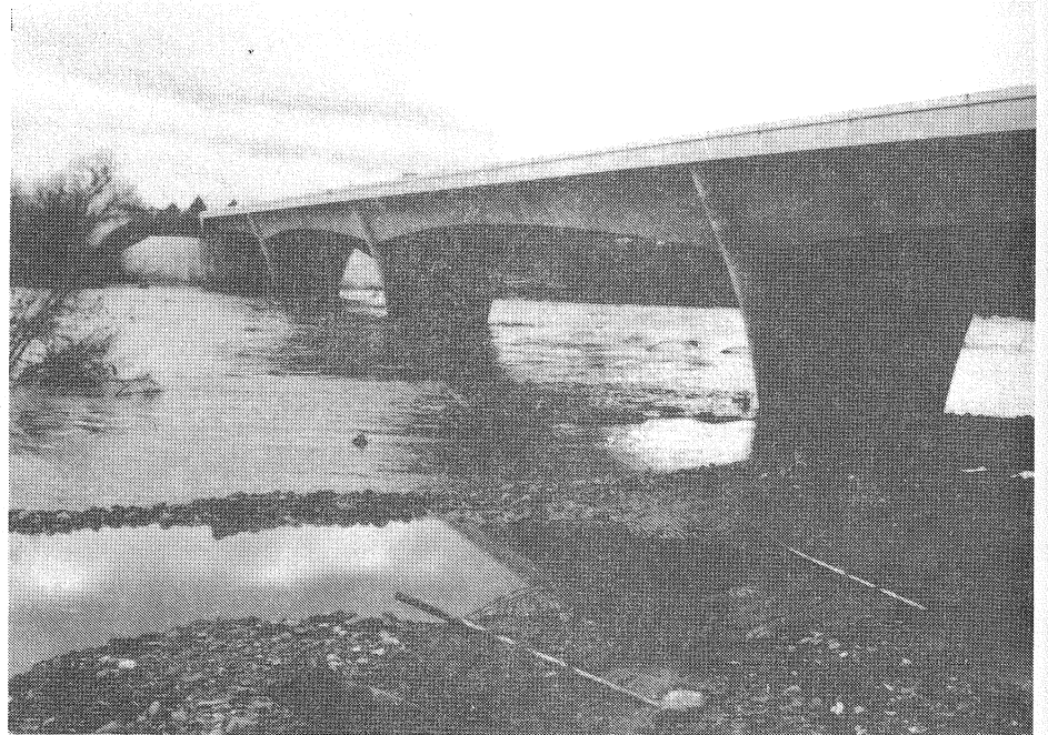
~Mile 79 - February, 1993 - Receding Floodwaters ~
