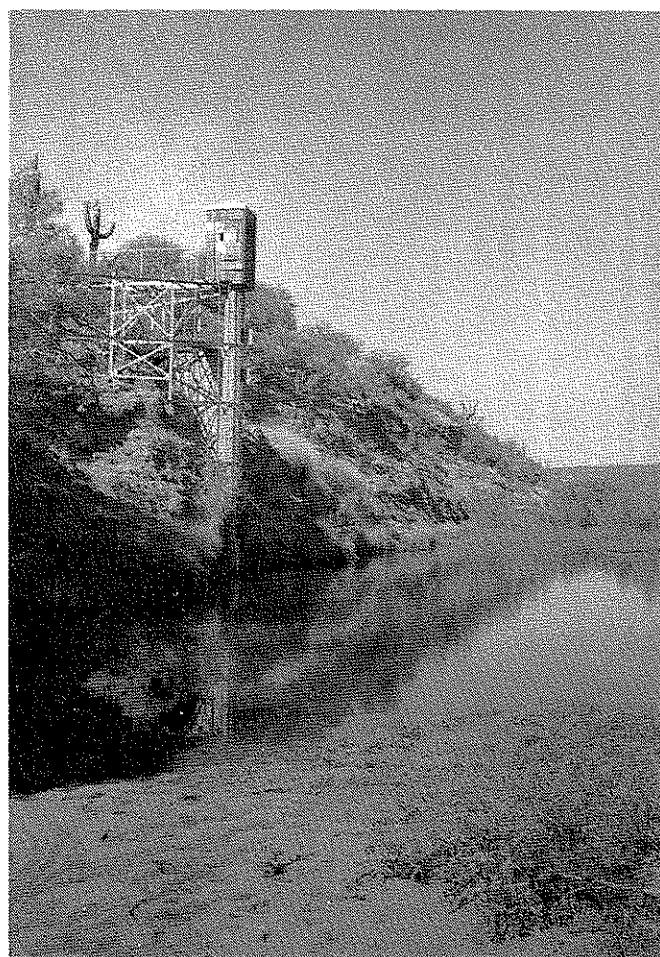
~ Gauging Station - Mile 153.9 ~
