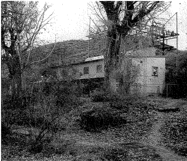
~ Childs Power Plant - Mile 106.5 ~
