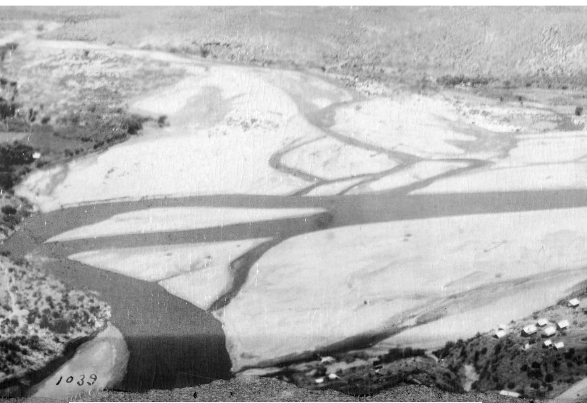
Salt River Roosevelt Dam Site – Preconstruction (Lubken), (Zoom)
