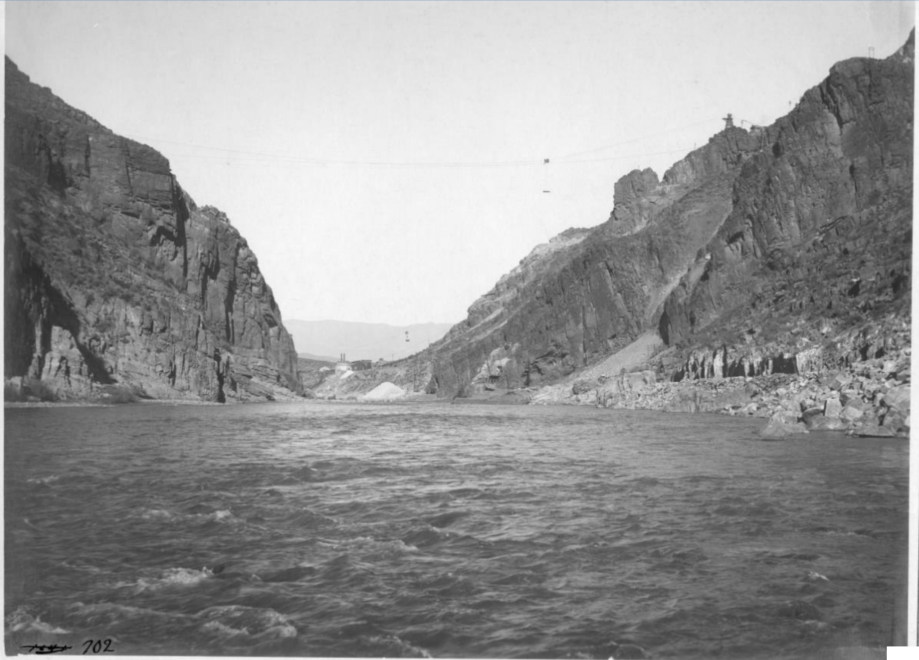
Salt River Dam Site Looking Upstream. Both Tramways in Action (Lubken), March 8, 1906
