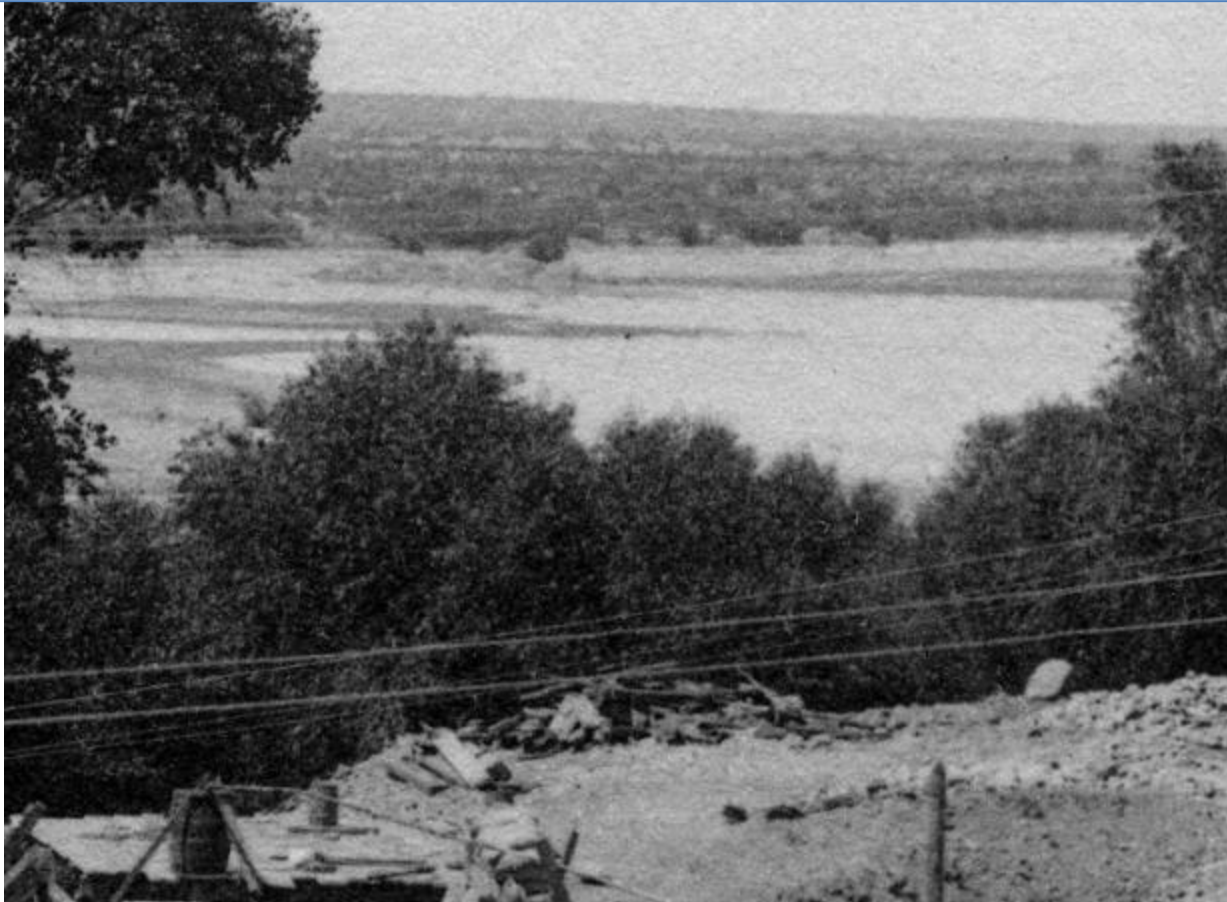
Coffer Dam, Arizona Canal, Granite Reef (Lubken), June 6, 1908, (Zoom 1)
