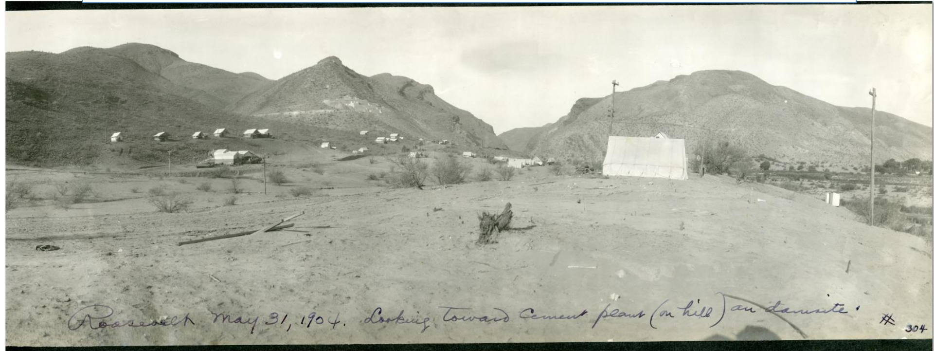
Roosevelt, Looking Toward Cement Plant and Damsite (Lubken), May 31, 1904
