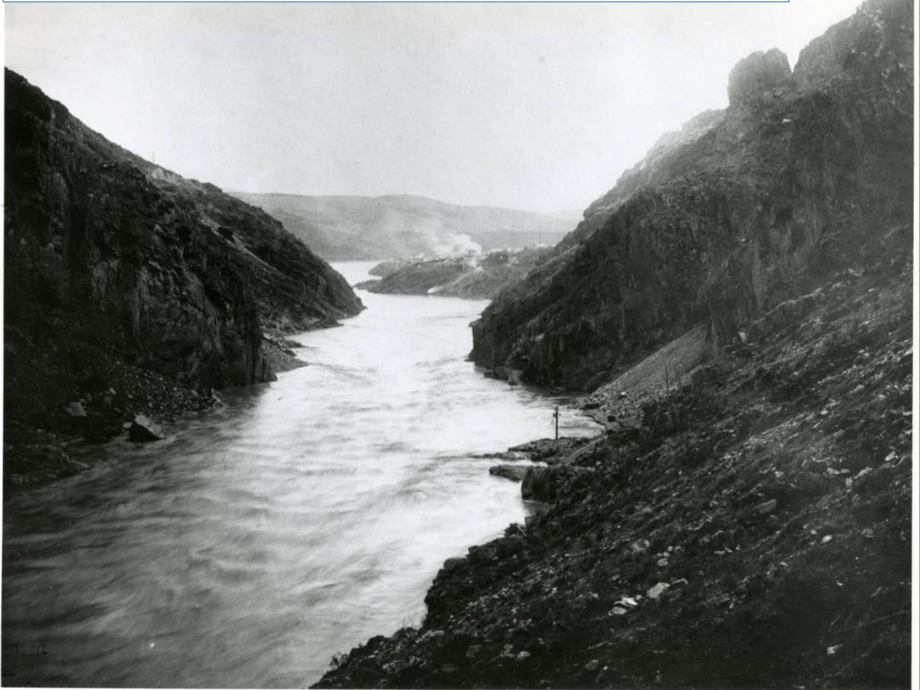
Salt River Dam Site Looking Downstream from Pt 3 (WJL), March 12, 1906
