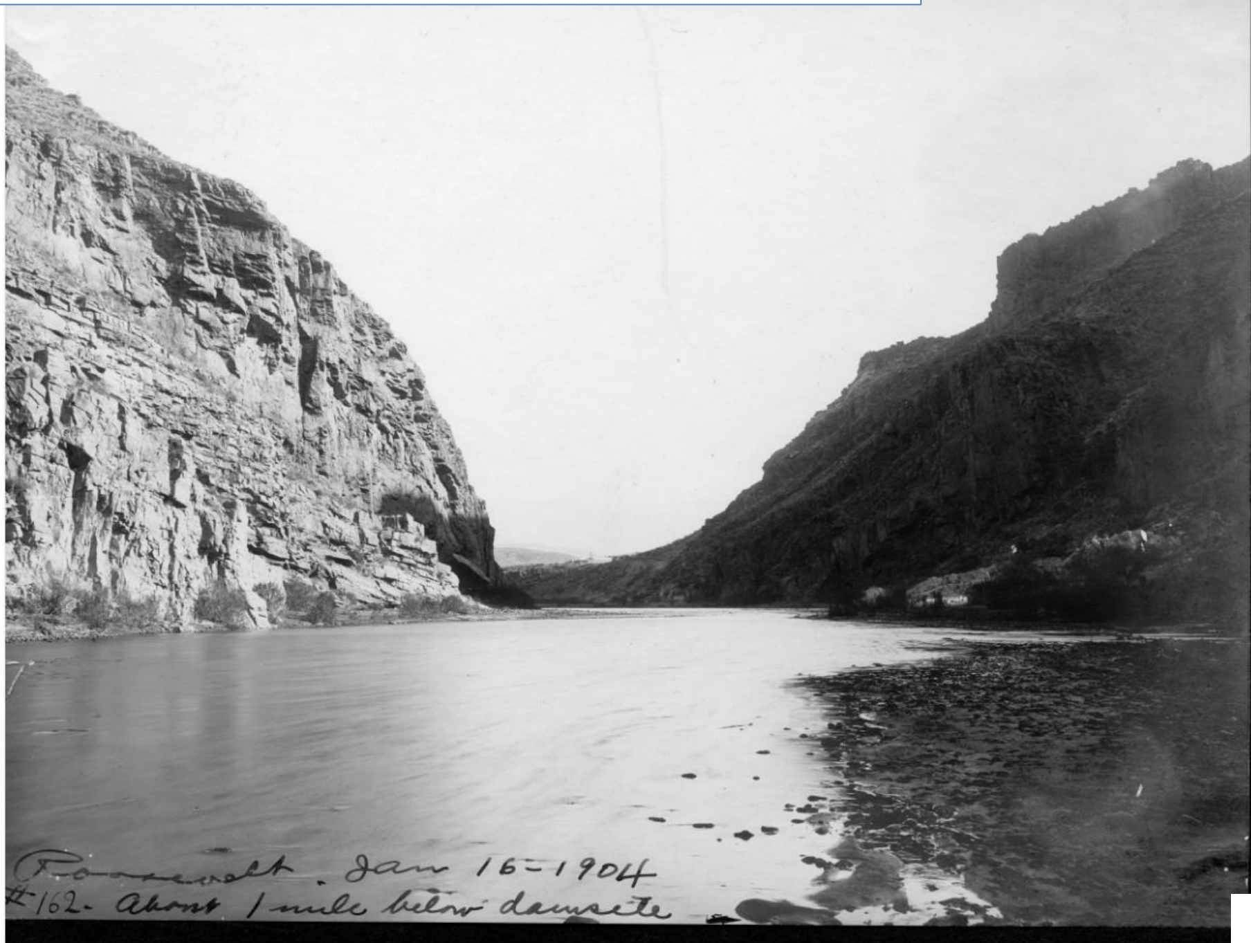
Roosevelt, About 1 Mile Below Damsite (Lubken), January 16, 1904
