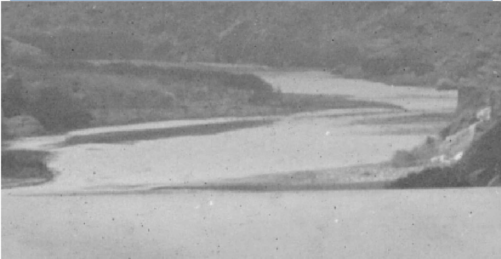
Roosevelt, Looking Down Canyon Toward Cement Plant & Damsite (Lubken), January 16, 1904 (Zoom)
