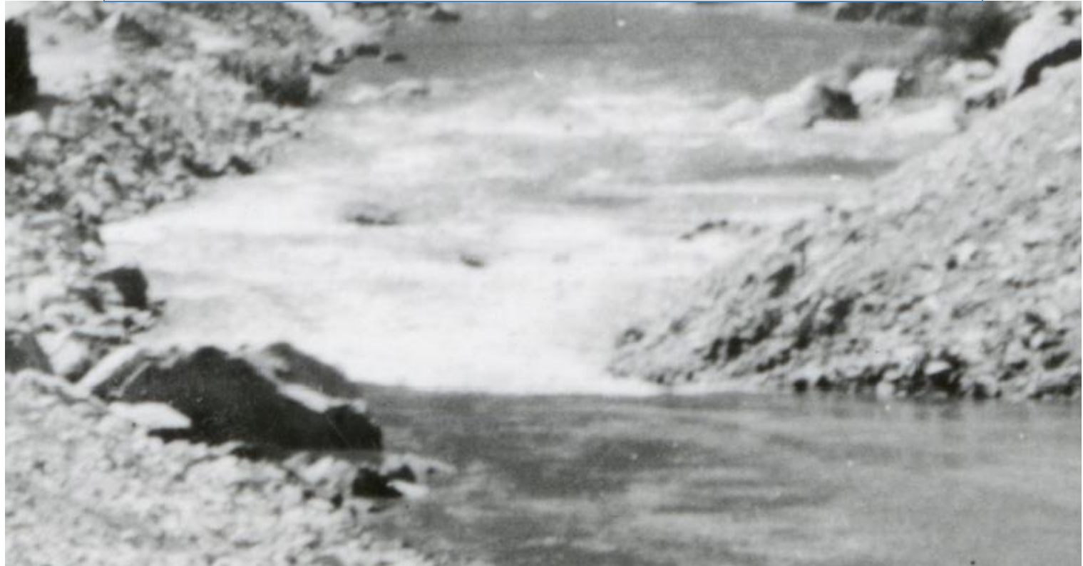
Horse Mesa Dam Excavation – September 24, 1925 (Zoom)
