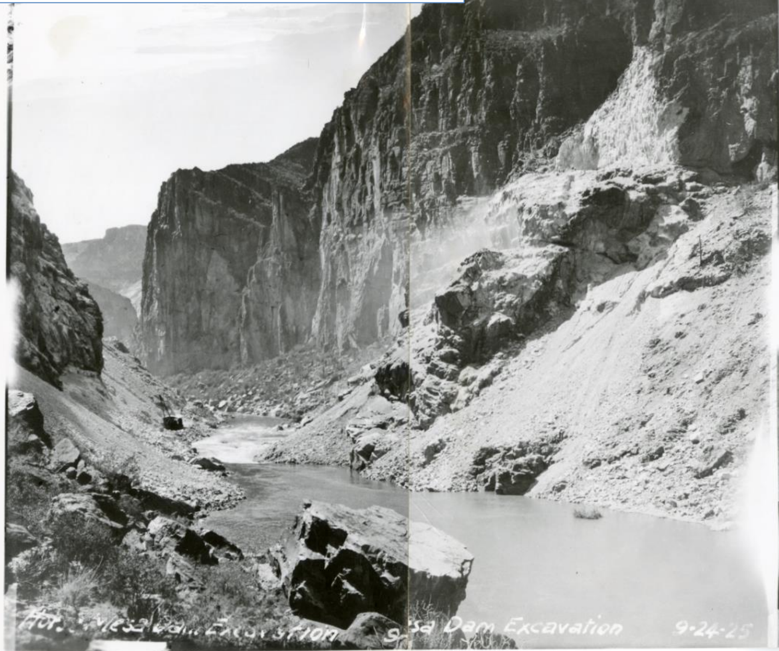
Horse Mesa Dam Excavation – September 24, 1925
