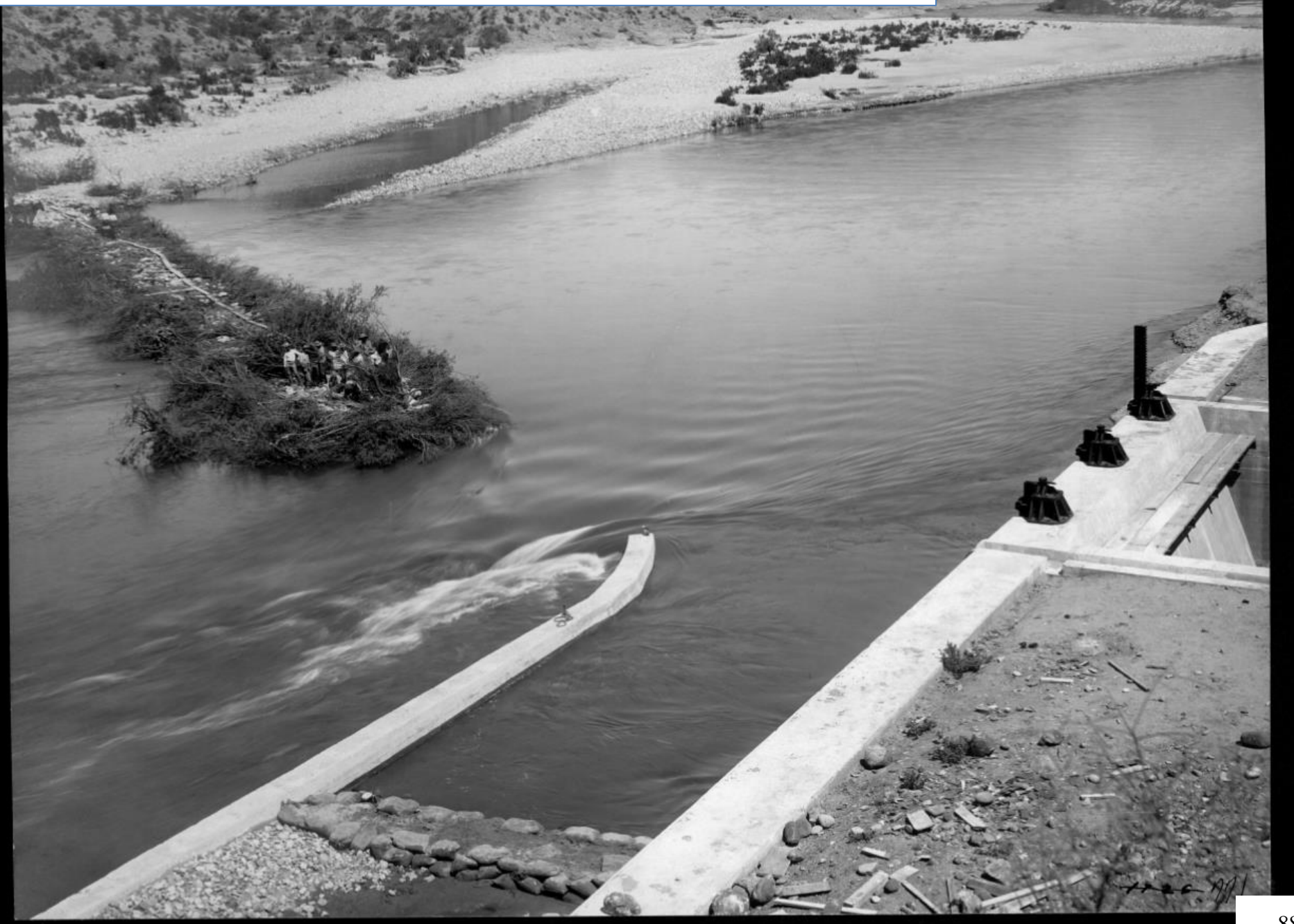
Temporary Bush Dam Intake of Power Canal (Lubken), May 1, 1906
