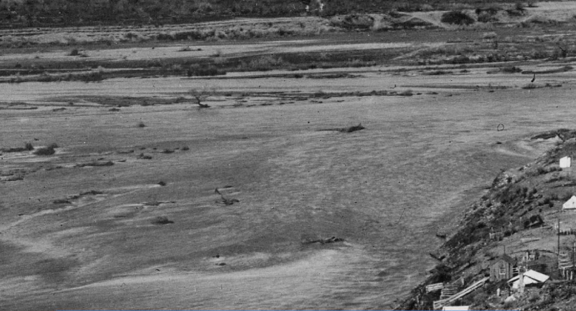
Cement Plant and Electric Powerhouse (Lubken), February 21, 1905 (Zoom 2)
