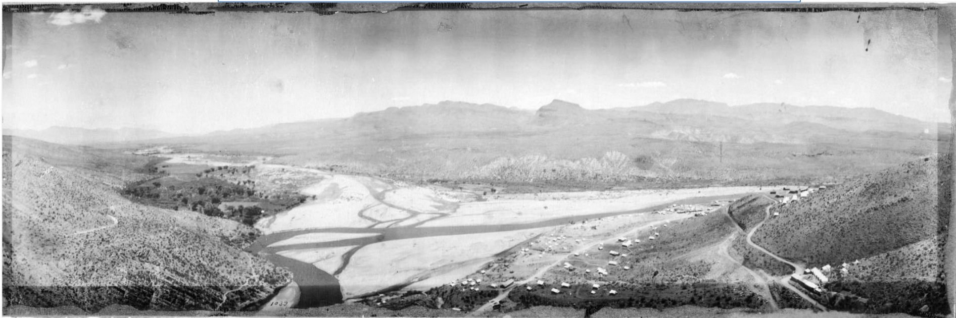
Salt River Roosevelt Dam Site – Preconstruction (Lubken)
