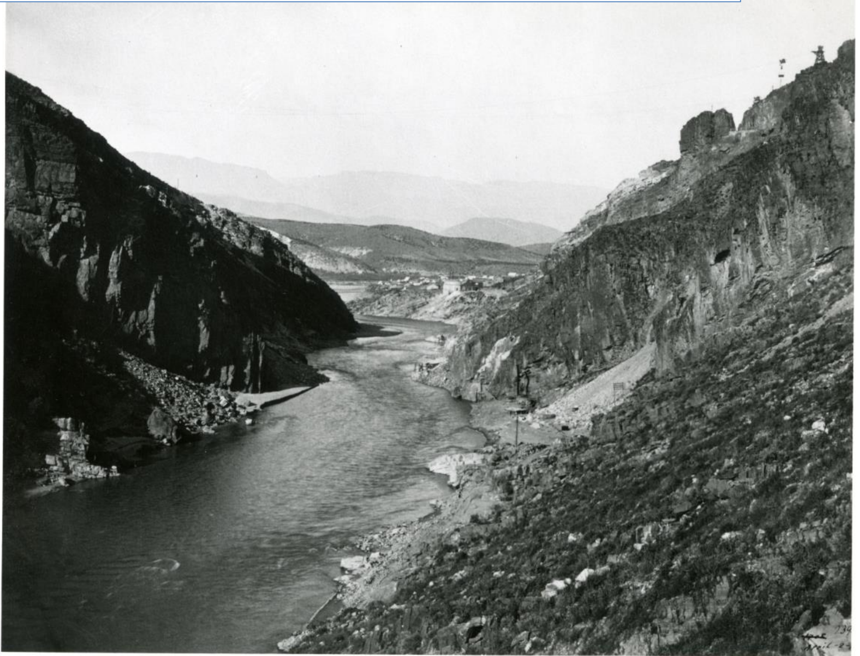
Salt River Dam Site Looking Upstream from Pt 3 (WJL), March 12, 1906
