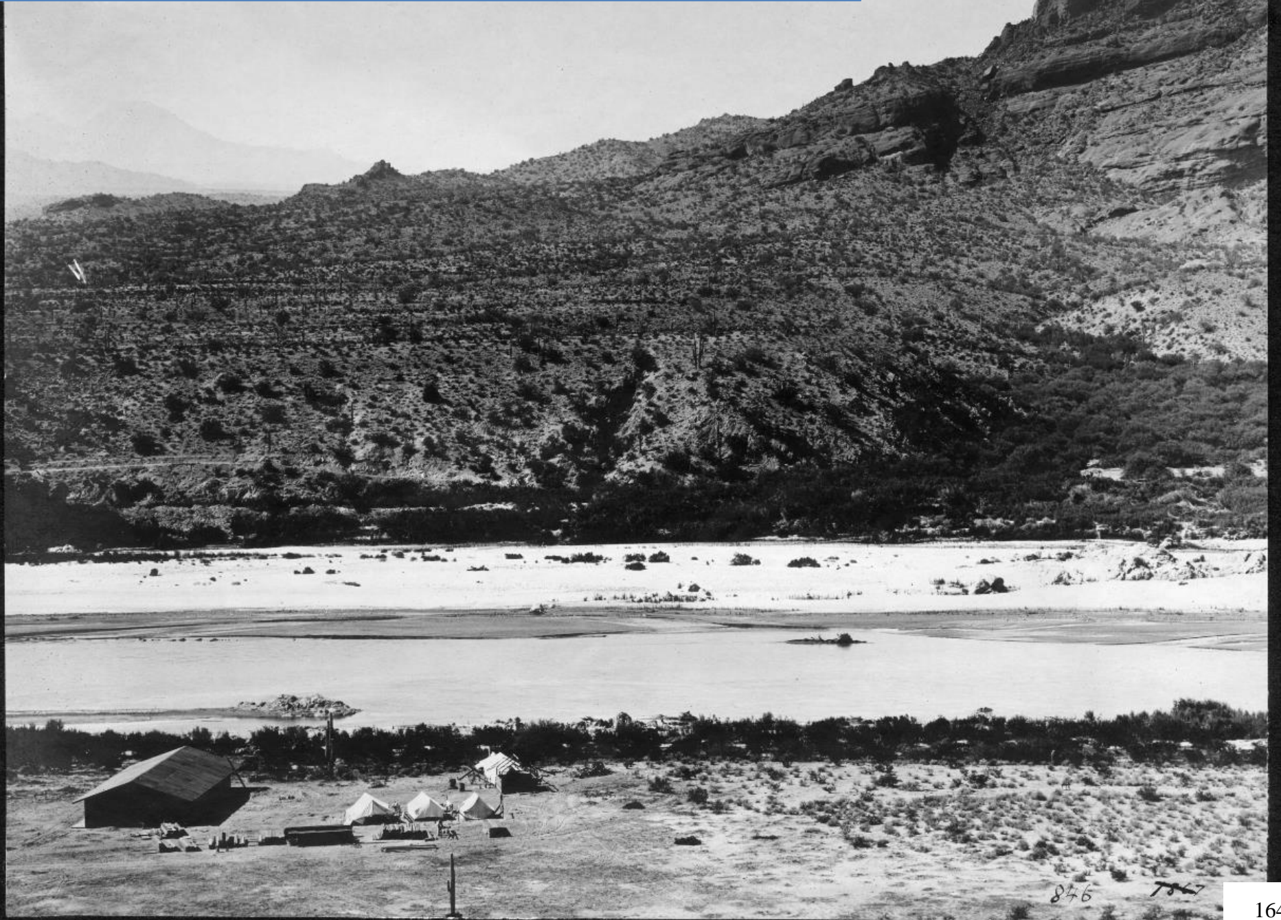
Dam Site & Camp at Granite Reef (Lubken), September 5, 1906
