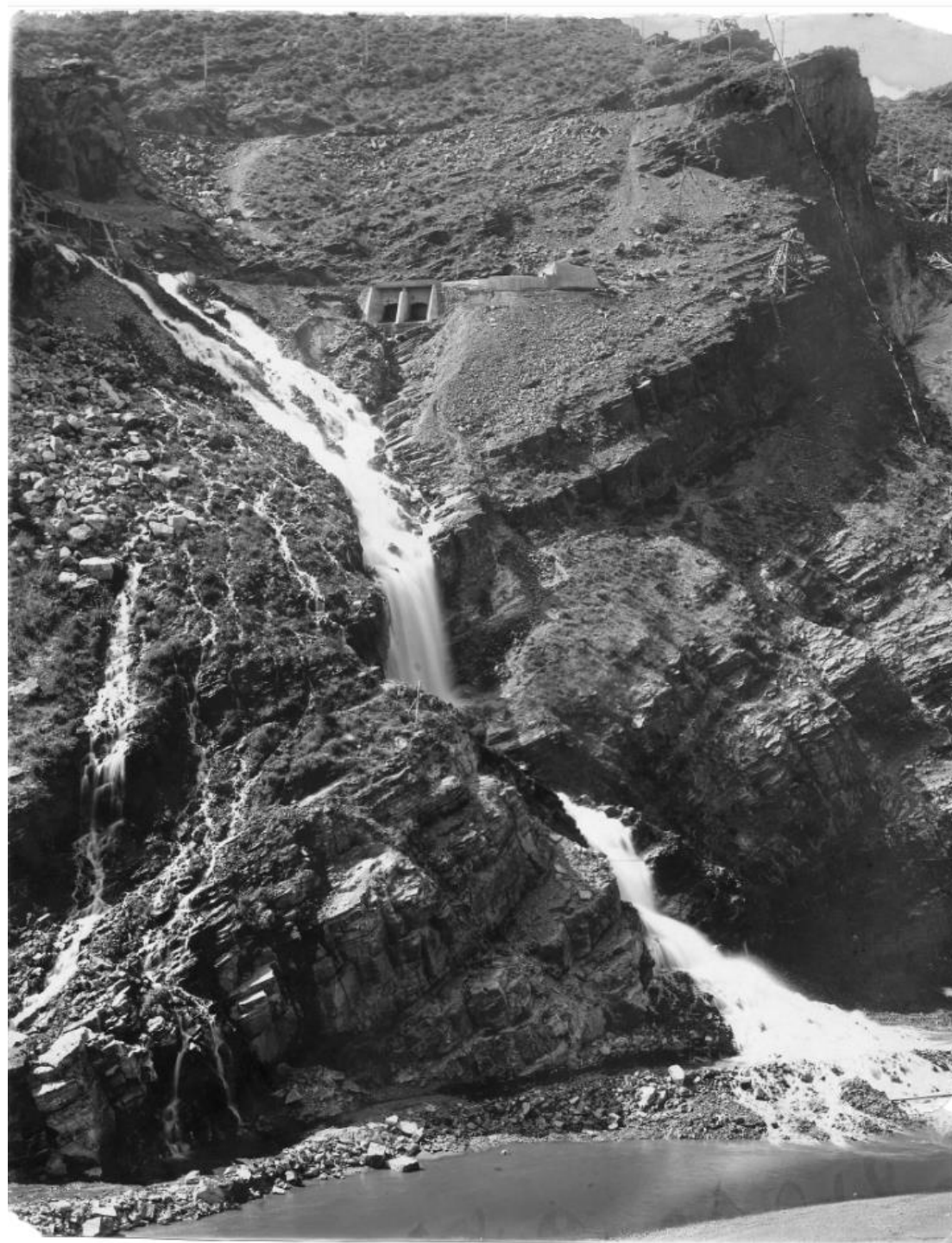
Overflow Weir at Head of Penstock Tunnel on Salt River Power Canal (Lubken), April 21, 1906
