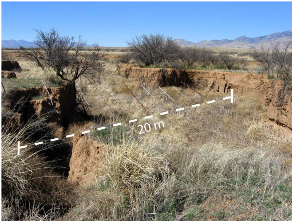
Figure 18. Recent headward erosion and arroyo cutting has undermined a fence across upper Aravaipa Creek.
