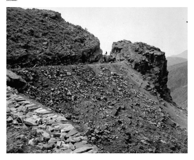
Figure 28: Construction of high-line wagon road directly above Roosevelt Dam site, March 29, 1905. Source: Records of the Bureau of Reclamation, U.S. National Archives Branch, Rocky Mountain Region, Denver, Colorado.
