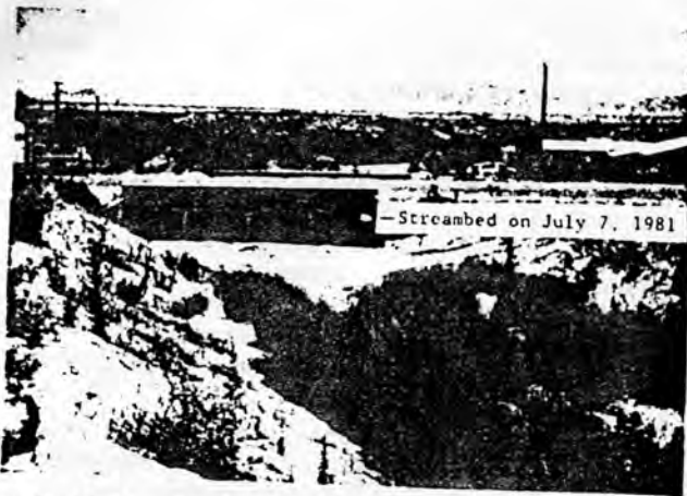
FIGURE 13 View looking downstream at culvert on U.S. Highway 80 in south Benson, Arizona. The opening was nearly filled during the flash flood of July 6, 1981. Floodflow velocities in the main channel downstream from the culvert were very high and a local resident observed two standing waves about 20 feet apart at the flood peak. See figure 11 for location of photograph.
