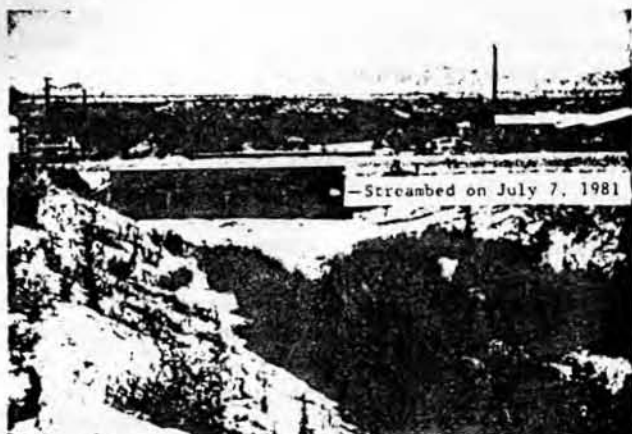
FIGURE 13 View looking downstream at culvert on U.S. Highway 80 in south Benson, Arizona. The opening was nearly filled during the flash flood of July 6, 1981. Floodflow velocities in the main channel downstream from the culvert were very high and a local resident observed two standing waves about 20 feet apart at the flood peak. See figure 11 for location of photograph.
