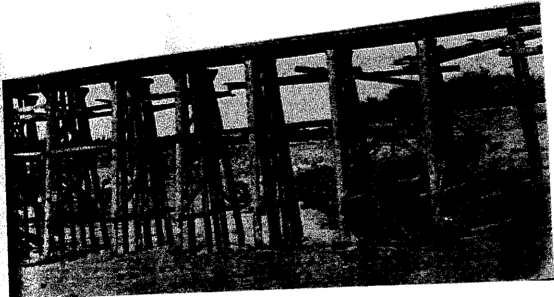
Below: A temporary railroad trestle spans the river.
